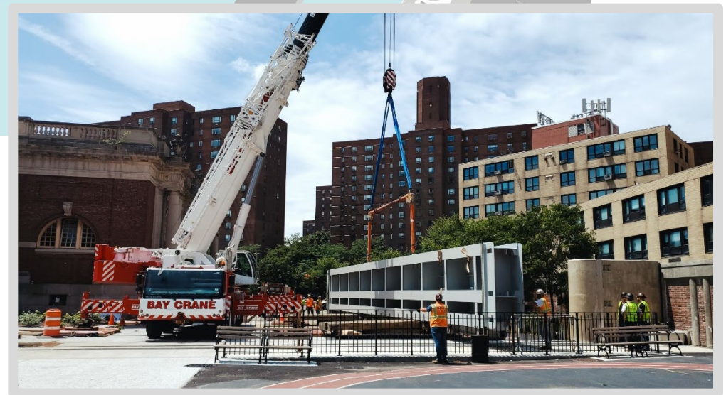
Floodgate 18 installed at Asser Levy Playground
