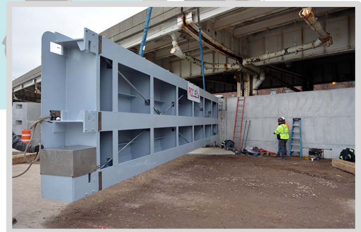
Operation 1: First floodgate installed at Stuyvesant Cove Park February 24, 2022.
