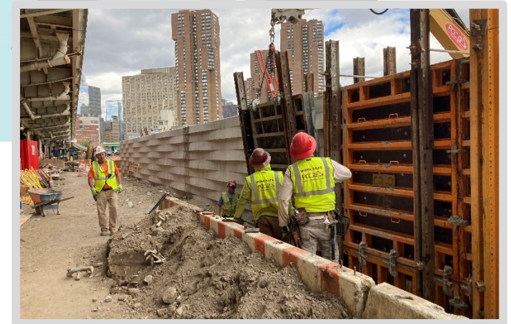
Operation 1: Ongoing floodwall construction in Stuyvesant Cove Park.
