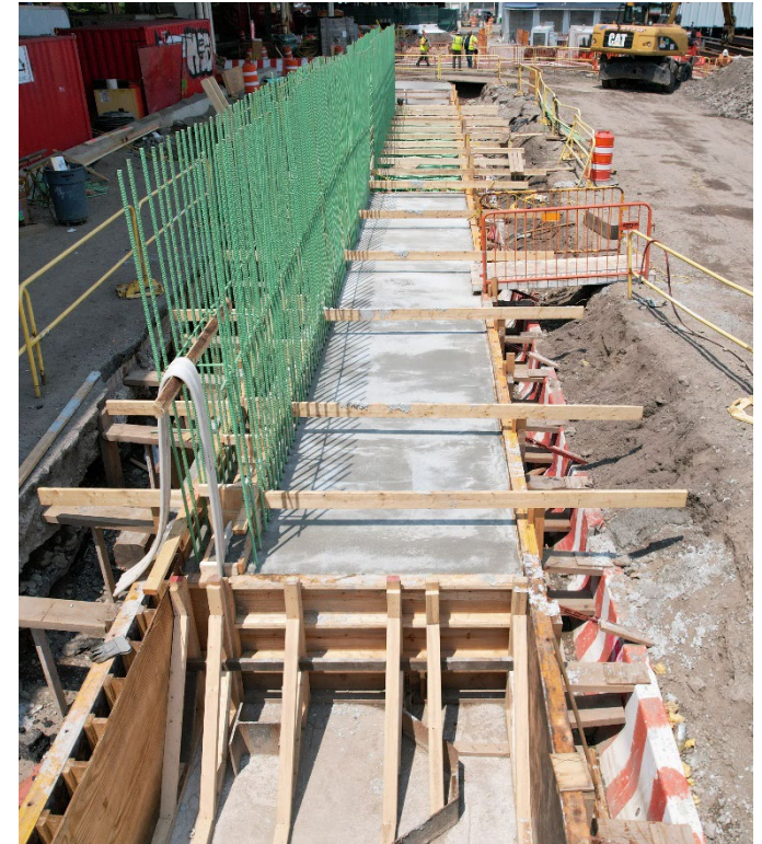
Operation 1: Flood wall foundation work progresses.
