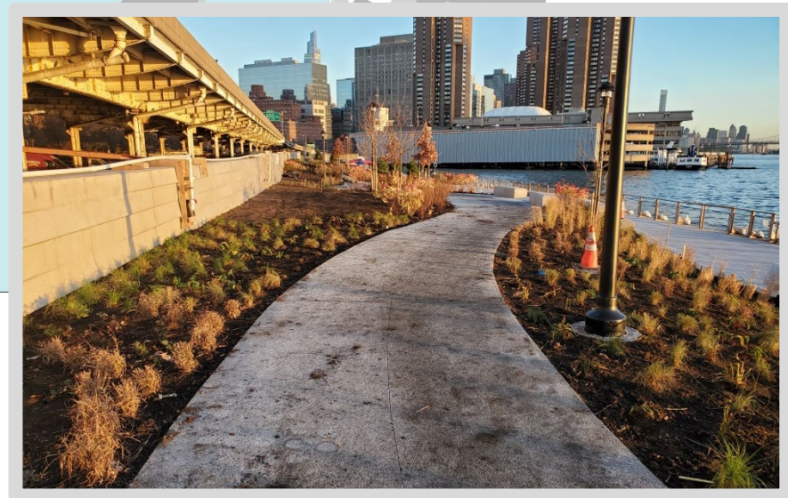
Stuyvesant Cove Park (Northern part) site restoration in progress, November 2022
