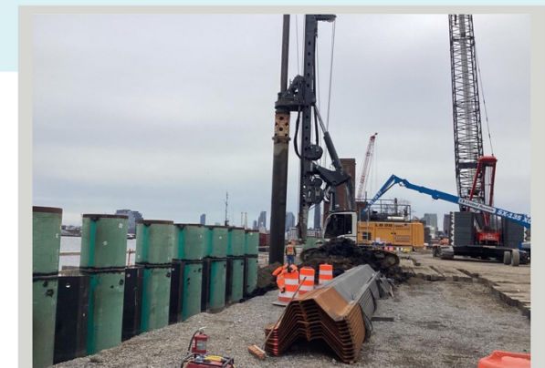
Combi-wall installation in East River Park, April 2023
