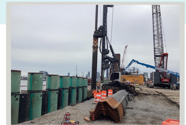
Combi-wall installation in East River Park, April 2023
