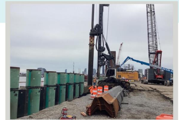
Combi-wall installation in East River Park, April 2023
