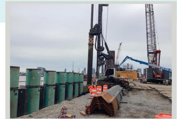
Combi-wall installation in East River Park, April 2023
