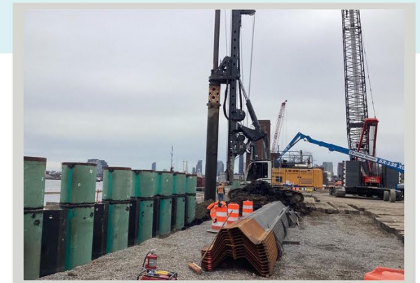
Combi-wall installation in East River Park, April 2023
