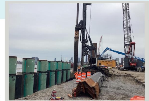
Combi-wall installation in East River Park, April 2023
