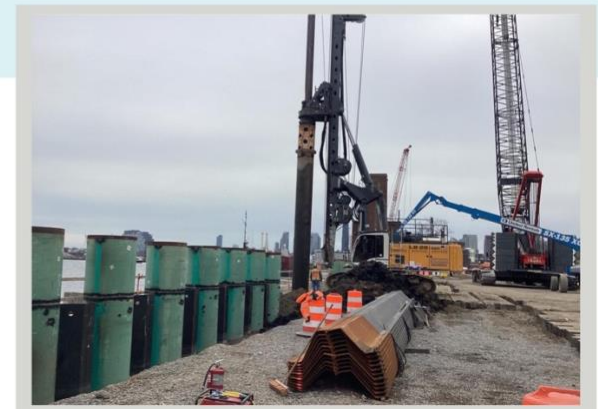
Combi-wall installation in East River Park, April 2023
