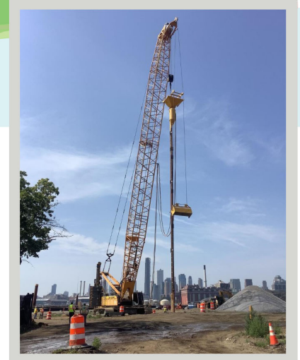
Soil Stabilization at East River Park waterfront, July 2022
