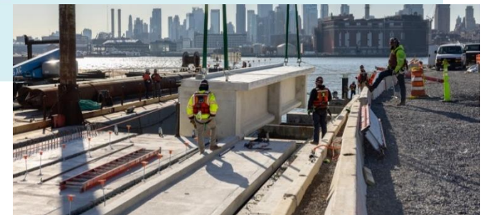
Pre-cast esplanade construction & installation - December 2023
