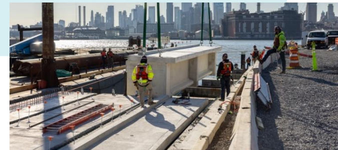
Pre-cast esplanade construction & installation - December 2023
