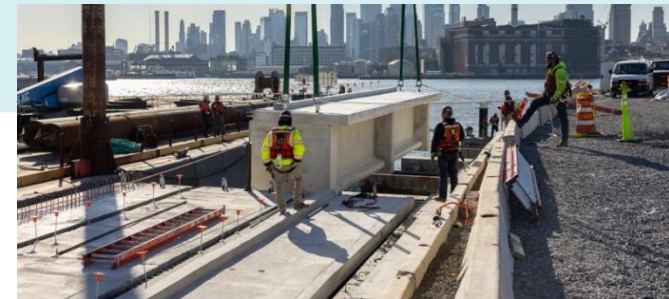
Pre-cast esplanade construction & installation - December 2023
