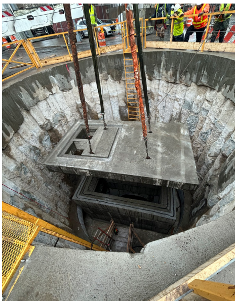
Deep drop manhole roof slab installation at Delancey St. S and Baruch Dr., February 2026
