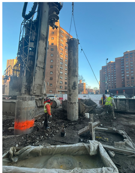
Secant pile installation for deep drop manhole at
