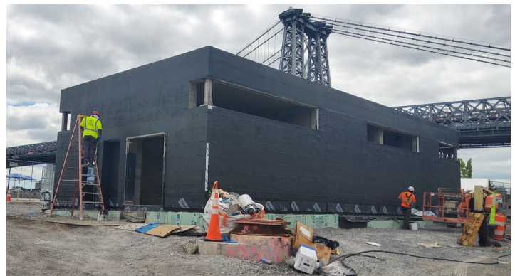
Installation of waterproofing at new Tennis building, June 2026
