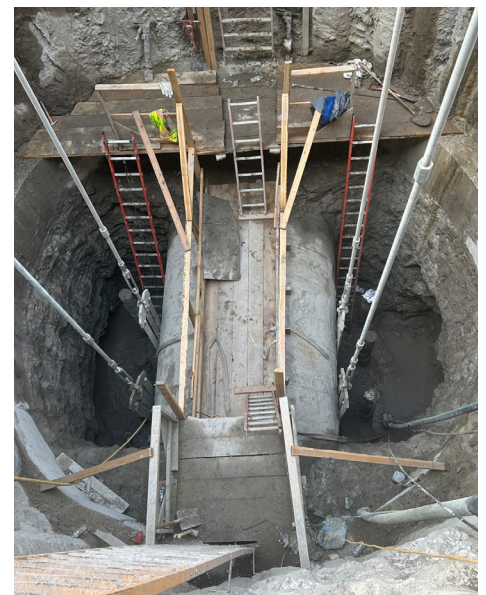
Supporting existing sewer in Delancey St. N deep drop manhole, April 2026
