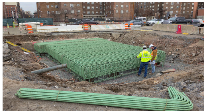
Rebar for E. 10th St. Bridge eastern abutment, March 2026
