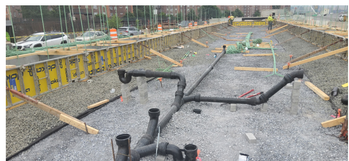
Plumbing work for new Track House, June 2026
