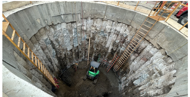
Excavation for deep drop manhole in Delancey St. North, March 2026
