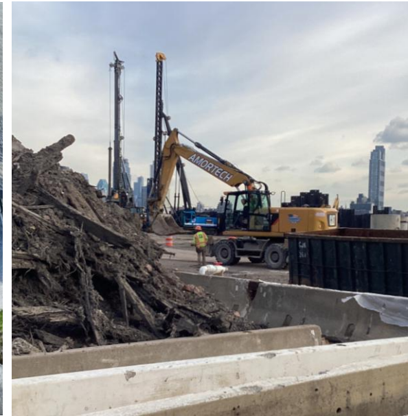
Debris excavated in Track area – Dec 2025
