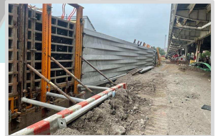
Operation 2: Ongoing floodwall construction in Stuyvesant Cove Park.
