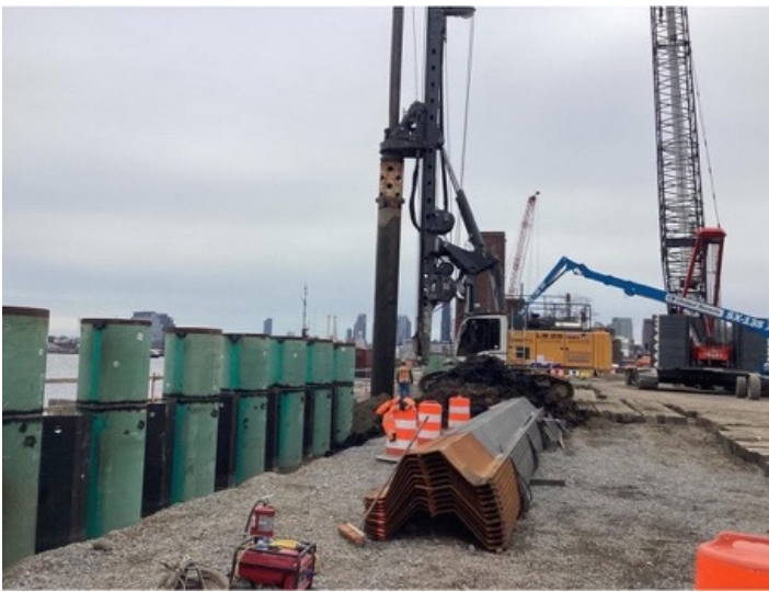
Combi-Wall construction, April 2023
