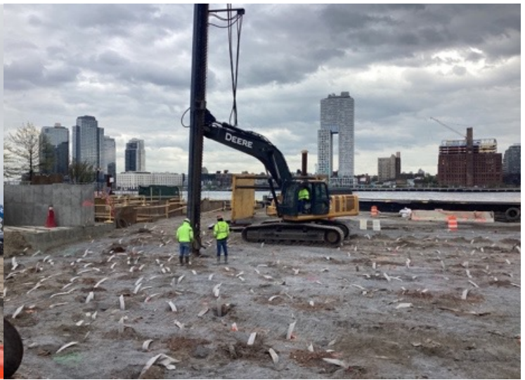
Wick drain installation, April 2023
