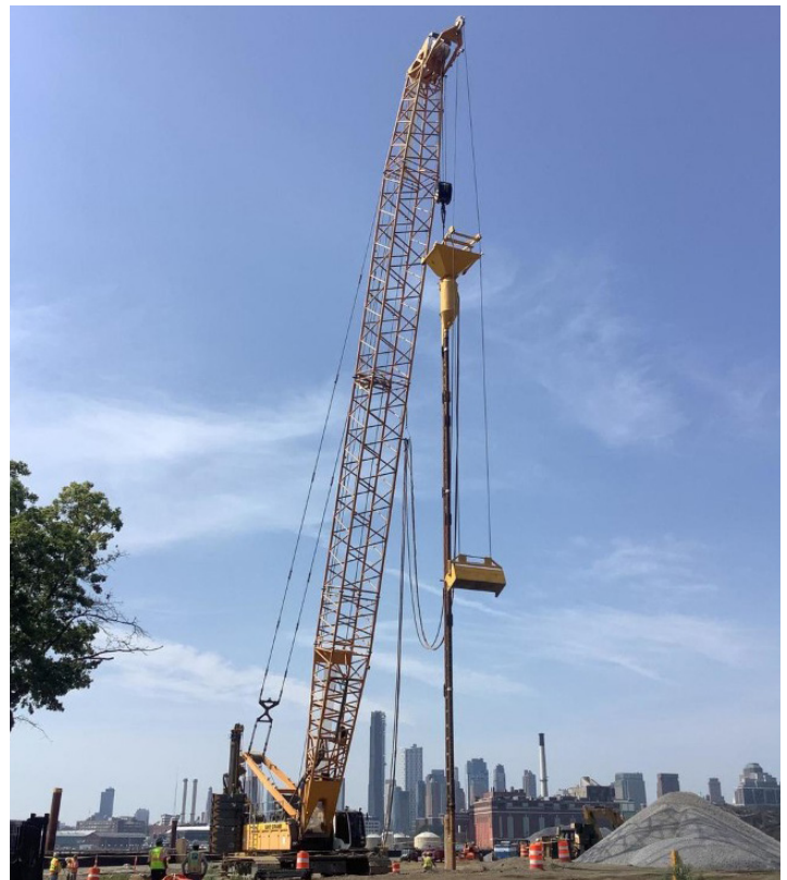
Soil Stabilization at East River Park Waterfront, July 2022
