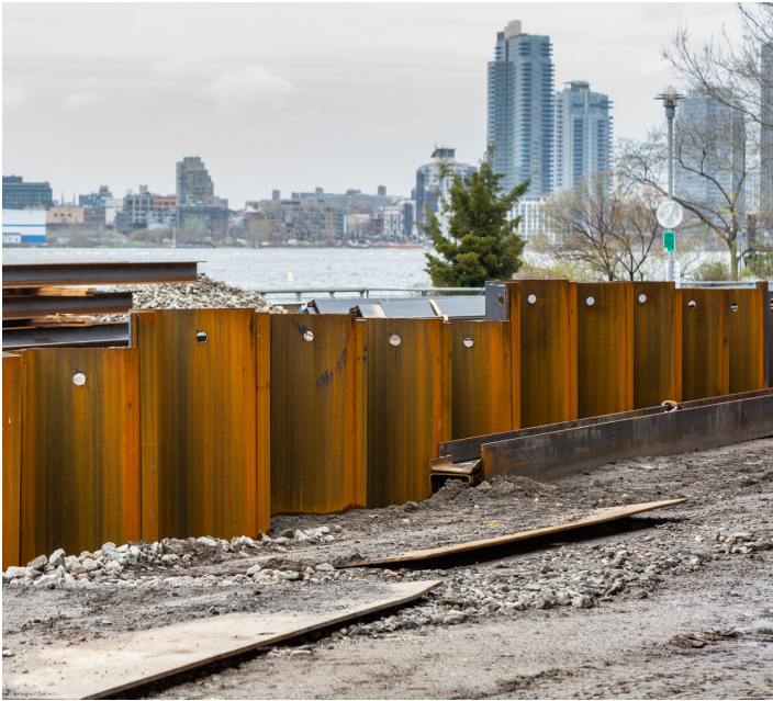
Sheet piles installed at Stuyvesant Cove Park
