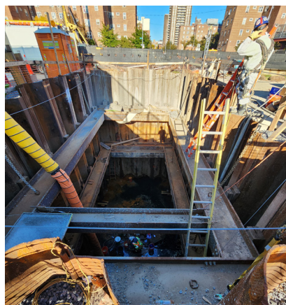
Launching pit construction, October 2024
