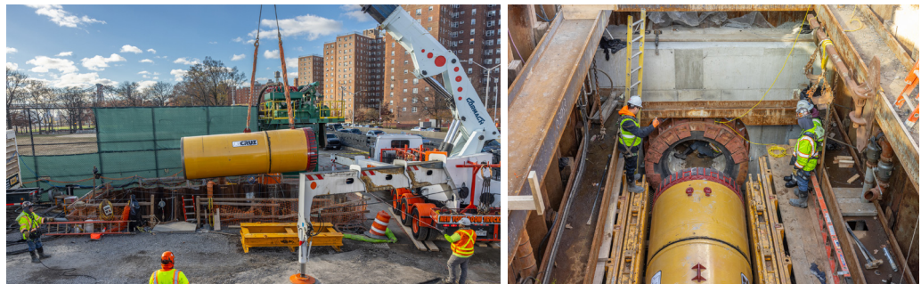
Microtunneling machine being lowered into launching pit in East River Park, December 2024
