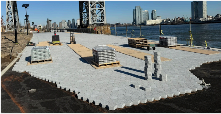
Pavers installed on esplanade south of Williamsburg Bridge, December 2024
