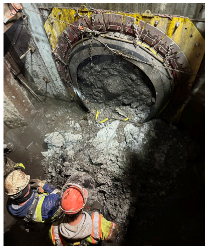
Microtunneling machine breaking through receiving pit in E. 10th St., December 2024
