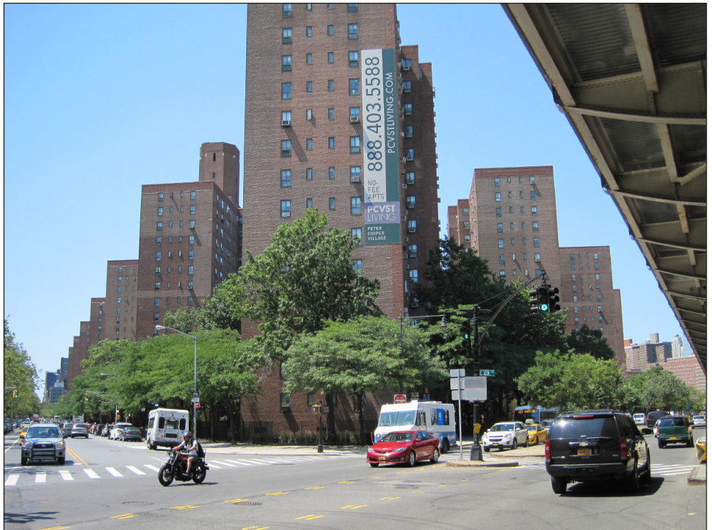
Peter Cooper Village (#17). View northwest at FDR Drive and East 20th Street 23
