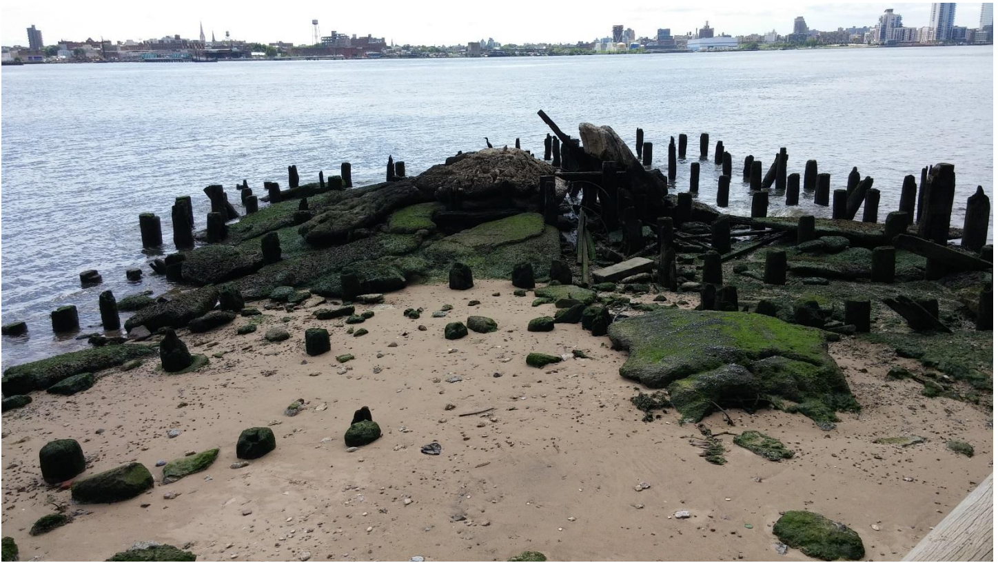
Photo 16 – Intertidal sand flat associated with remains of derelict dock/pier. Photo taken facing southeast.
