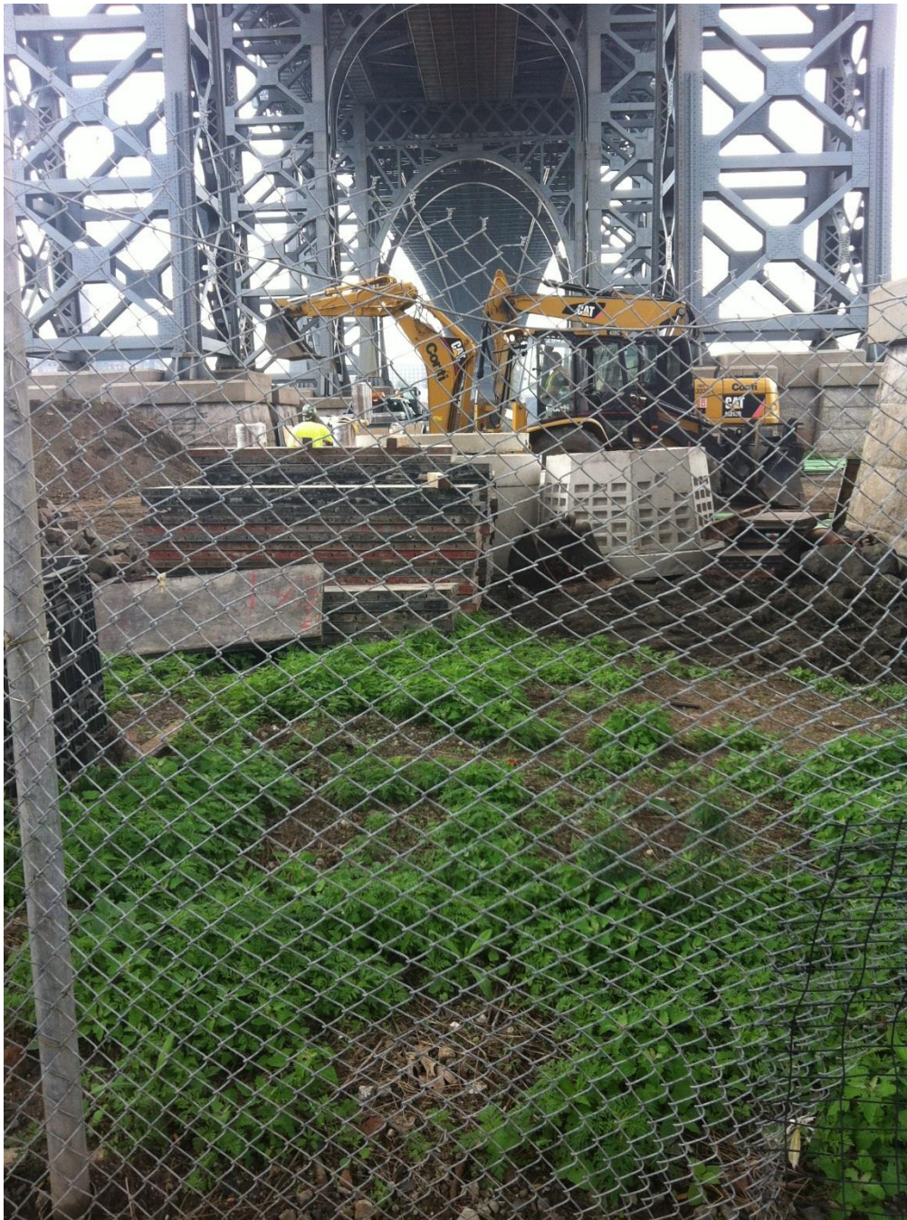
Photo 1 – Active construction underneath the Williamsburg Bridge. Photo taken facing southeast.
