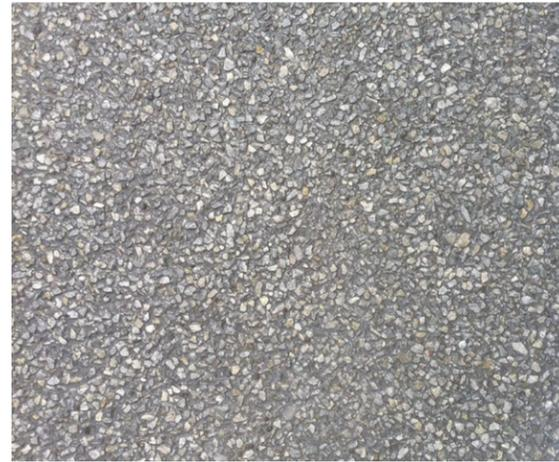
**EXPOSED AGG. CONCRETE PAVEMENT W/ SAW CUT JOINTS**
