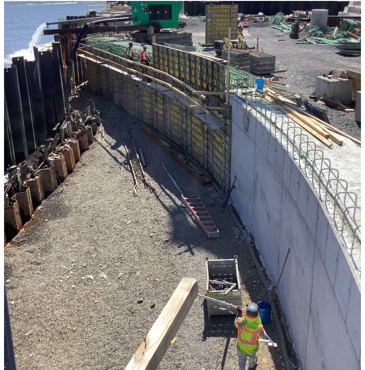
Concrete formwork for new embayment at E. Houston Street – September 2026
