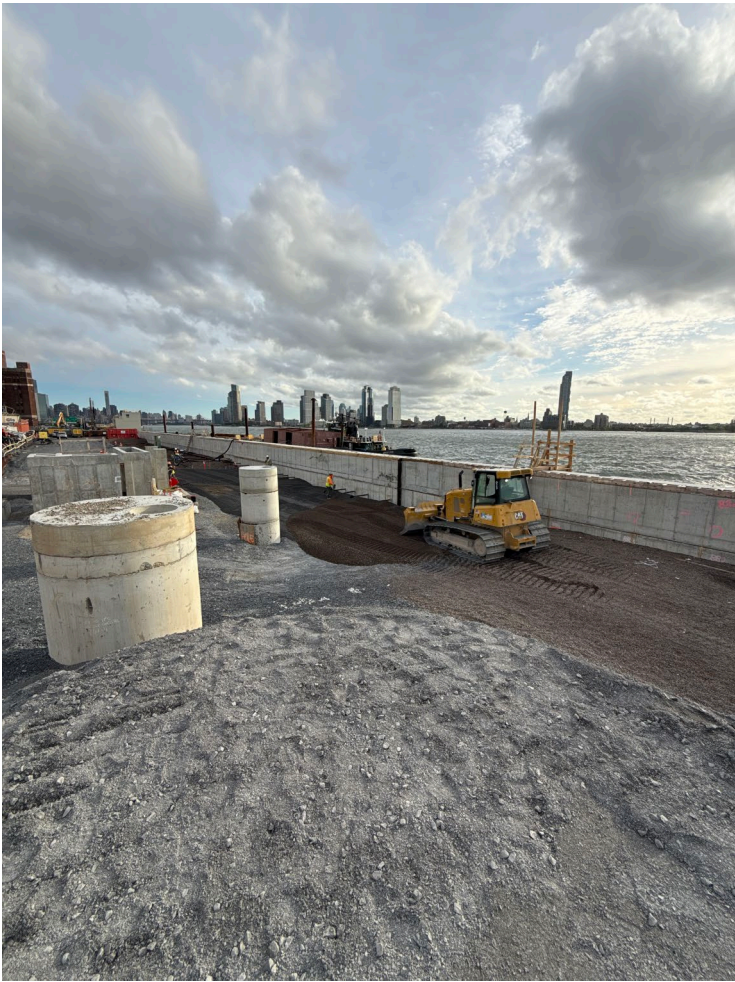
Compaction of lightweight fill along esplanade near Field 7 – September 2026
