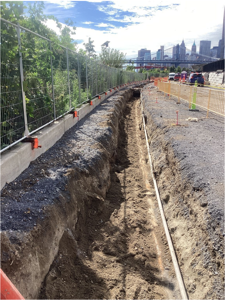
Trench for water main adjacent to Pier 42 – September 2026
