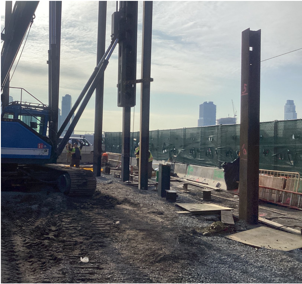
Installation of piles for E. 10 th Street bridge ramps – September 2026
