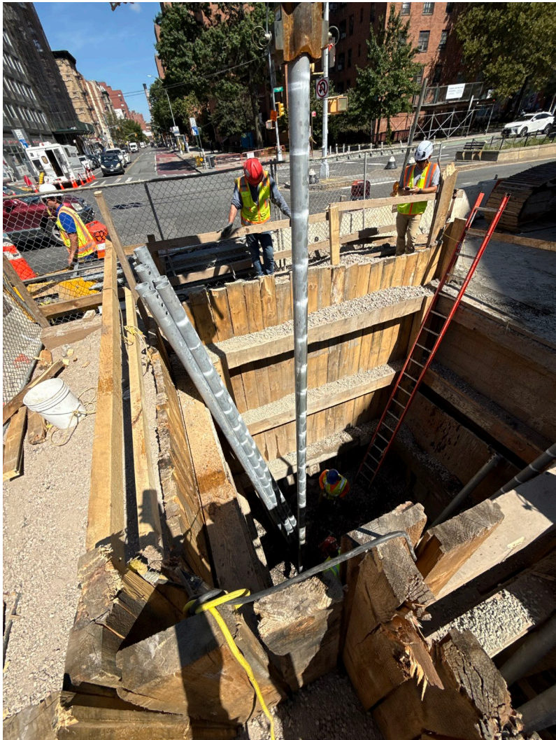
Helical pile installation in Columbia Street – September 2026
