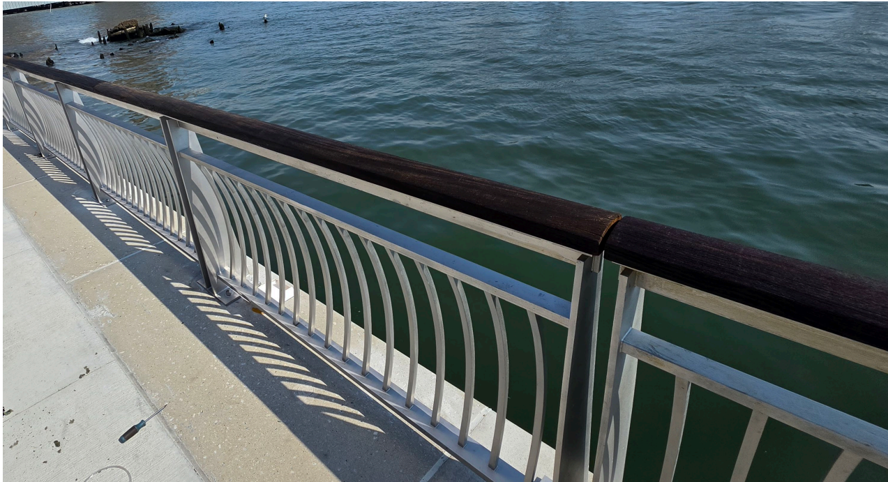
Replacement of sea rails in Stuyvesant Cove Park (punch list) – September 2026
