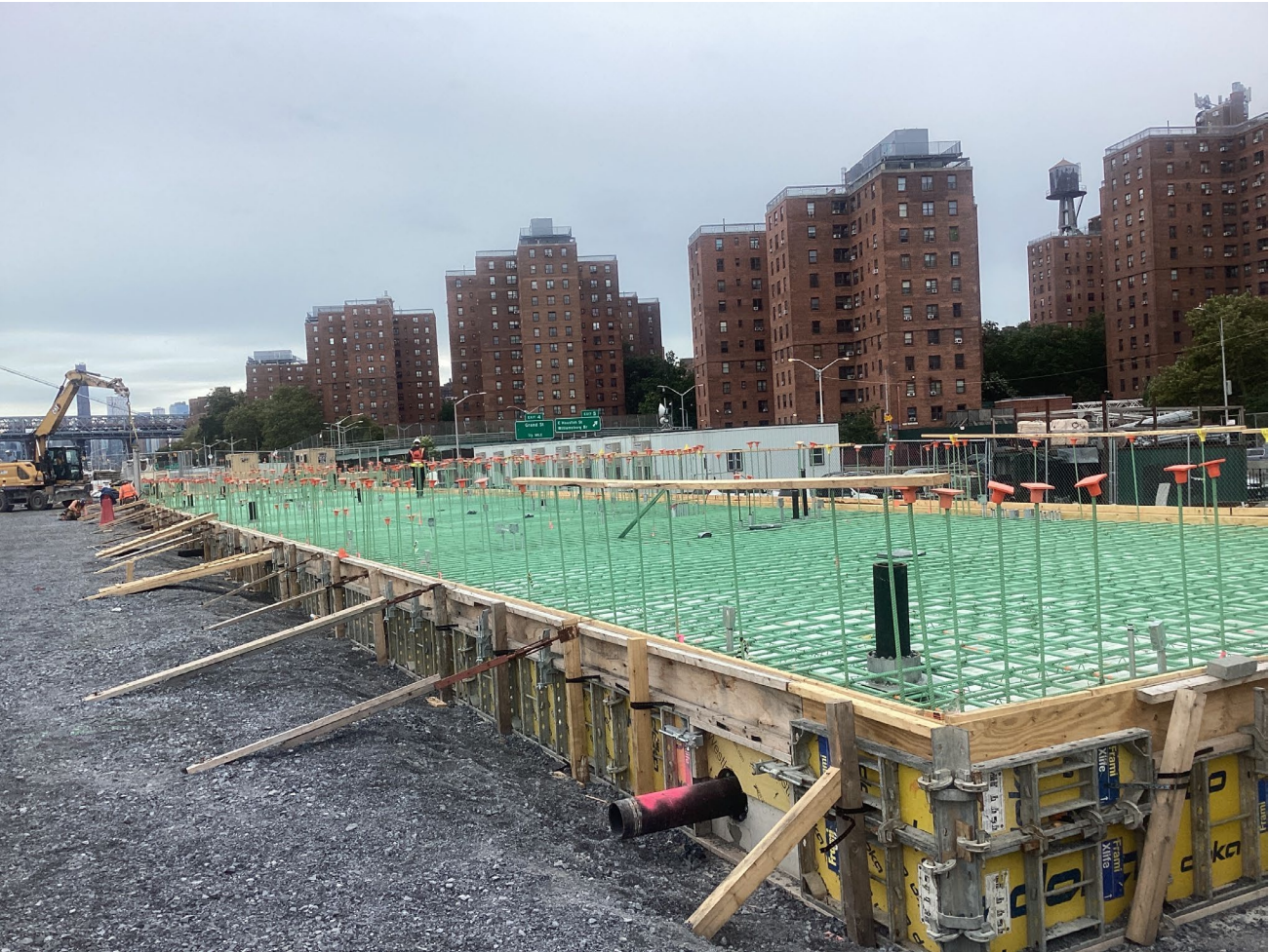
Installation of rebar for track house foundation slab – September 2026
