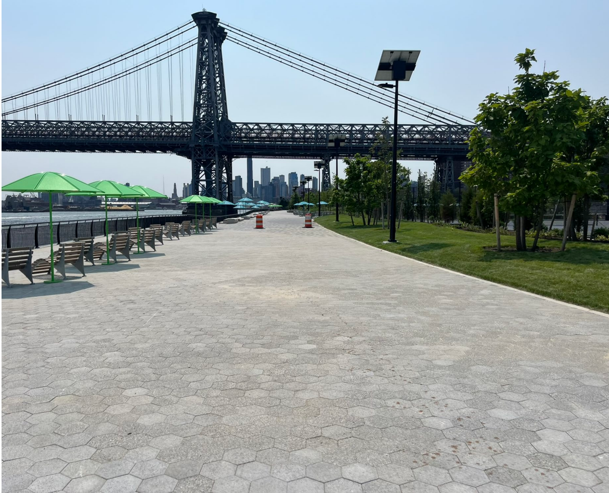
New portion of esplanade opened adjacent to north tennis courts – August 2026
