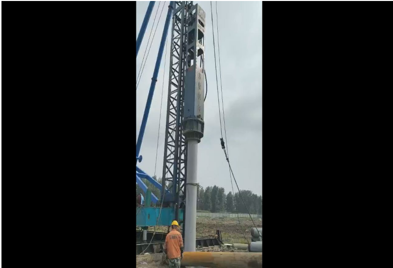
Example of impact hammer pipe pile installation, via https://www.youtube.com/shorts/avgWzm1MXpA
