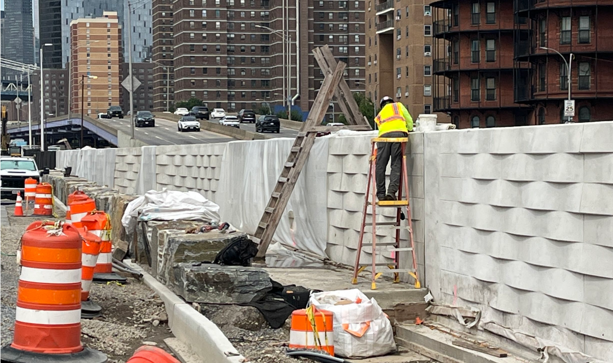
Floodwall construction and curb work south of Corlears Hook – August 2026
