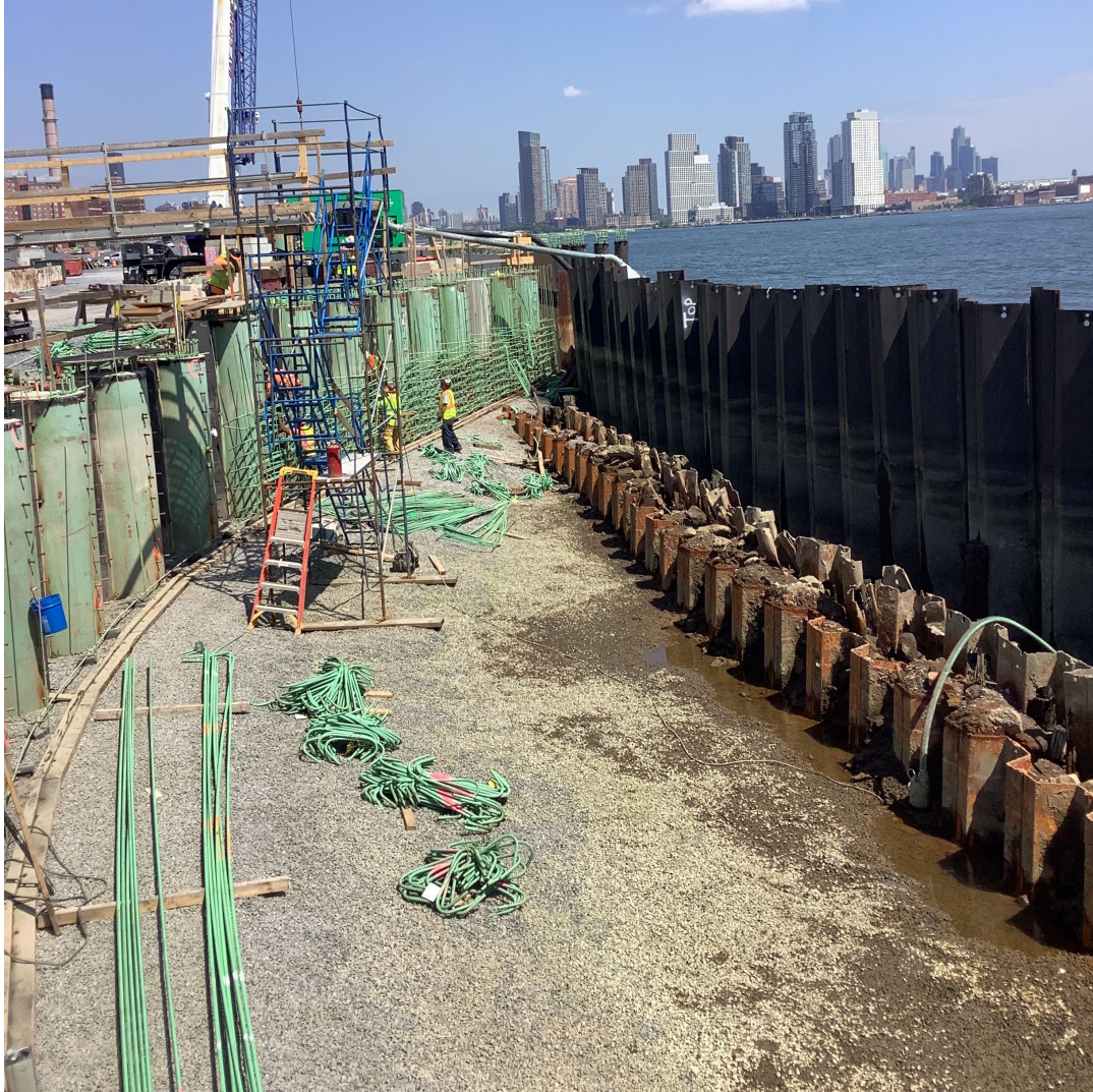
Northern embayment construction – August 2026
