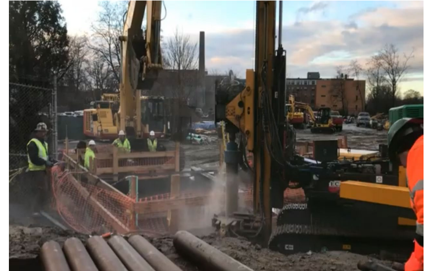
Example of drilled/micropile installation, via https://www.youtube.com/watch?v=a8VNRzrwyIU
