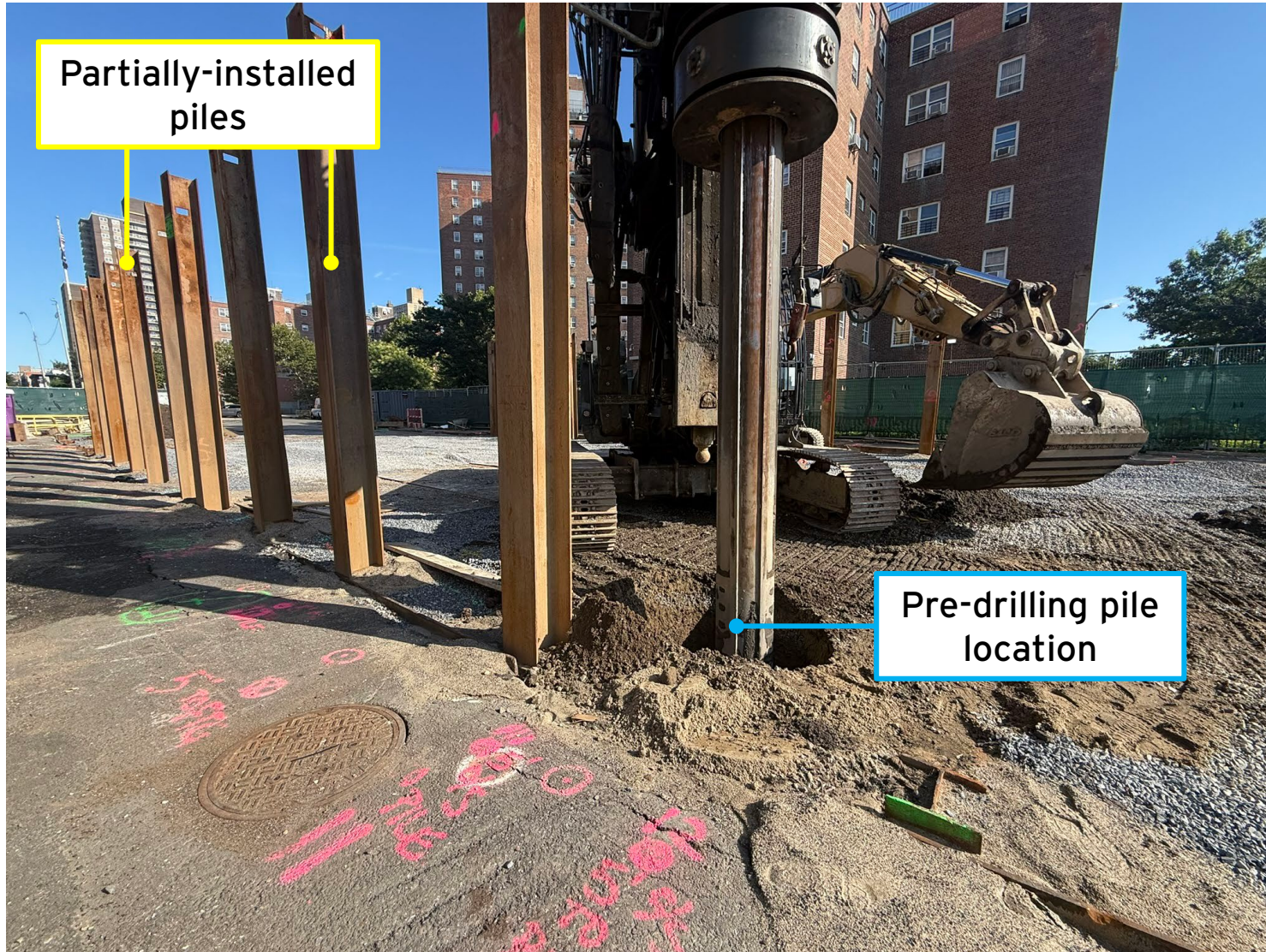
E. 10 th Street bridge pile installation – August 2026
