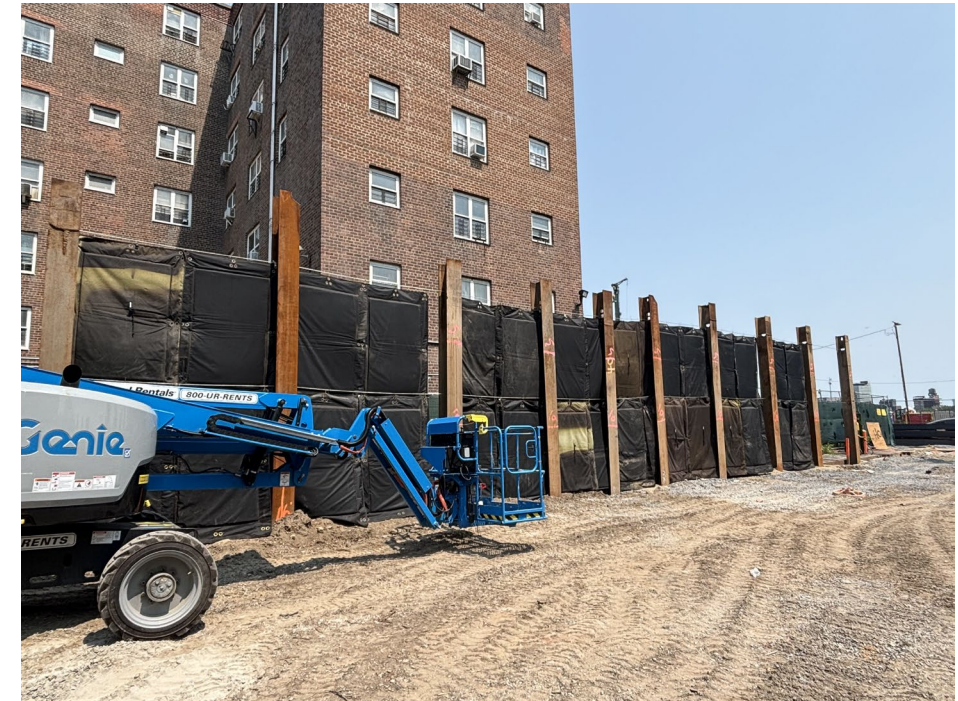
Noise mitigation blankets installed adjacent to bridge work area – August 2026
