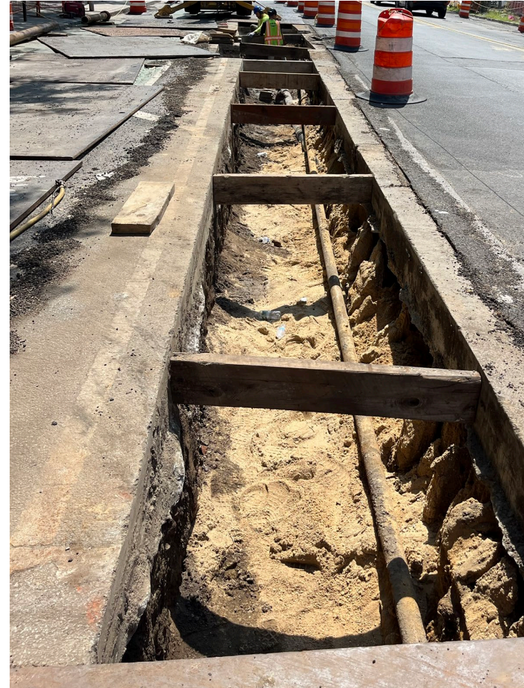
Gas main installation near E. 20 th Street – August 2026
