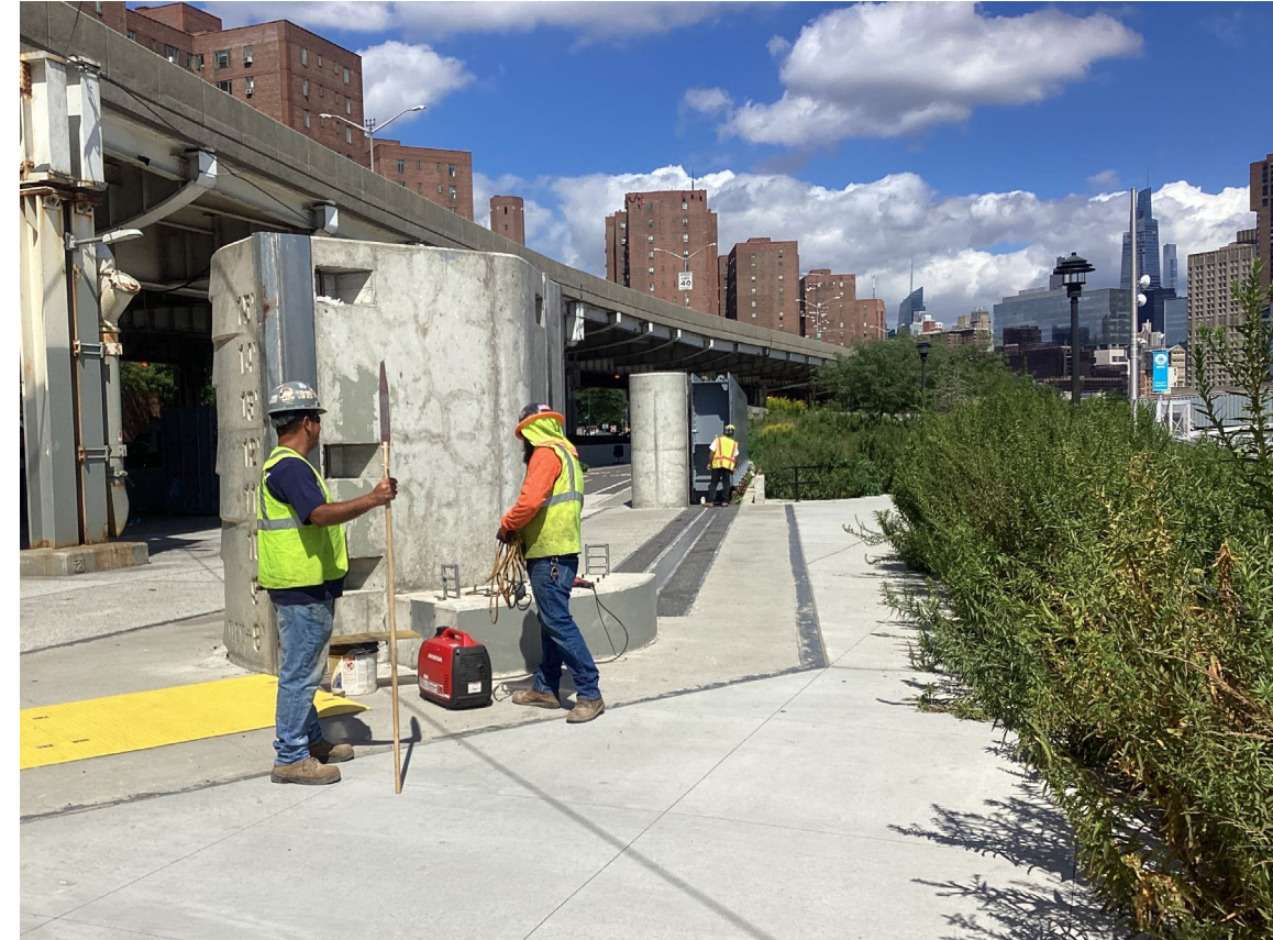
Punch list work ongoing in Stuyvesant Cove Park – August 2026
