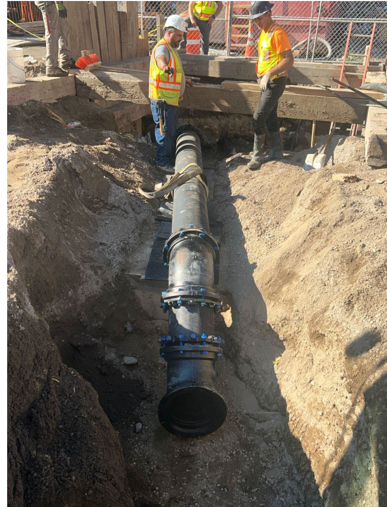
Water main installation in Delancey Street North – August 2026
