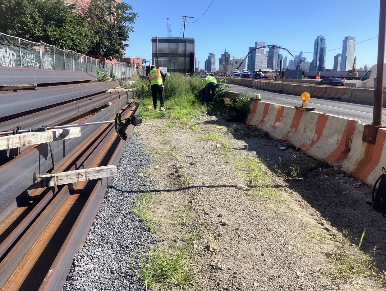
Performing site maintenance near E. 10 th Street bridge construction – August 2026
