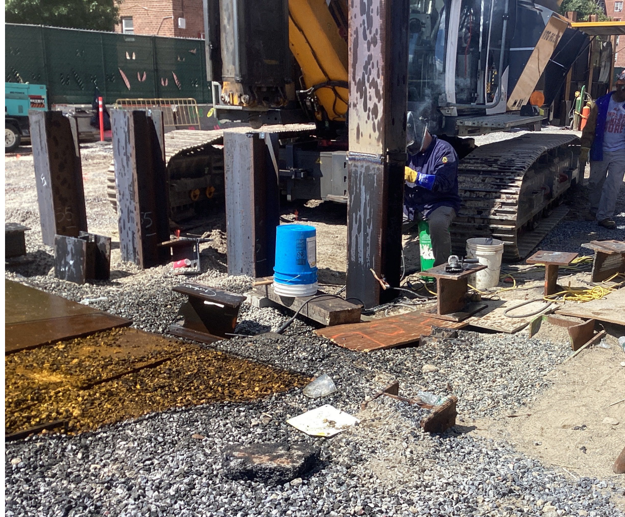
Bridge pile splicing (welding) – August 2026
