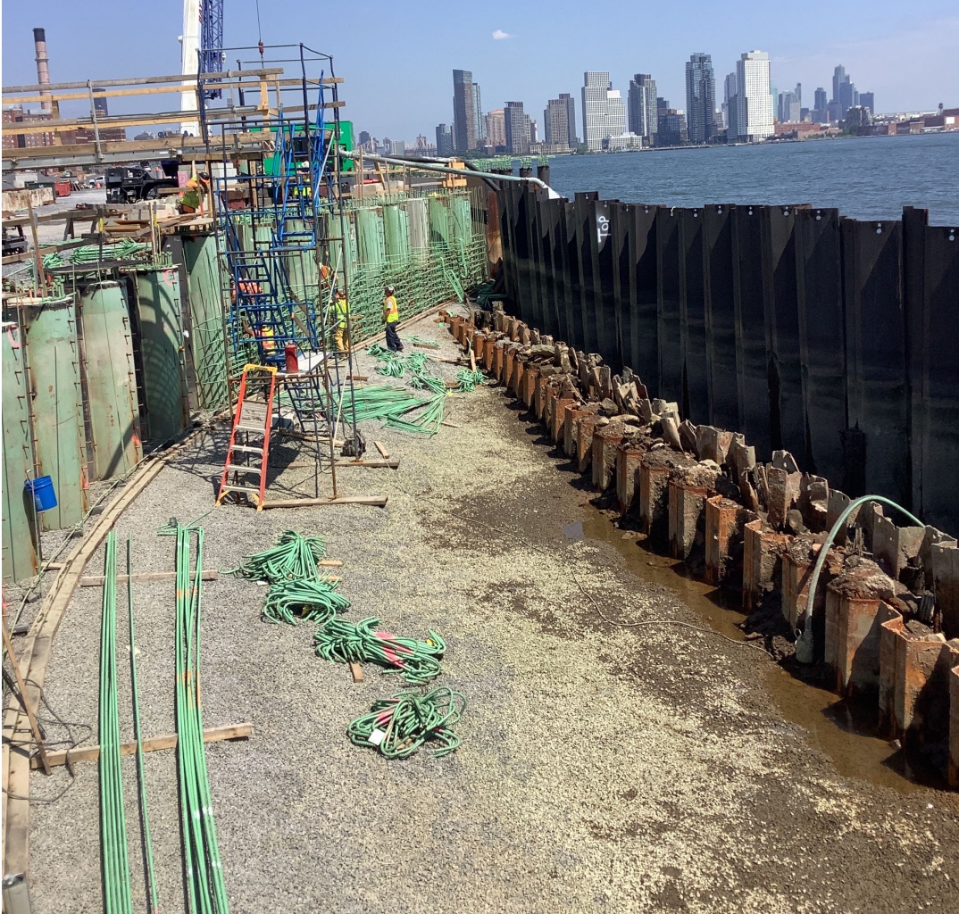
Northern embayment construction – August 2026
