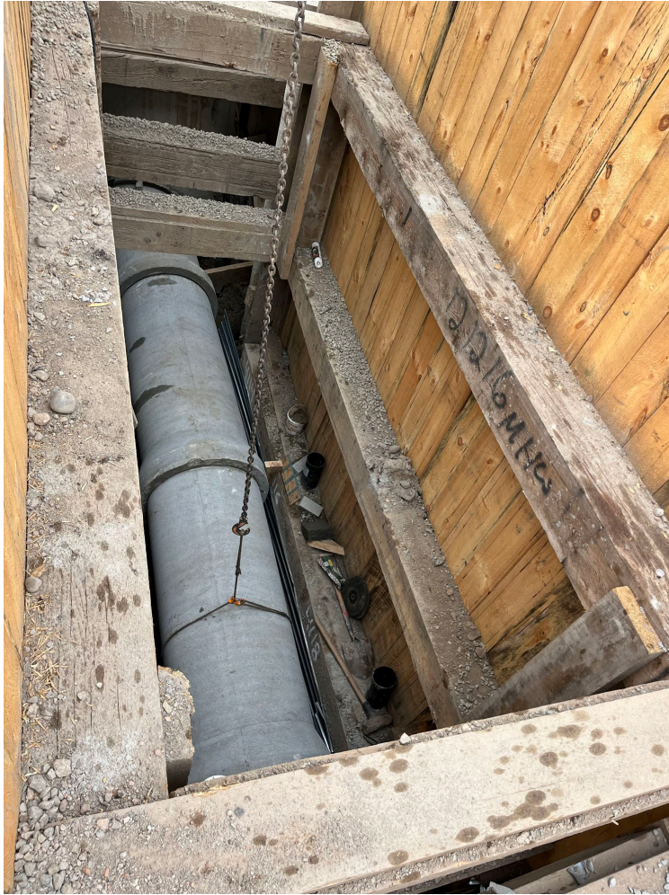
PC sewer installation in Columbia Street – August 2026
