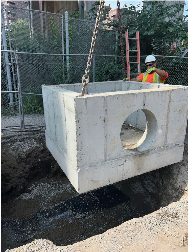
Catch basin installation in Delancey Street North – August 2026
