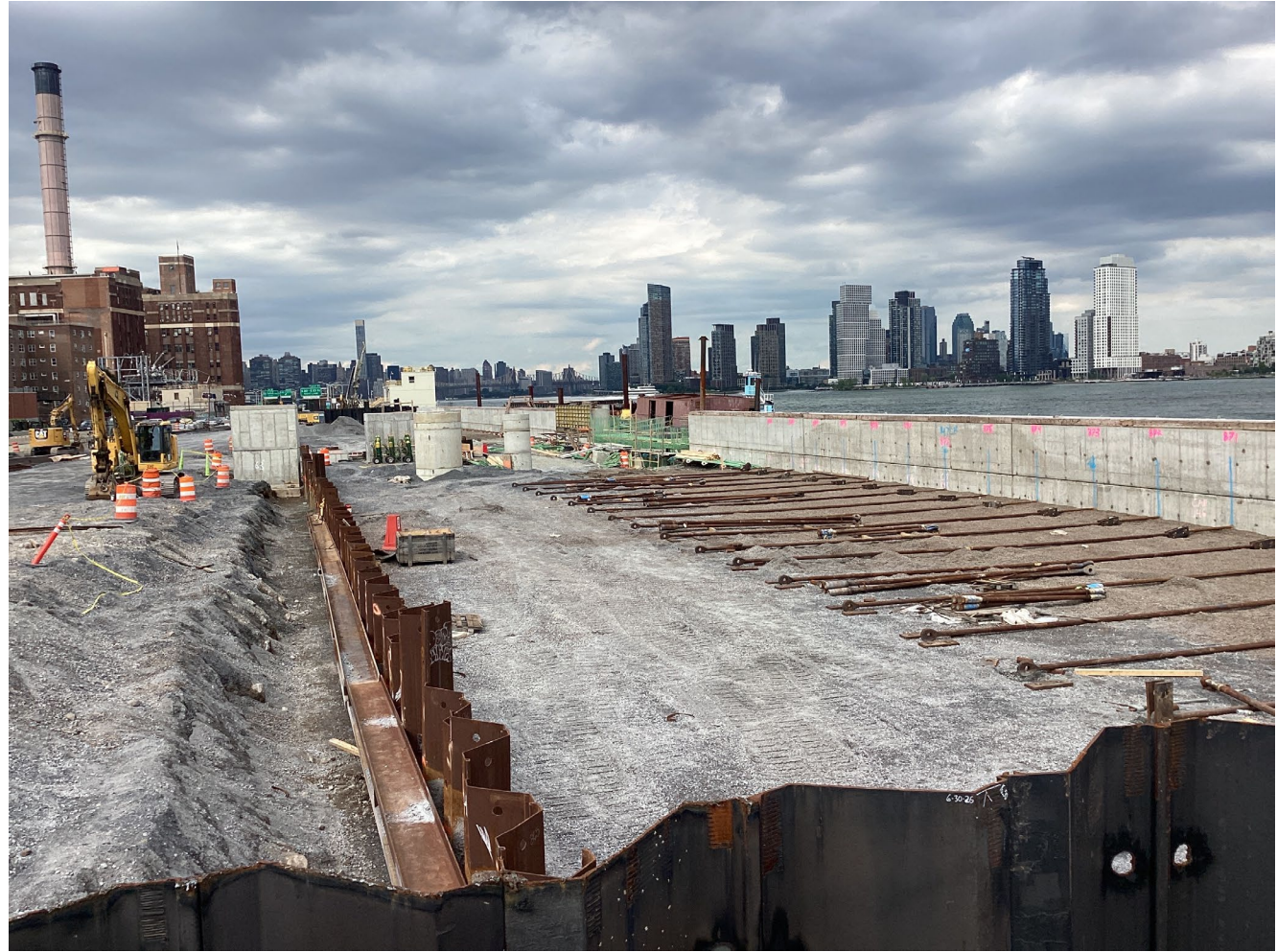
Buried floodwall (left), tie rods (middle), bulkhead wall (right) – August 2026
