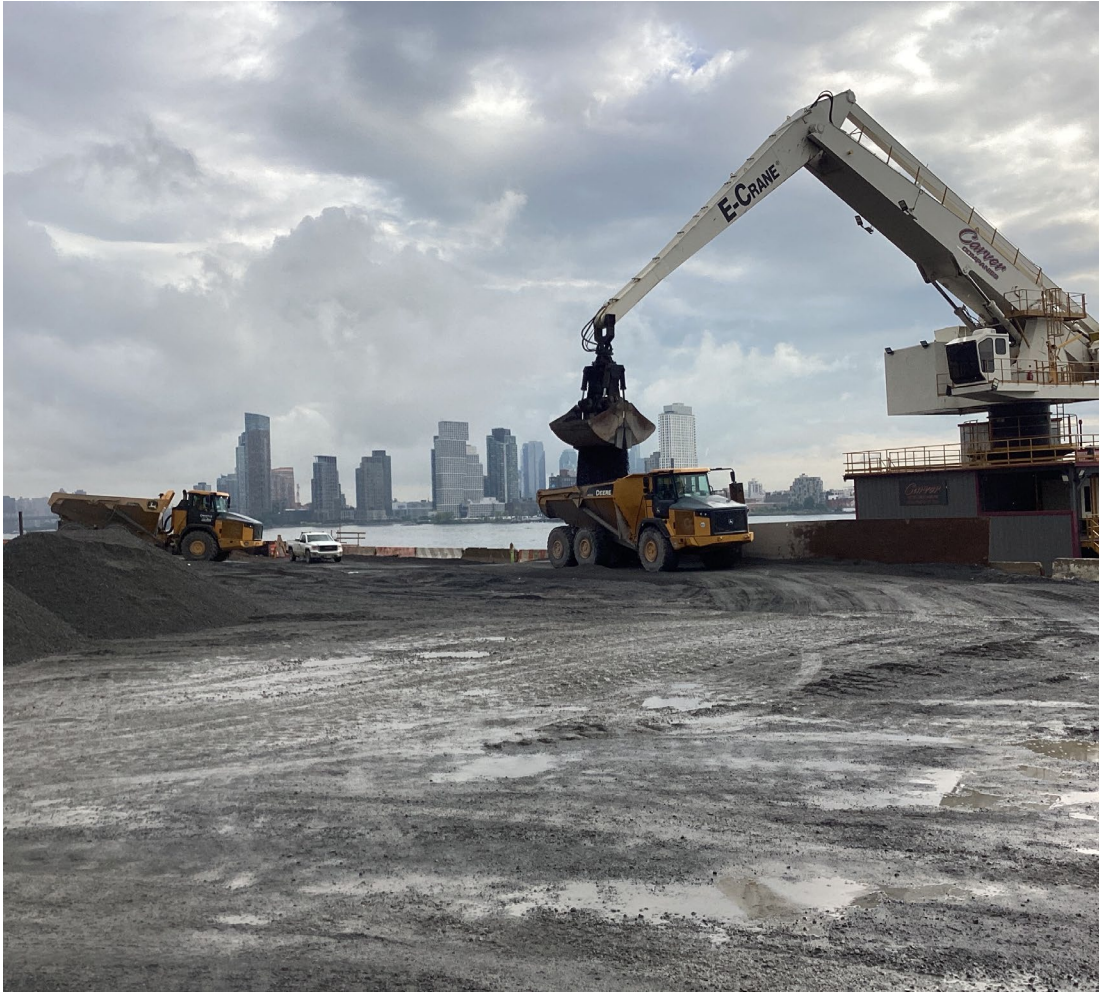
E-Crane loading clean fill via barge onto site – August 2026
