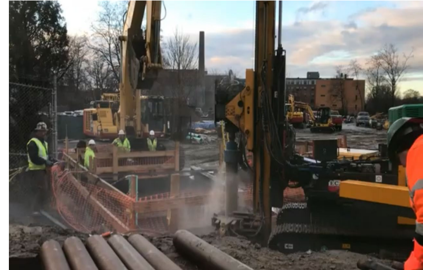
Example of drilled/micropile installation, via https://www.youtube.com/watch?v=a8VNRzrwyIU
