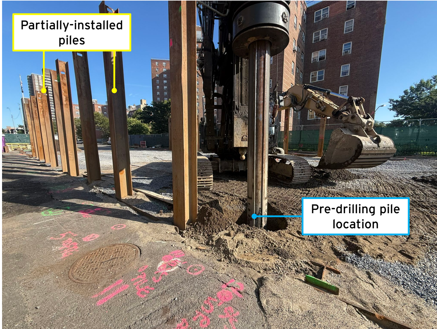
E. 10 th Street bridge pile installation – August 2026
