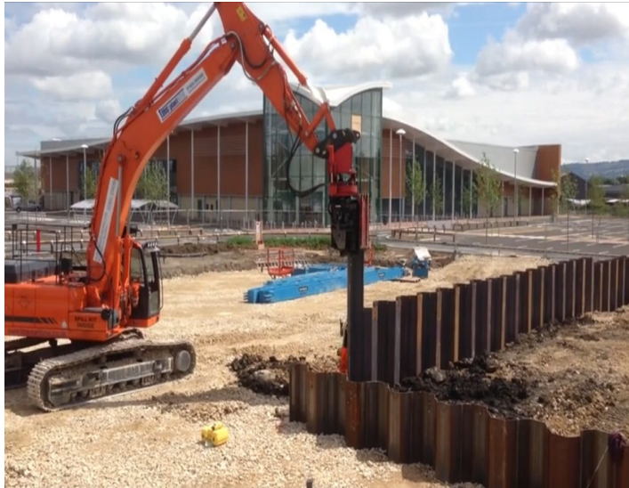
Example of vibratory sheet pile installation, via https://www.youtube.com/watch?v=A47OAosNnG4
