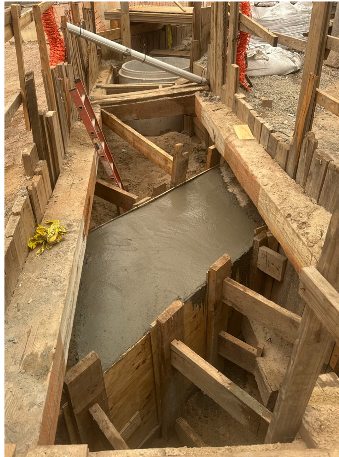
Steam main encasement in Columbia St. – July 2026
