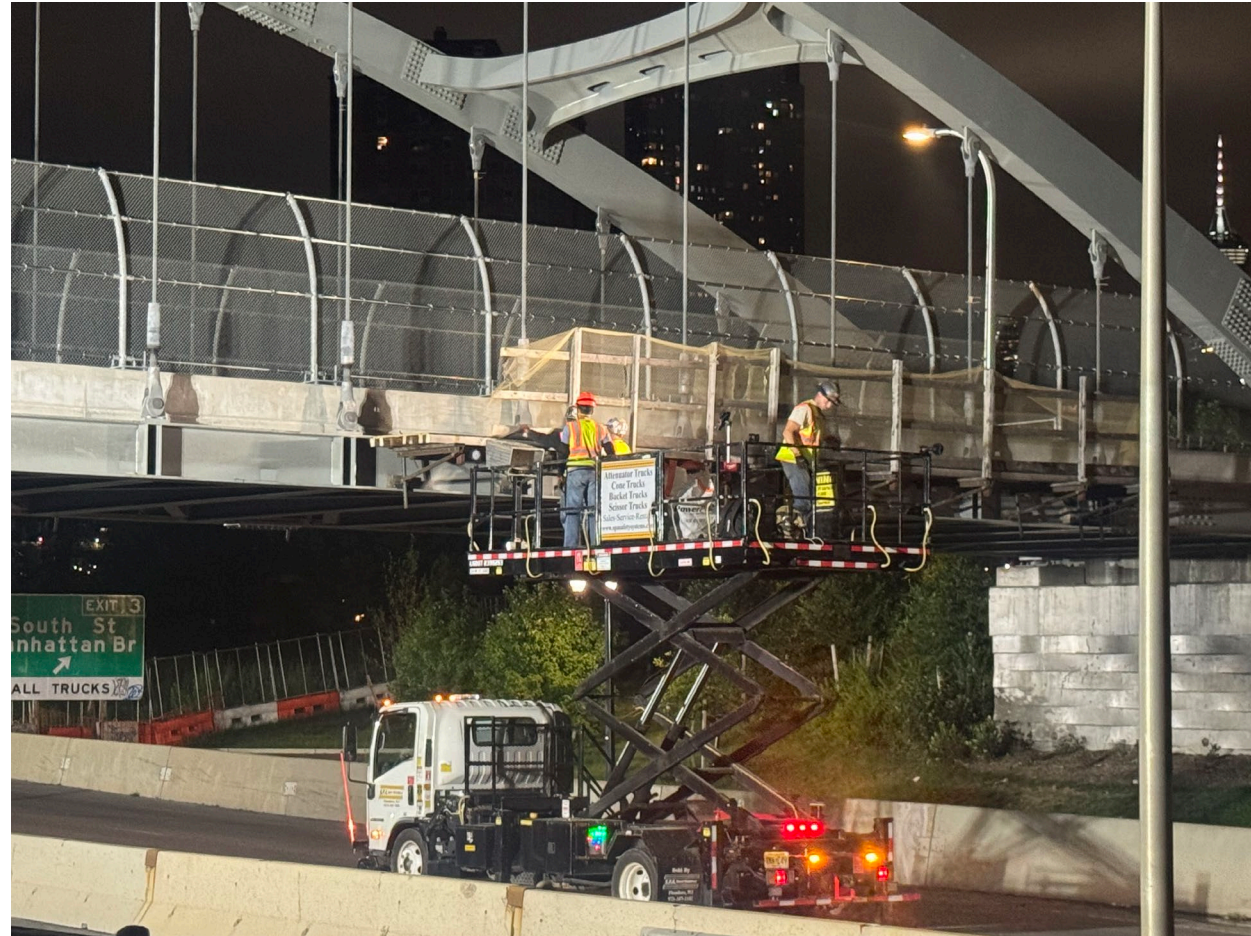
Removal of overhang protection materials from Corlears Hook Bridge – July 2026
