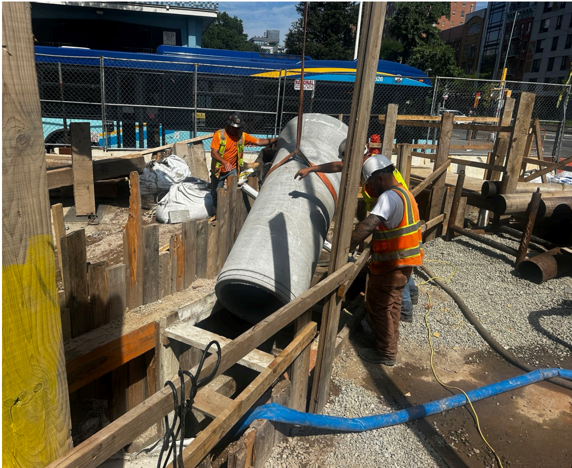
PC sewer installation in Columbia St. – July 2026
