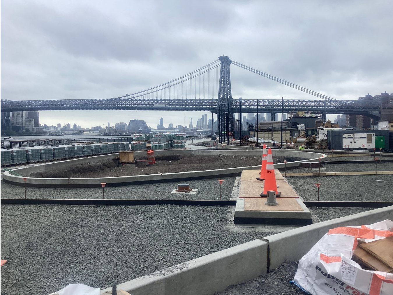
Curb formwork north of Fields 3 & 4 – July 2026
