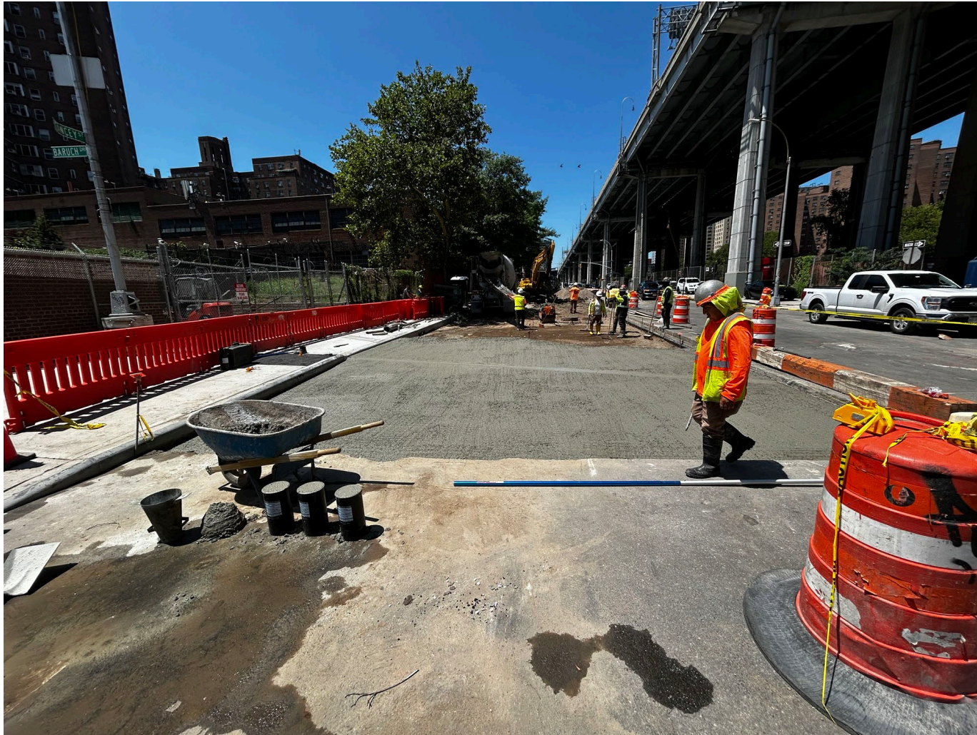
Final restoration in Delancey Street South – July 2026
