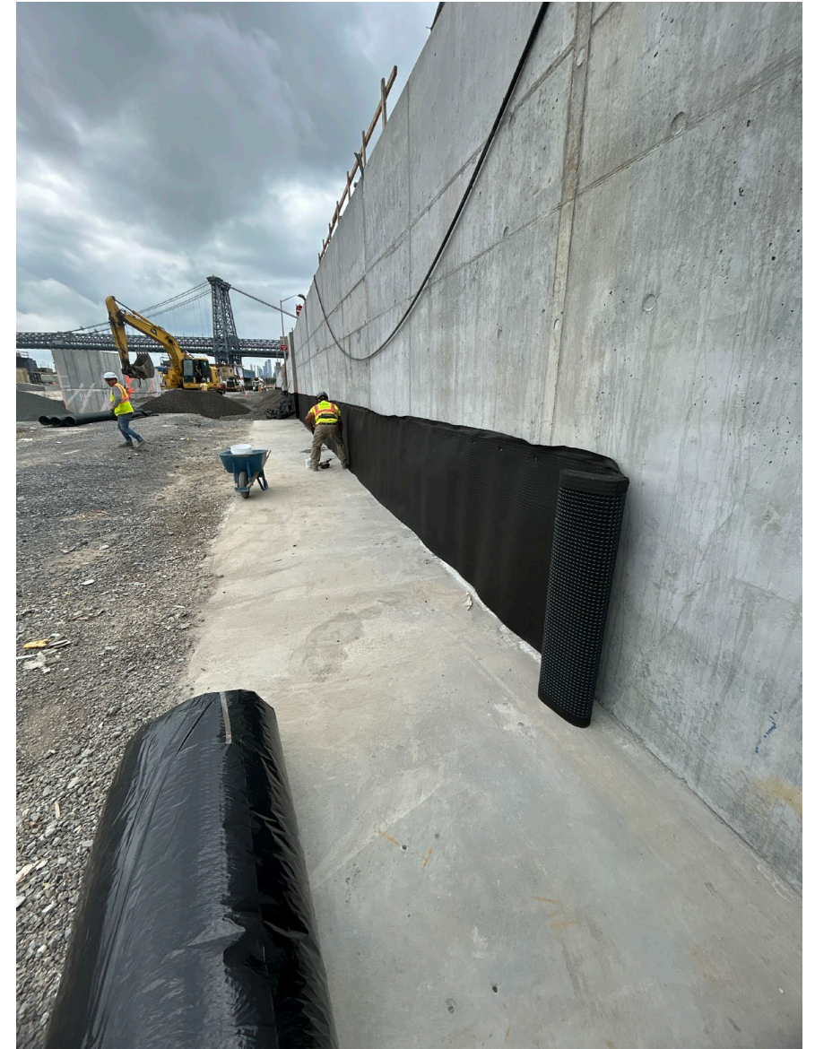
E. Houston Street retaining wall construction – July 2026
