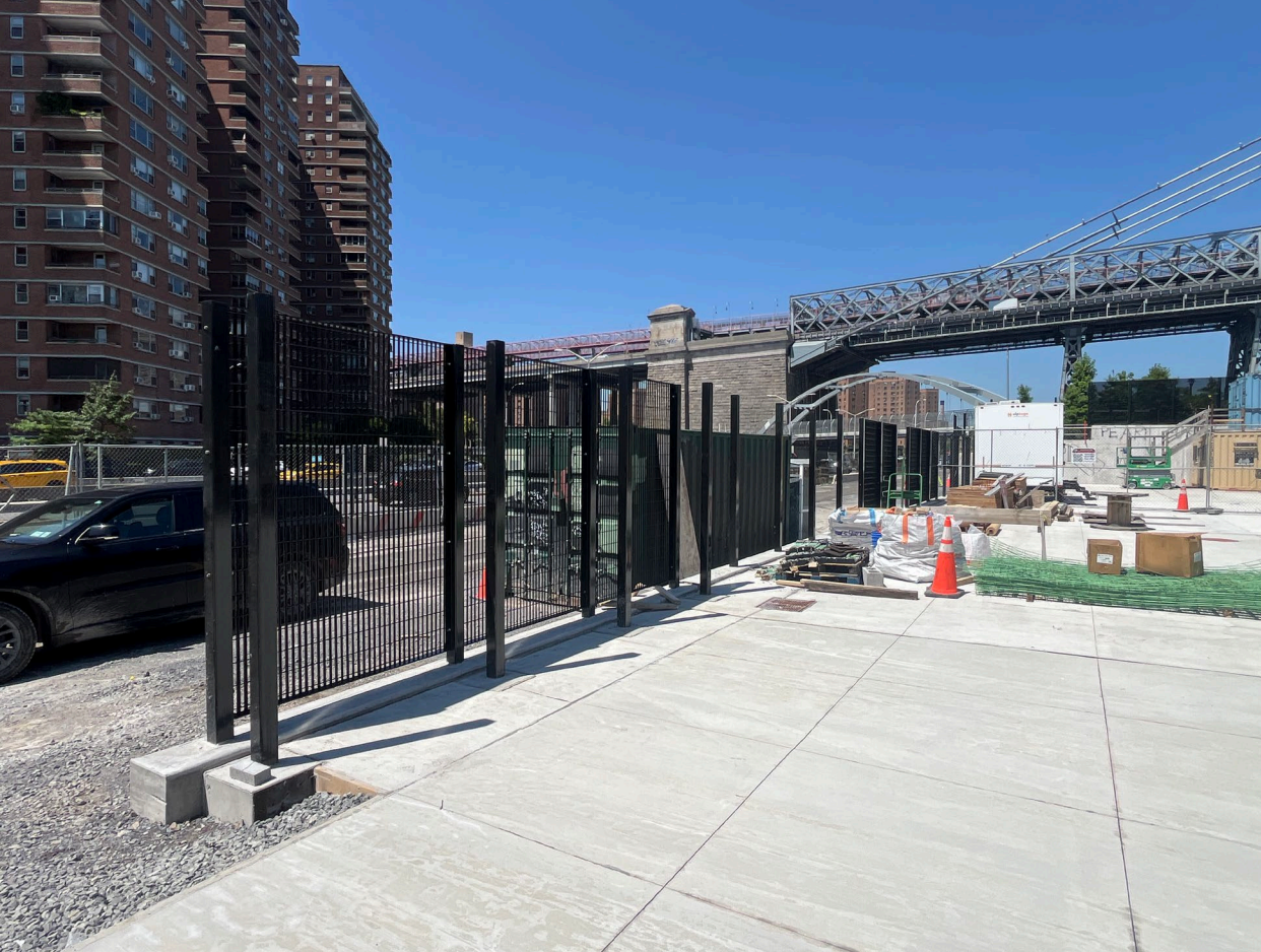
Privacy fencing installation at Parks M&O facility at Grand Street (M&O2) – July 2026
