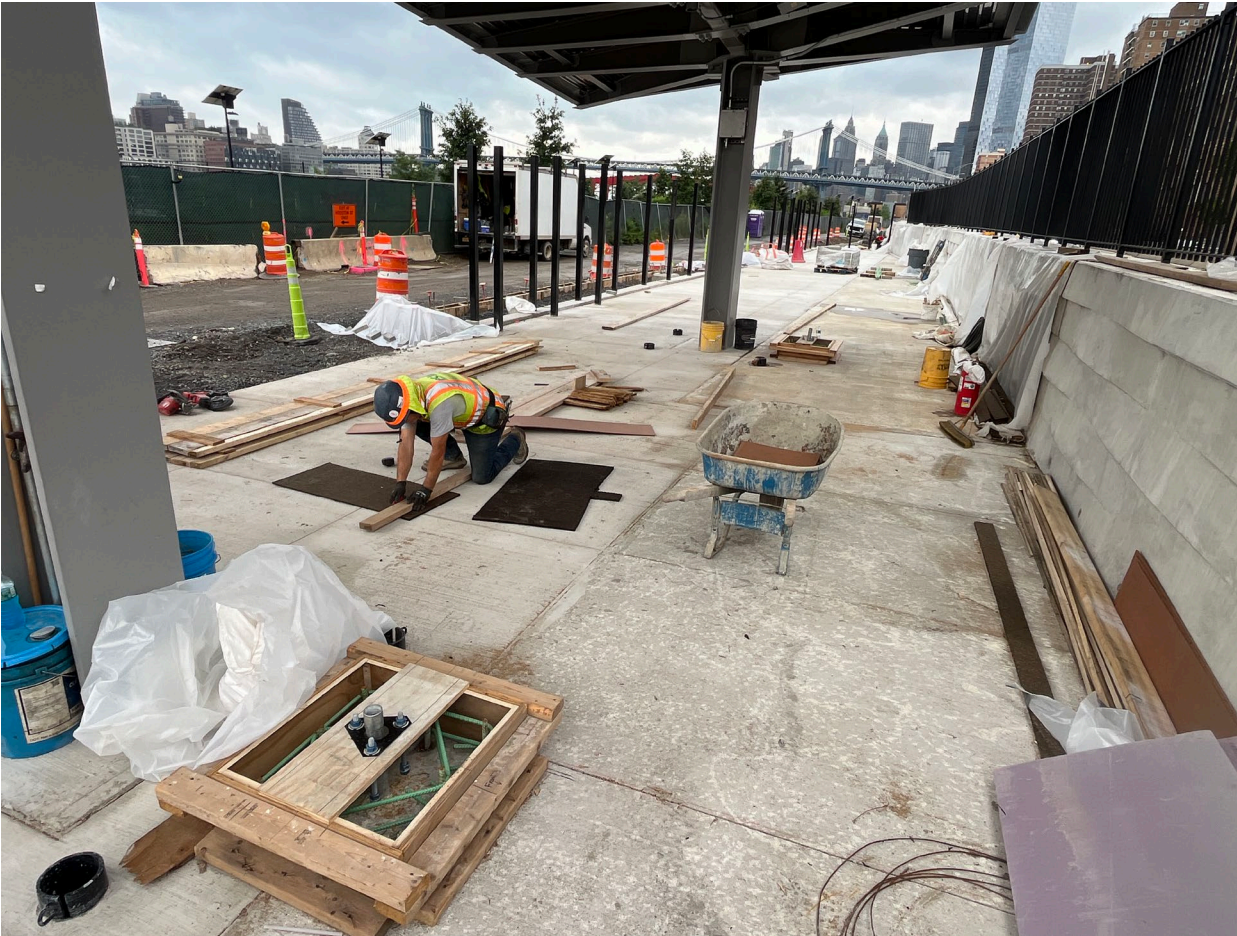
Vehicle parking area at Parks M&O facility near Pier 42 (M&O1) – July 2026
