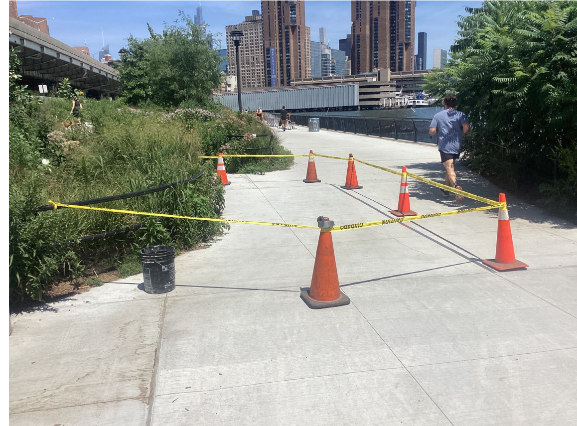
Punch list work ongoing in Stuyvesant Cove Park – July 2026
