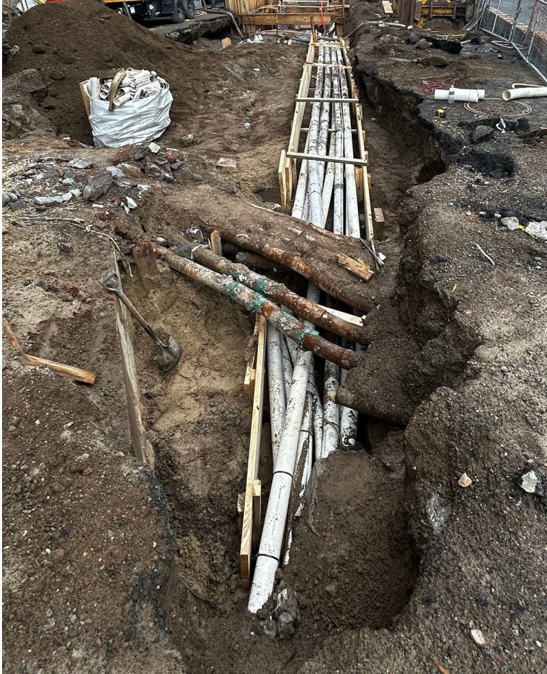
Utility relocation in Delancey St. N – July 2026
