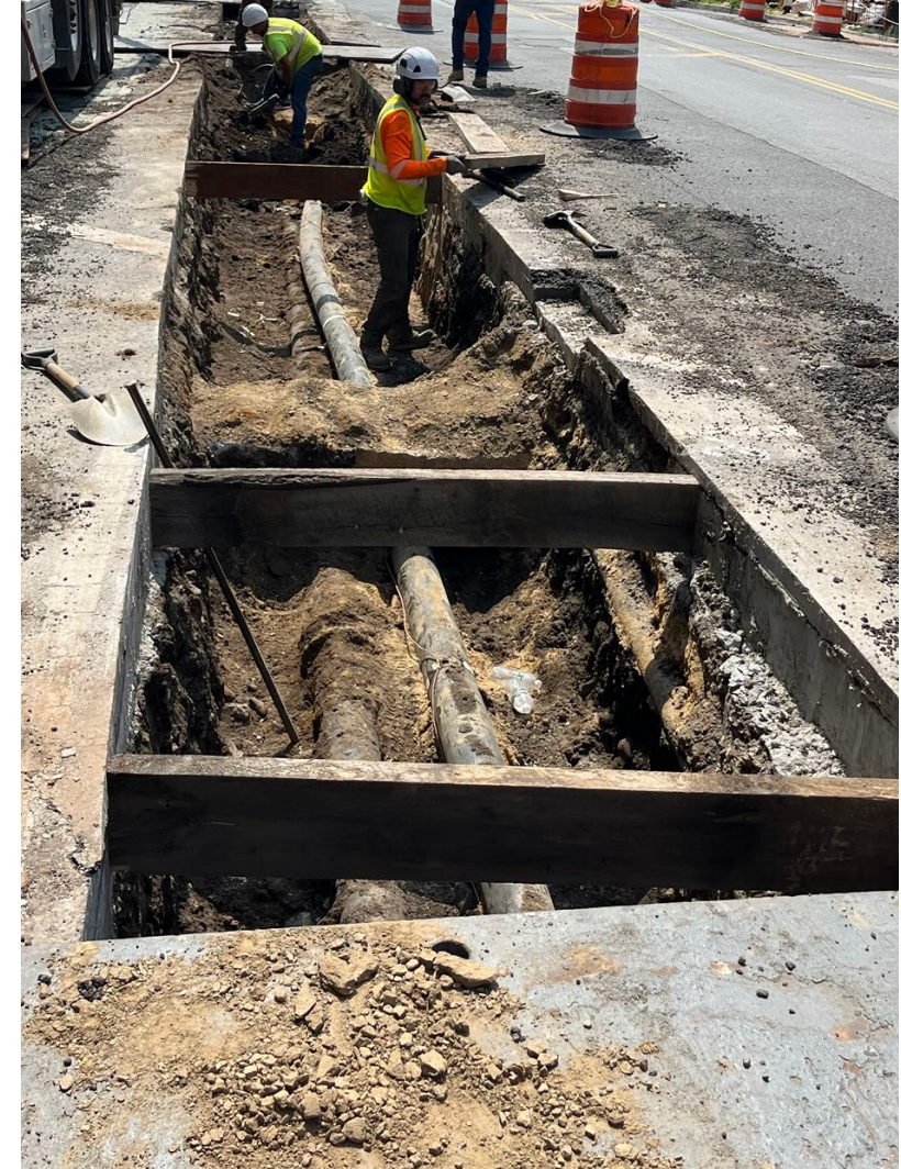
Excavation for gas main relocation – July 2026
