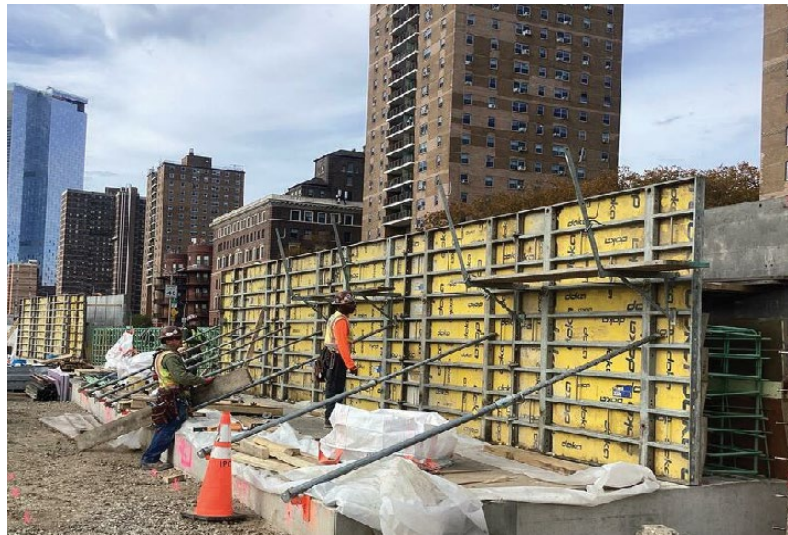
Southern floodwall formwork – December 2025
