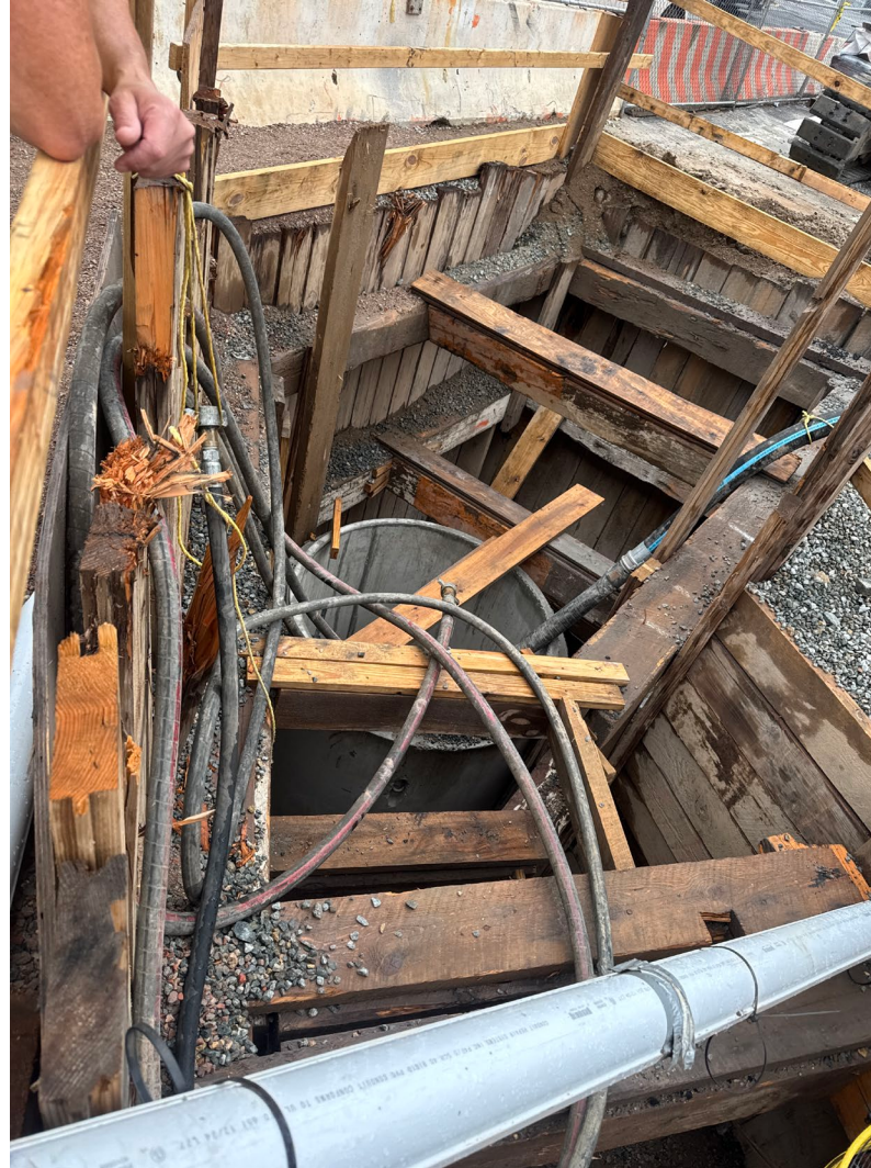
PC sewer installation in Columbia Street – July 2026
