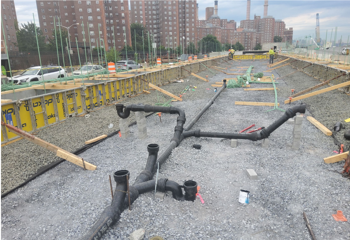
Foundation formwork and plumbing fixtures installed for future track house – June 2026
