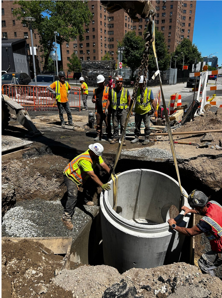
Precast manhole installation in Delancey St. N – June 2026
