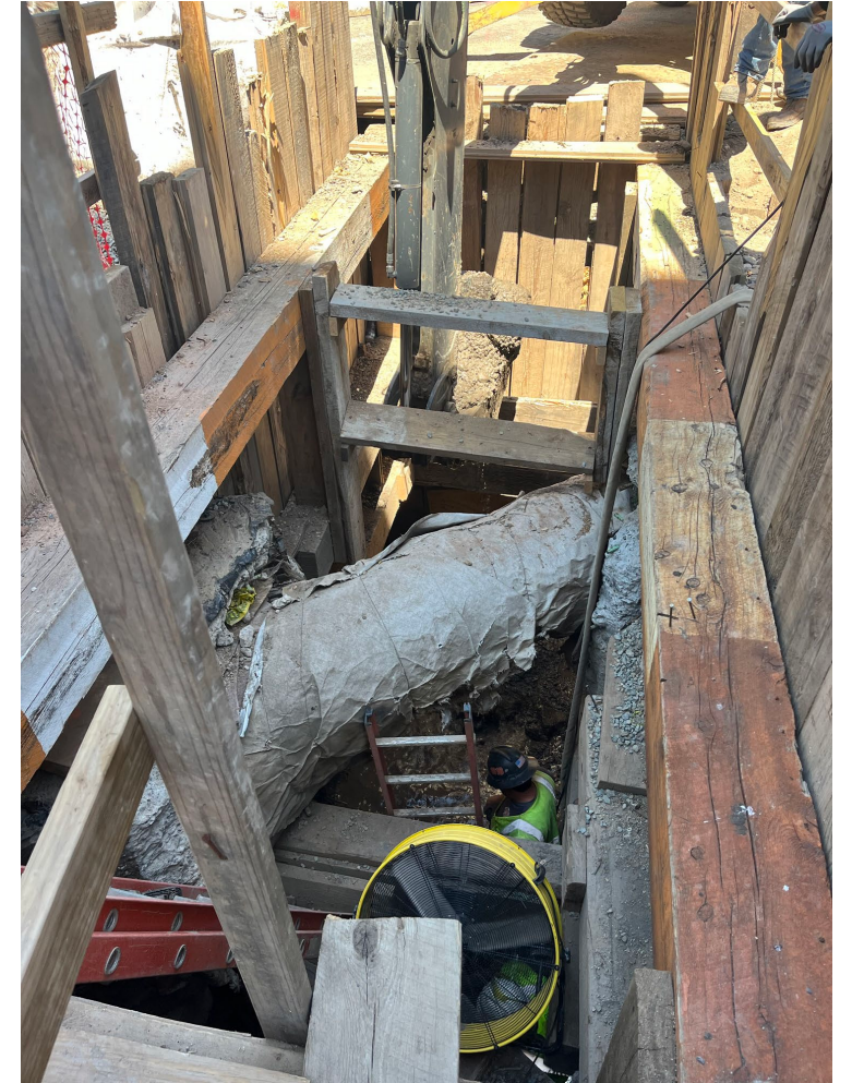
Excavation and support for PC sewer construction in Columbia Street – June 2026
