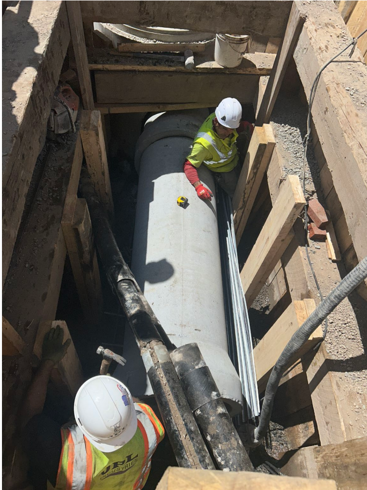
PC sewer installation in Delancey St. N – June 2026
