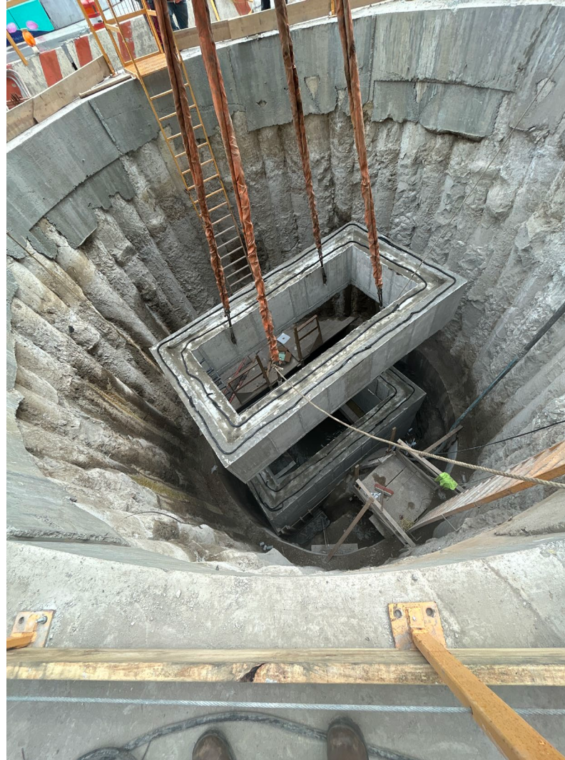
Installation of precast riser into deep drop manhole at Delancey St. N and Baruch Drive – May 2026
