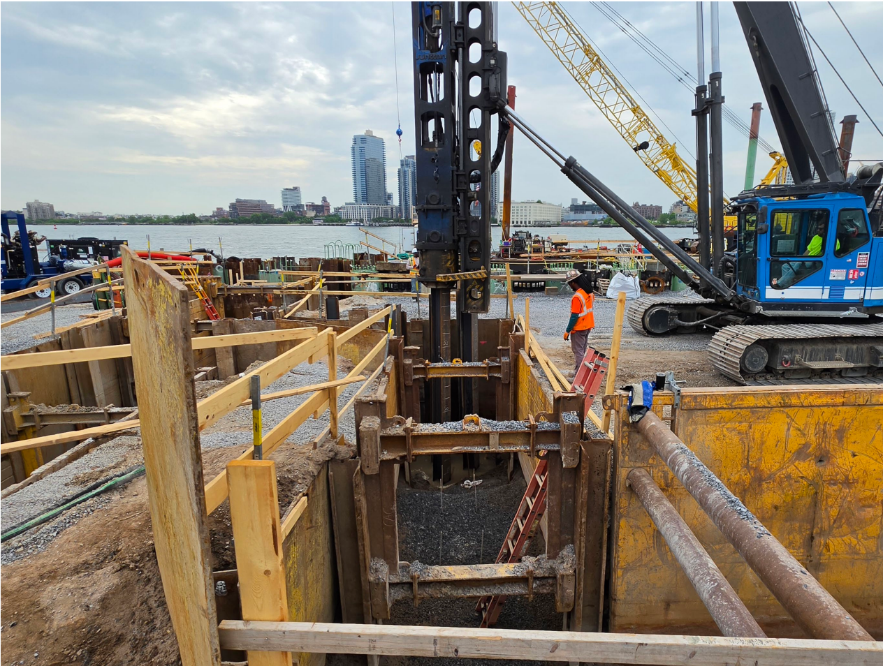
Installation of H-piles for sewer support near track area – June 2026
