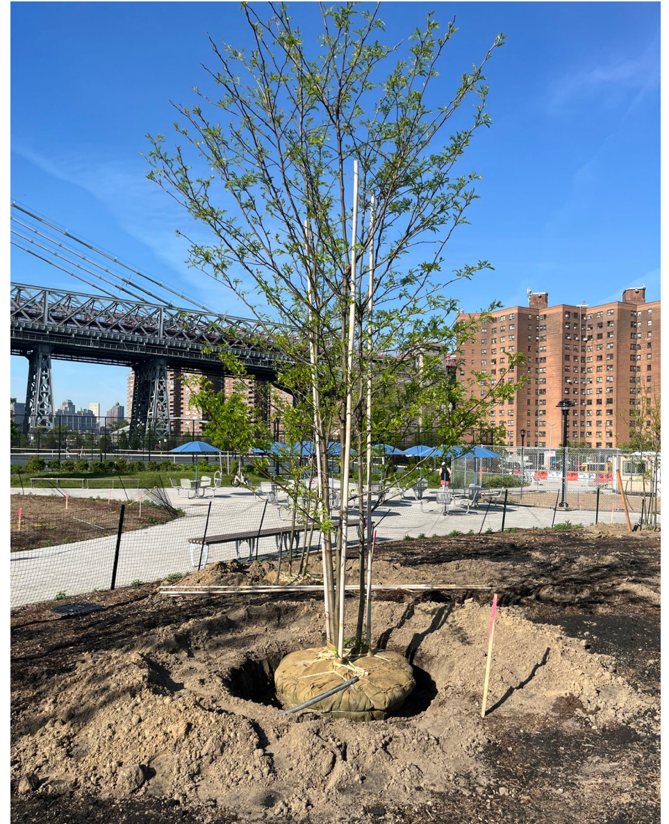
Tree installation near tennis courts and esplanade– June 2026
