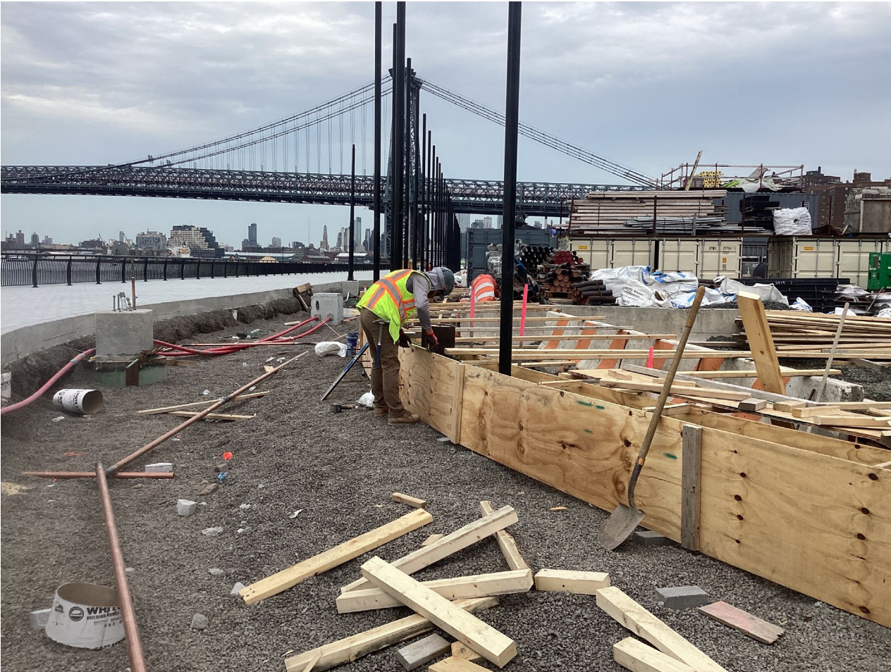
Forming fence and curb line for Field 4 – June 2026
