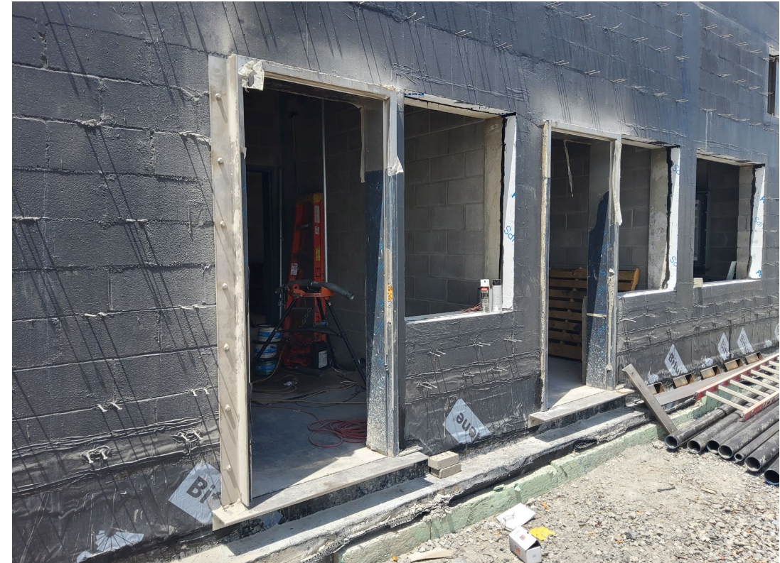
Tennis building construction – June 2026
