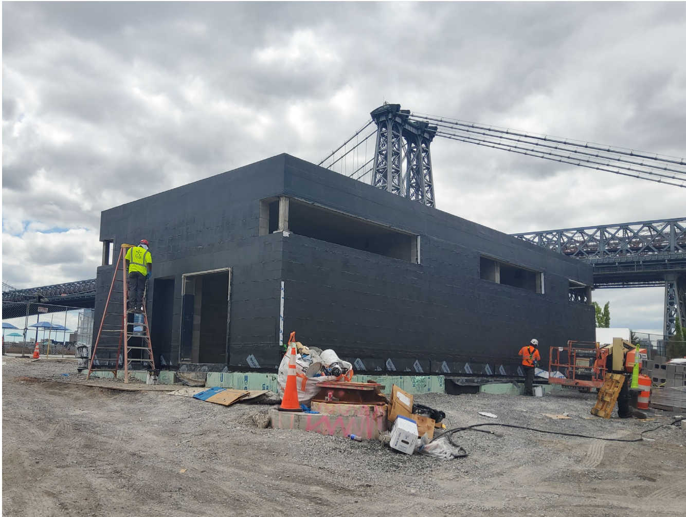
Waterproofing applied to tennis building – June 2026
