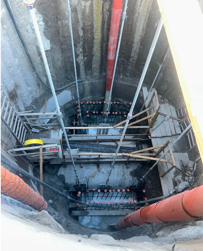
Construction of deep drop manhole at Delancey St. N and Baruch Drive – May 2026
