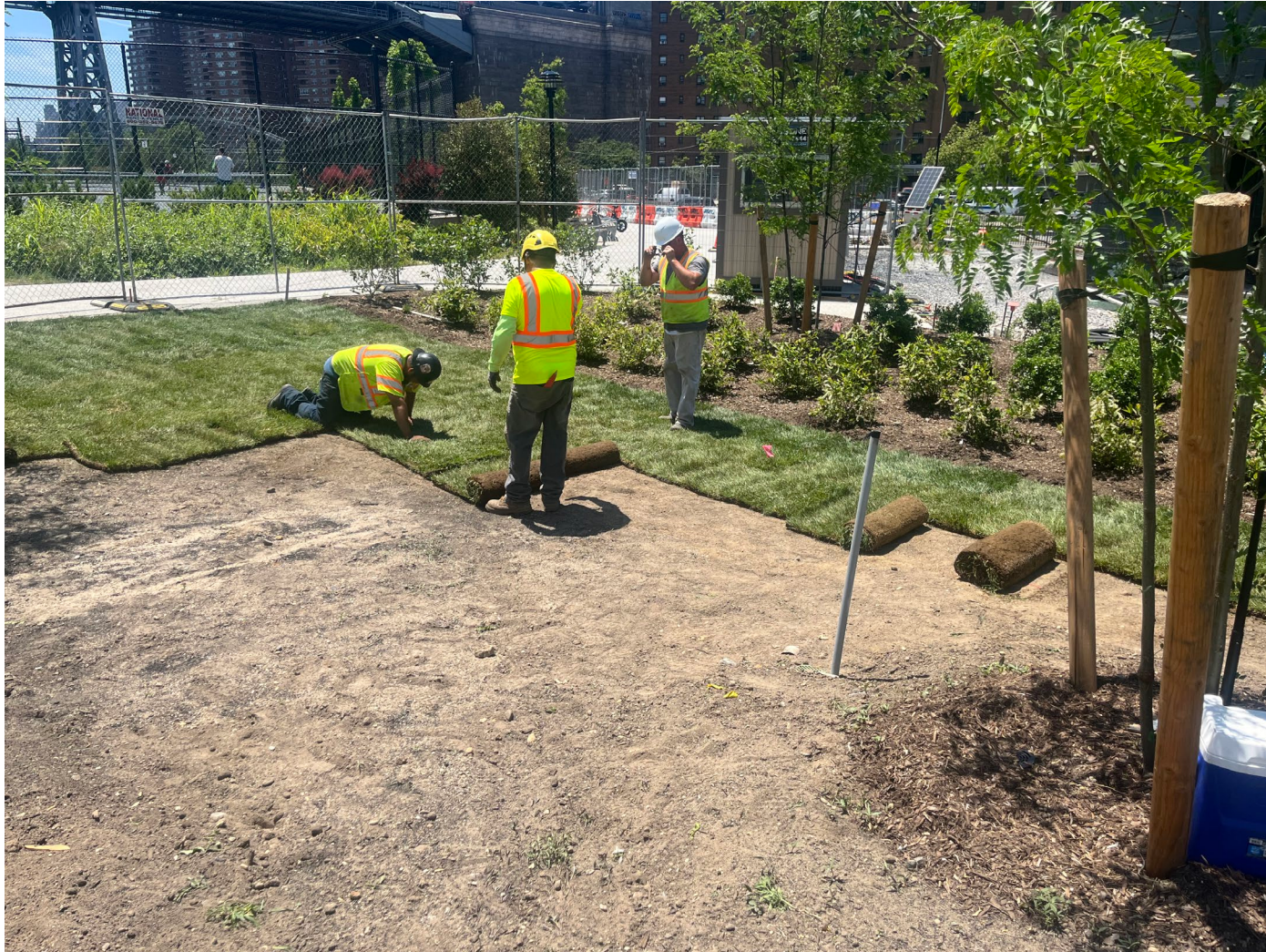
Sod installation near tennis courts – June 2026
