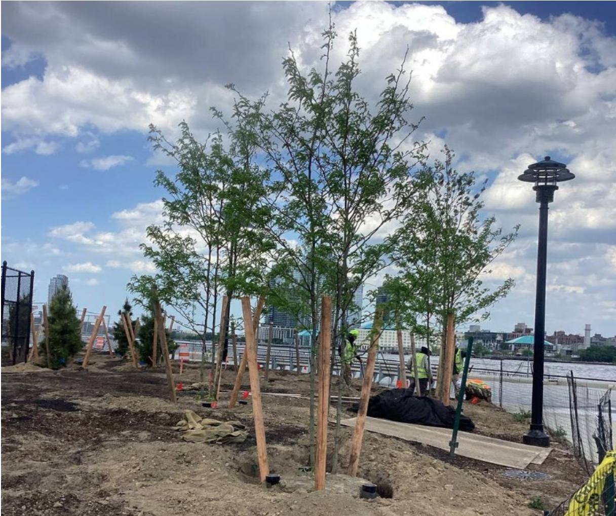
Irrigation and planting installation near Tennis Courts – May 2026
