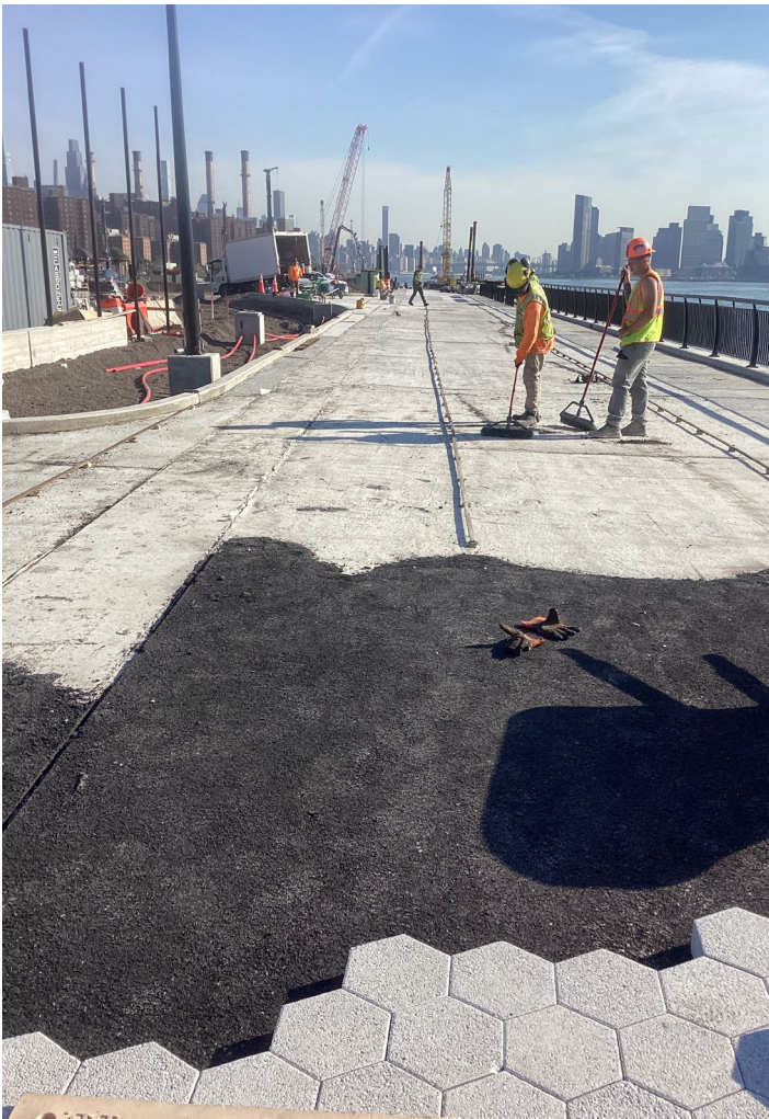
Esplanade paver base installation near Fields 3 & 4 – May 2026
