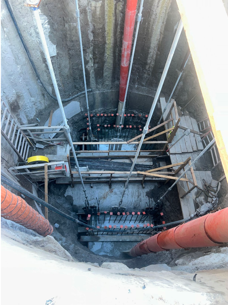
Construction of deep drop manhole at Delancey St. N and Baruch Drive – May 2026
