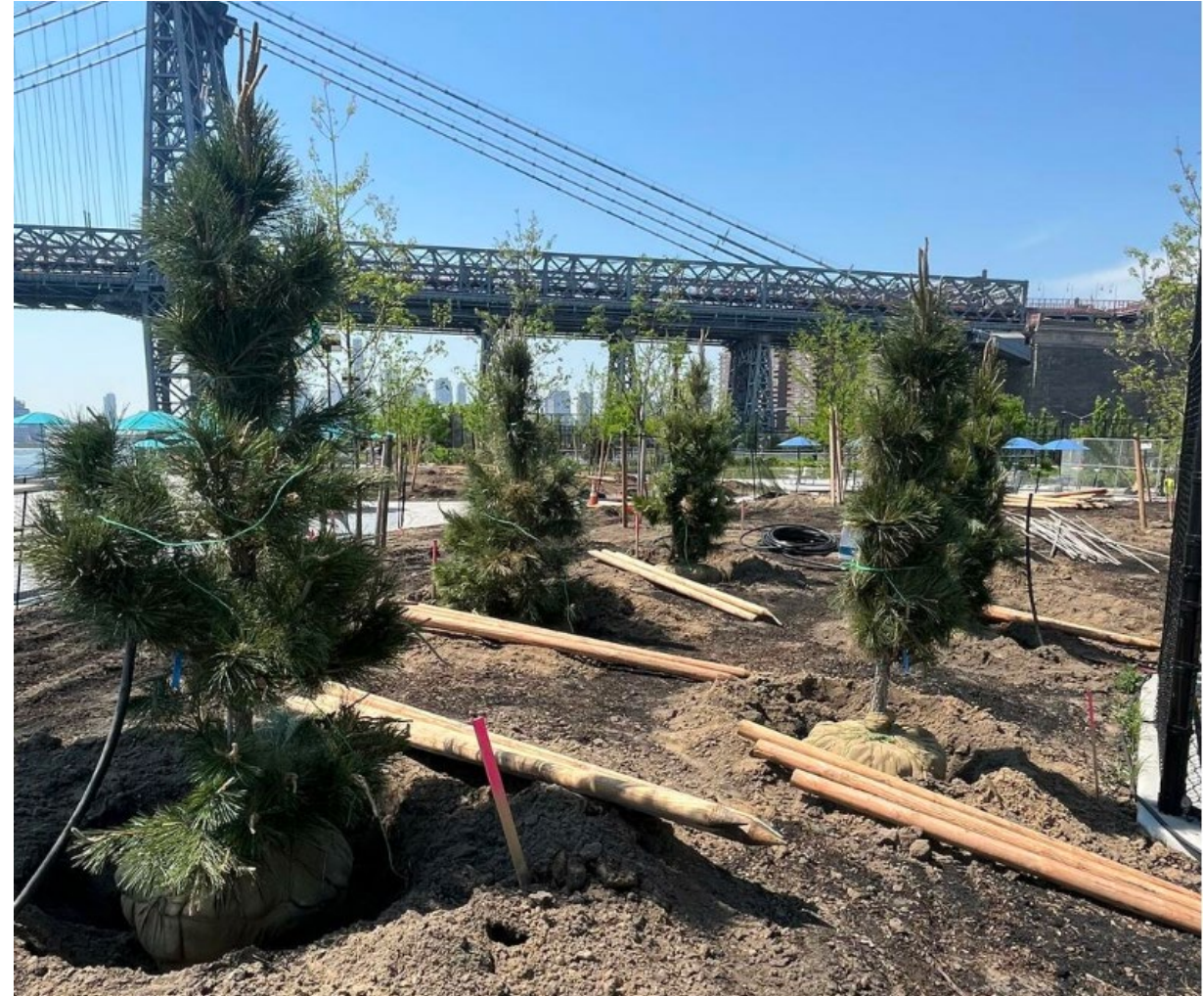
Tree installation near Tennis Courts – May 2026
