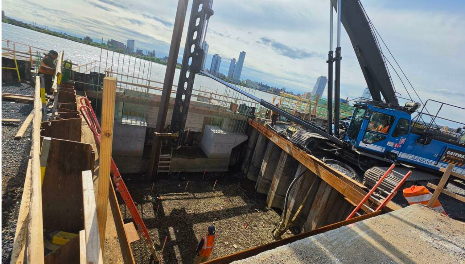
Construction of sewer outfall near Track and Field – May 2026
