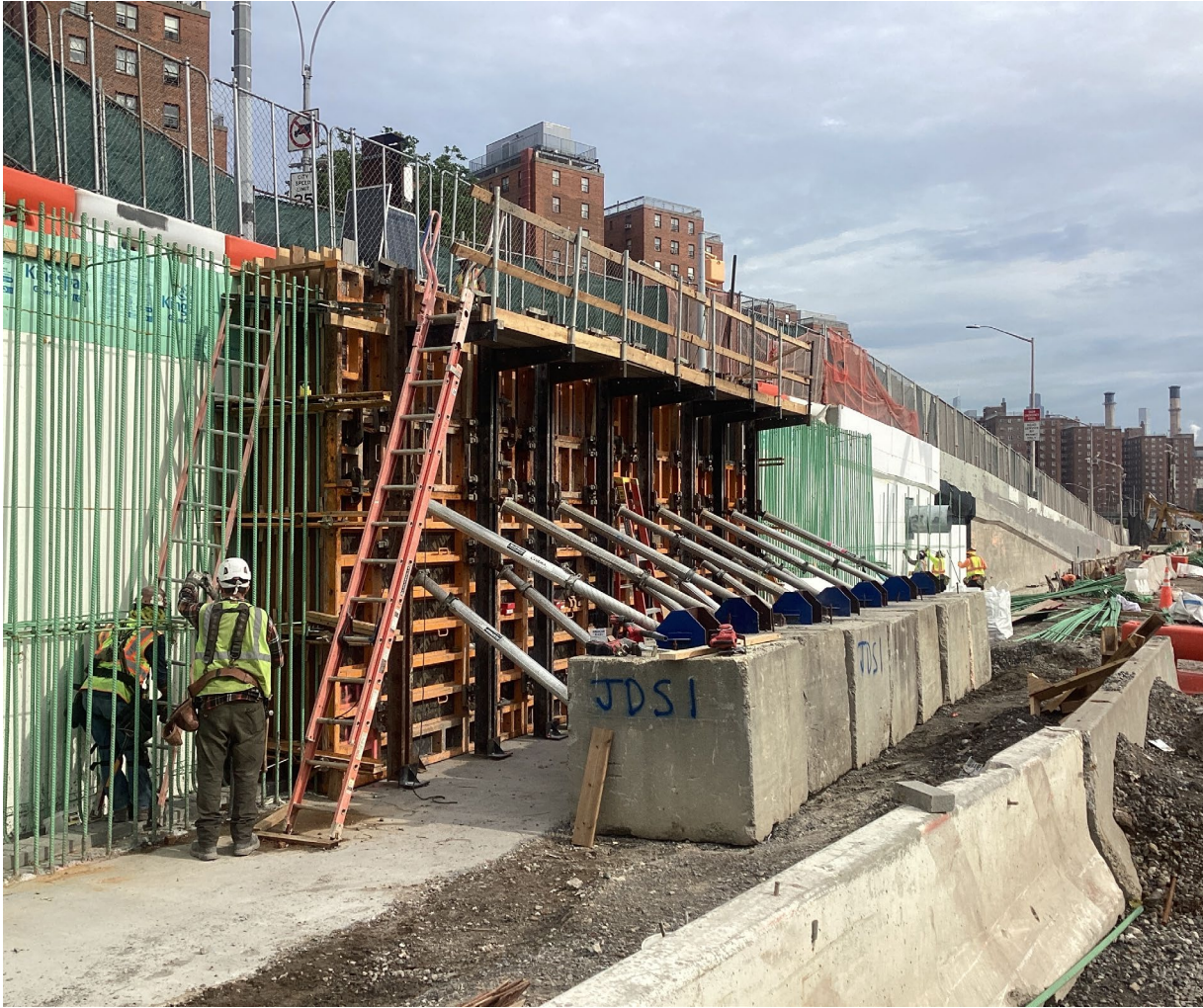
Installation of formwork for Houston St. retaining wall – May 2026
