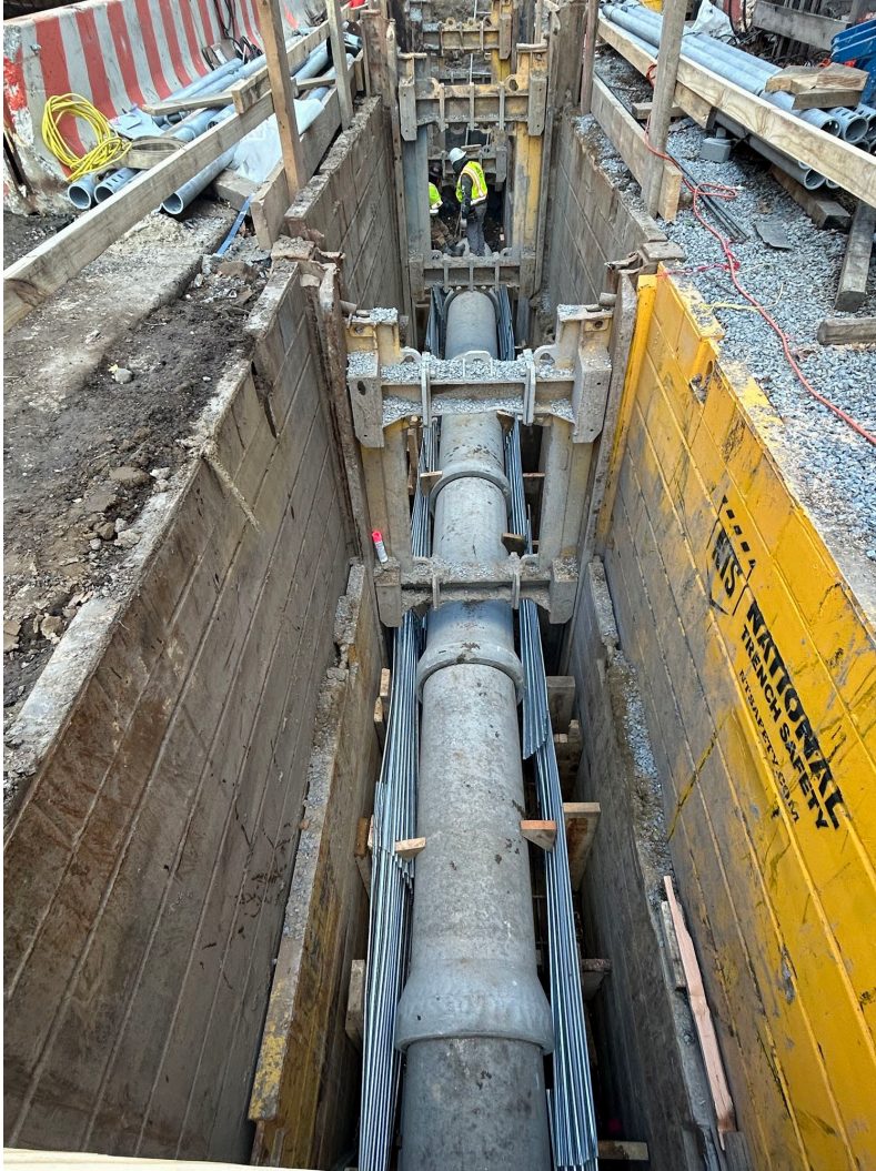
PC sewer installation in Lewis St. & Delancey St. S – December 2025
