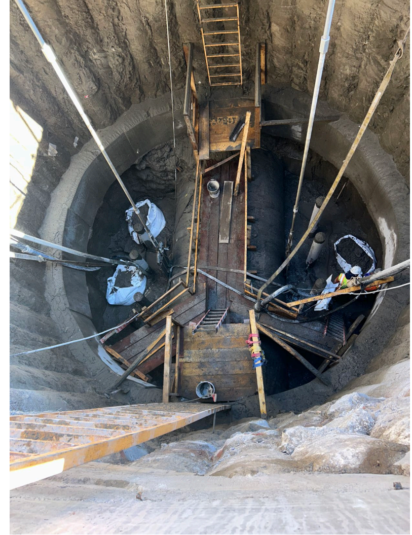
Deep drop manhole in Delancey St. North – April 2026
