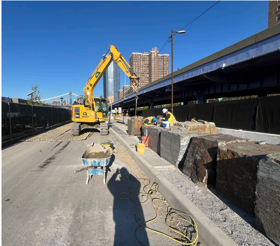
Installation of stone features adjacent to Pier 42 – April 2026
