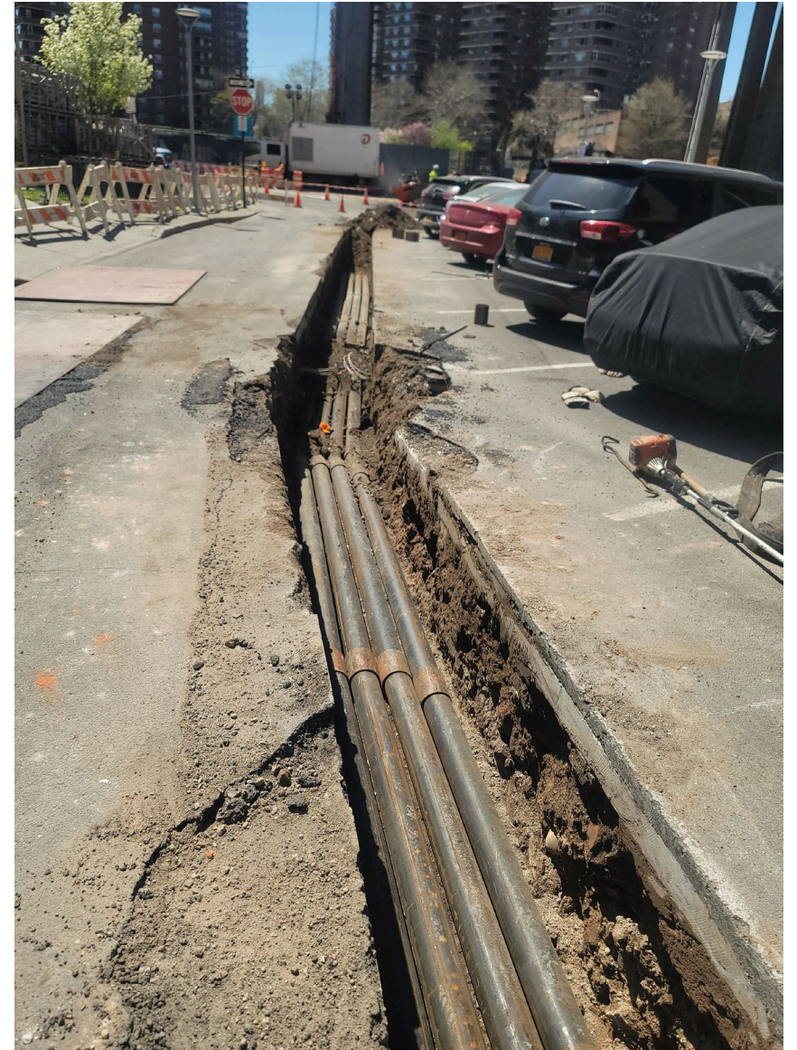
Con Edison conduit installation on Delancey St. North – April 2026
