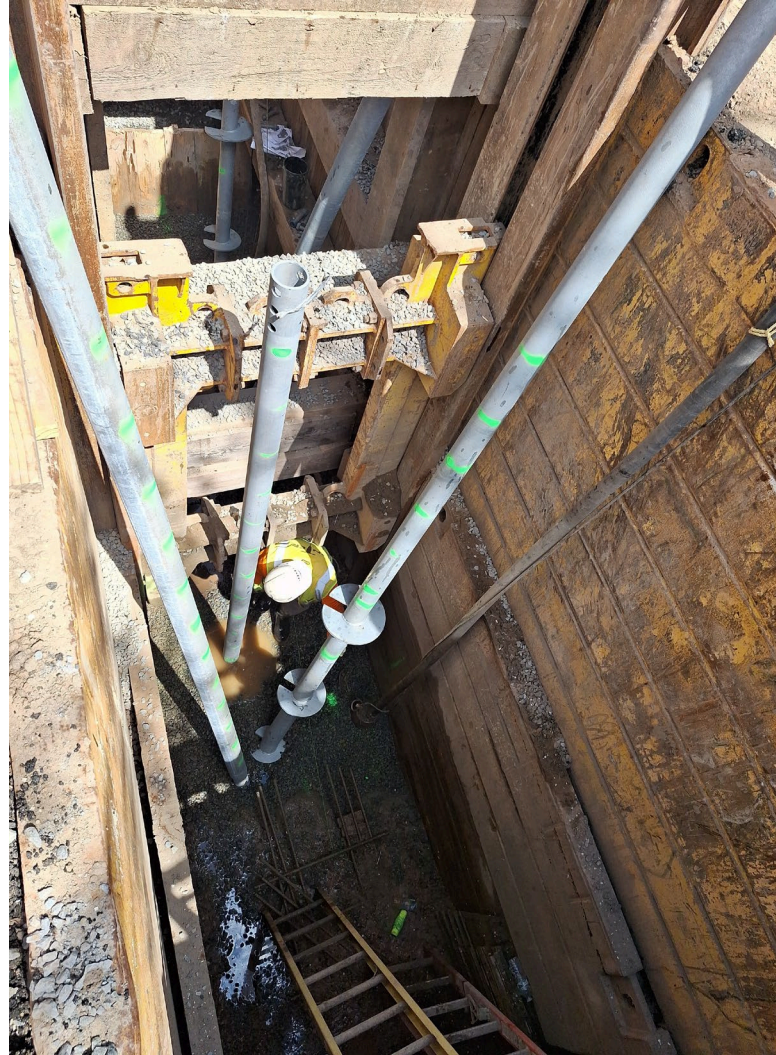
Helical pile installation in Delancey St. South – April 2026
