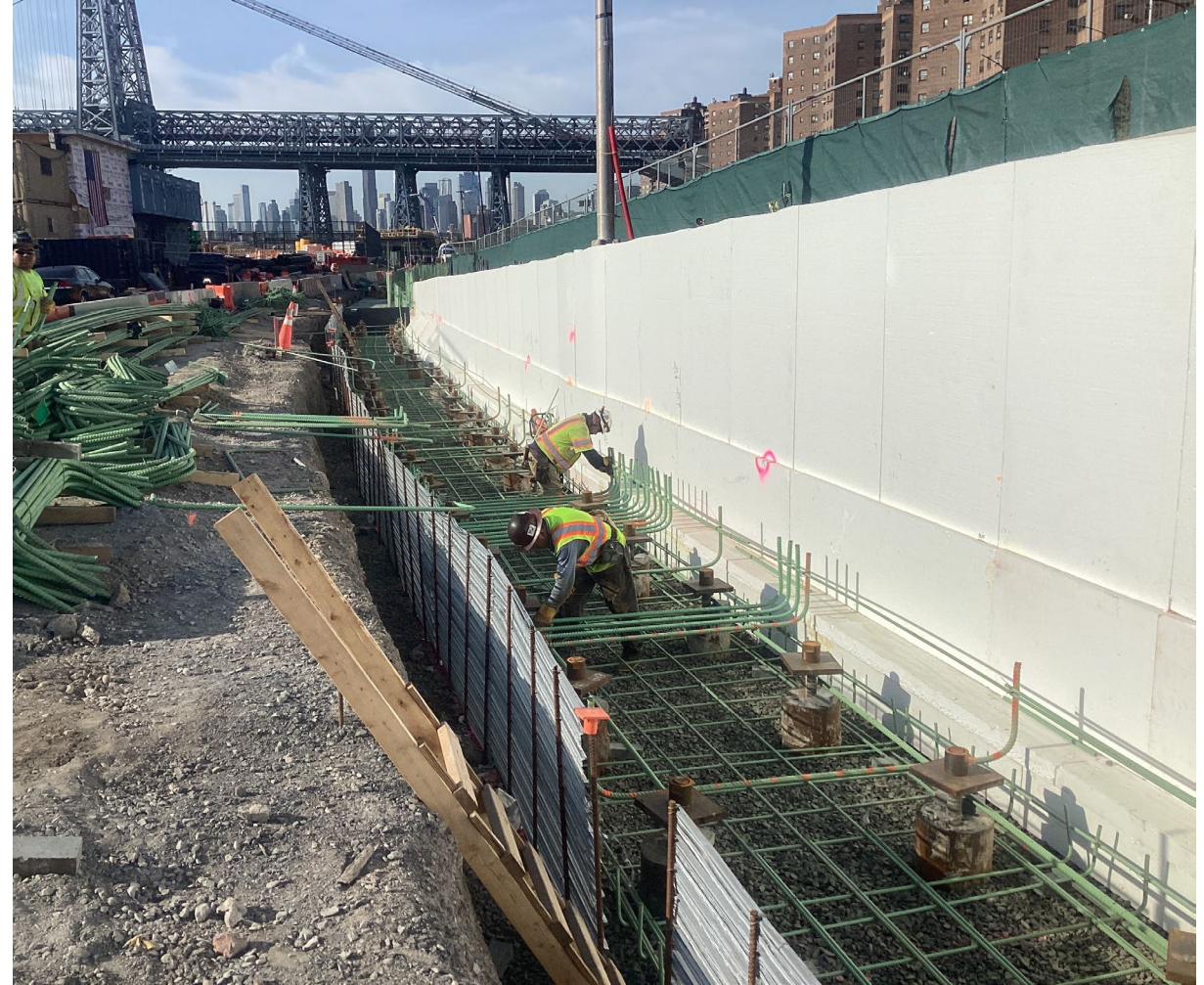
Installation of rebar for E. Houston St. retaining wall – April 2026
