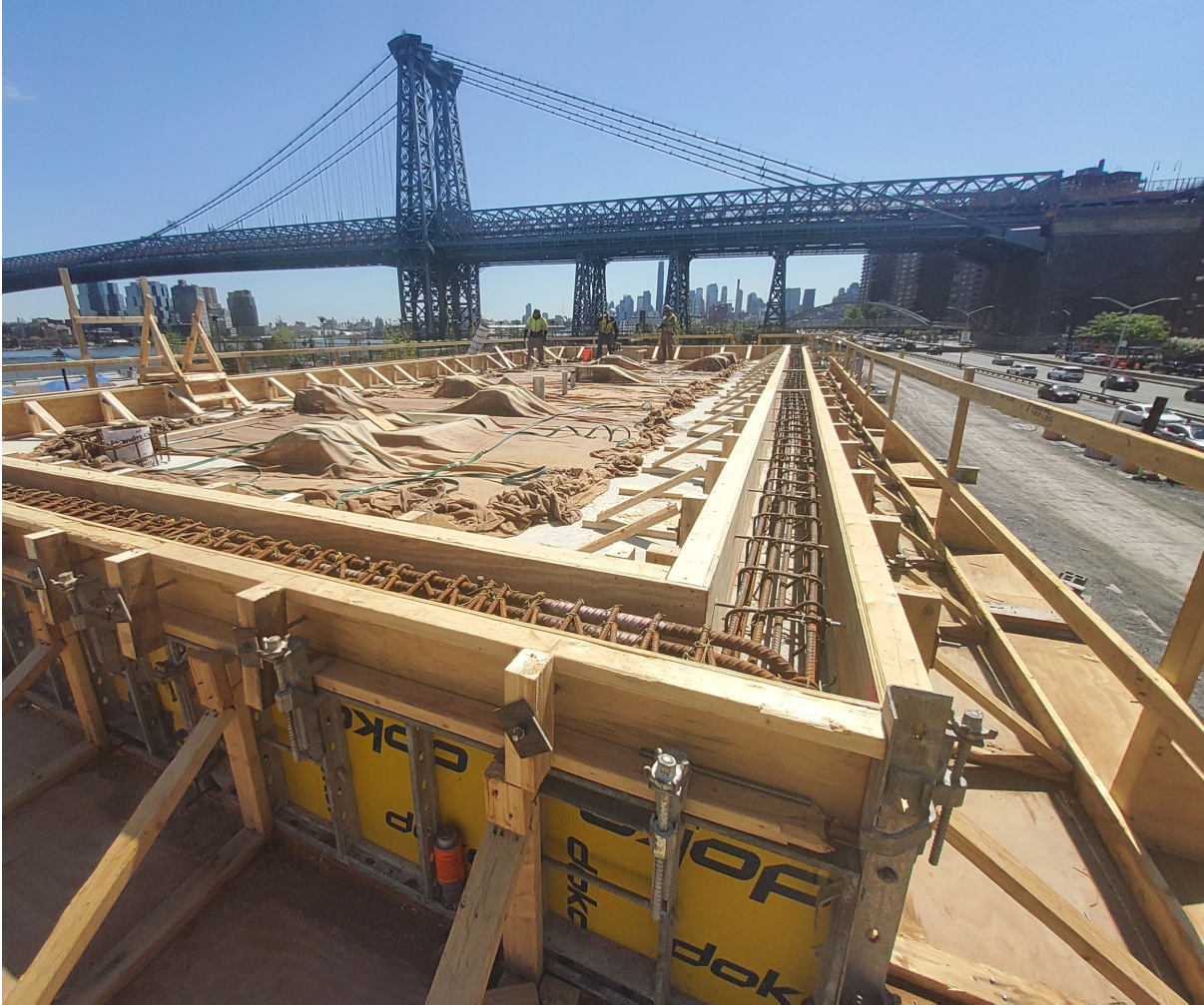
Formwork on rooftop of Tennis building – April 2026
