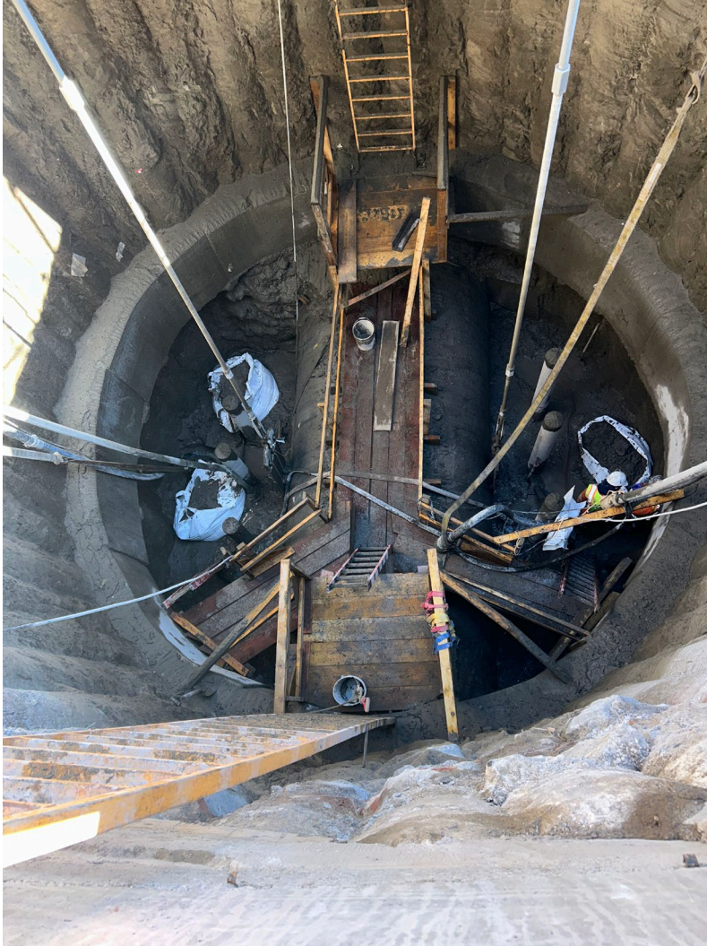
Deep drop manhole in Delancey St. North – April 2026
