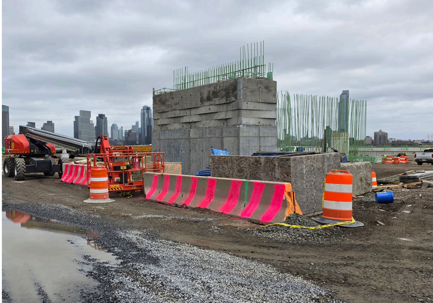
Eastern abutment for E. 10 th Street bridge – April 2026
