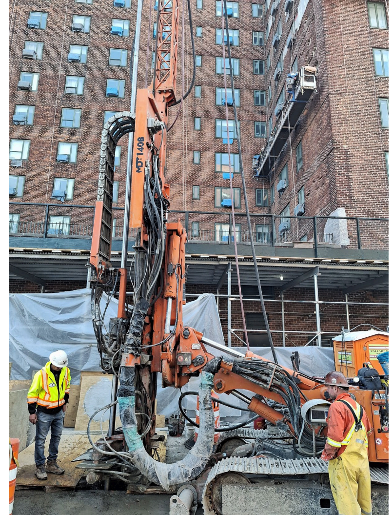
Jet grout column in E. 20 th Street – April 2026
