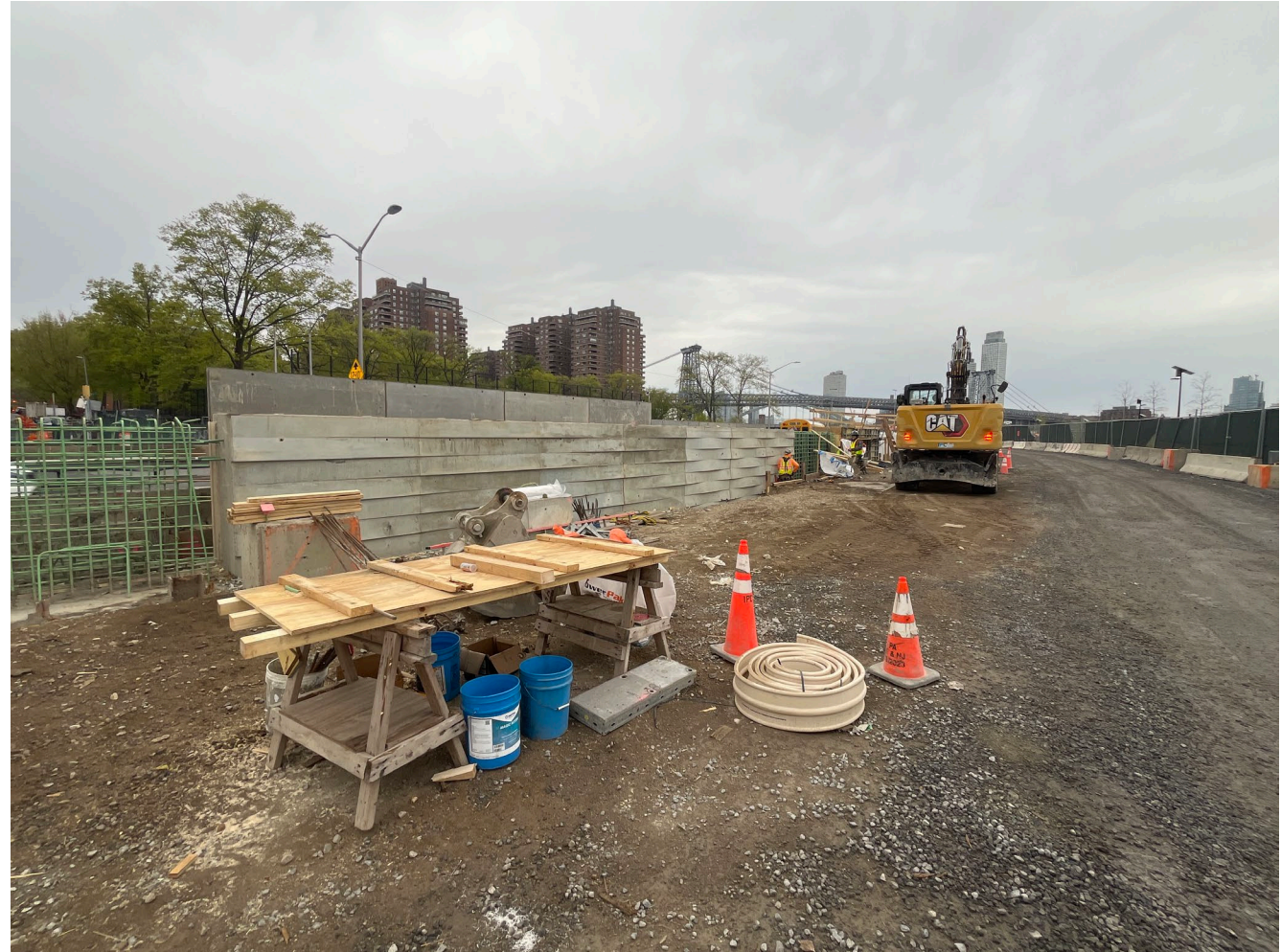
Floodwall concrete formwork removed adjacent to Pier 42 – April 2026
