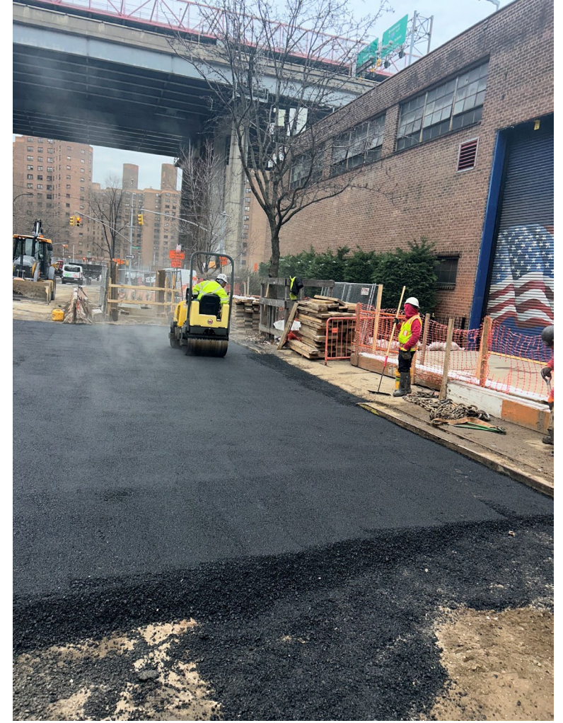
Backfilling sewer trench and installing temporary asphalt in Lewis Street – December 2025
