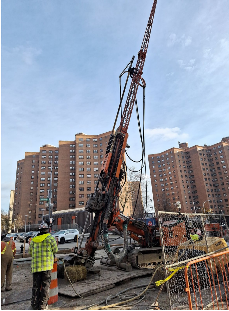
Jet grouting in Delancey St. North – December 2025
