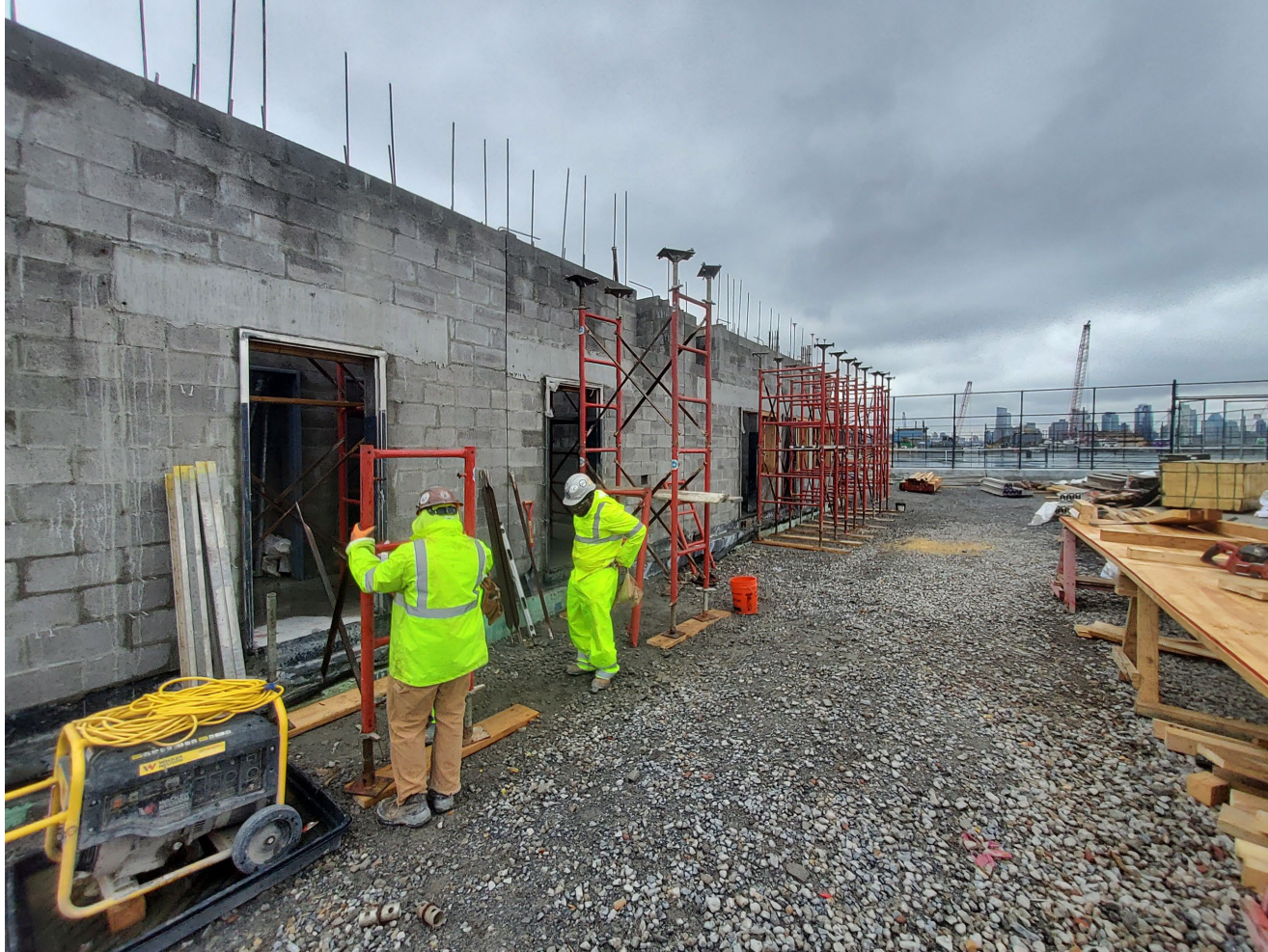
Scaffolding installed at tennis building site – March 2026
