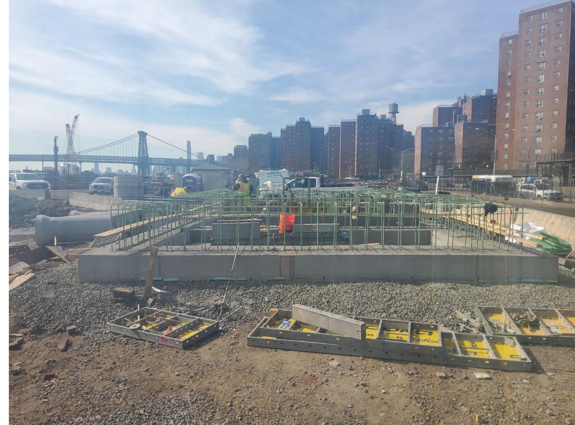
Rebar formwork for Parks maintenance building near Track – March 2026
