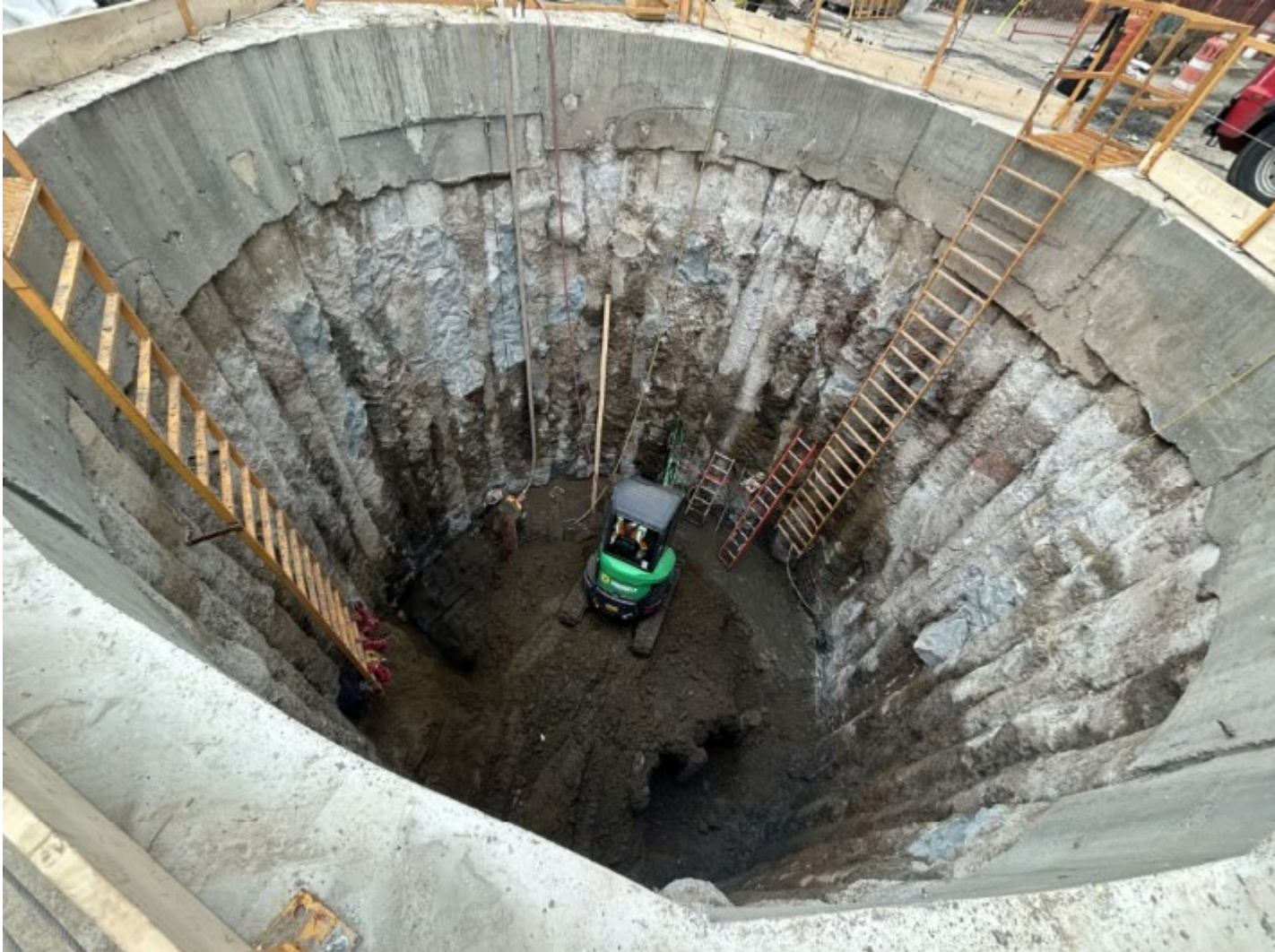
Excavation for deep drop manhole in Delancey St. North – March 2026
