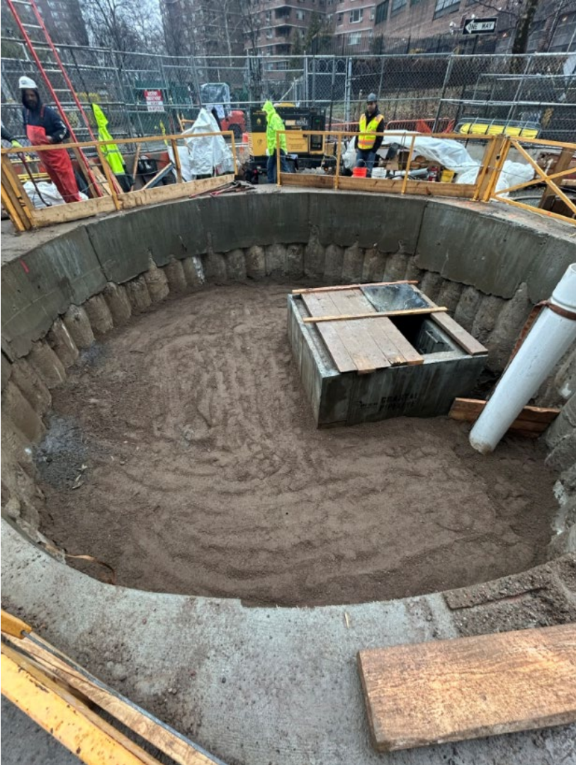
Backfilling deep drop manhole in Delancey St. South – March 2026
