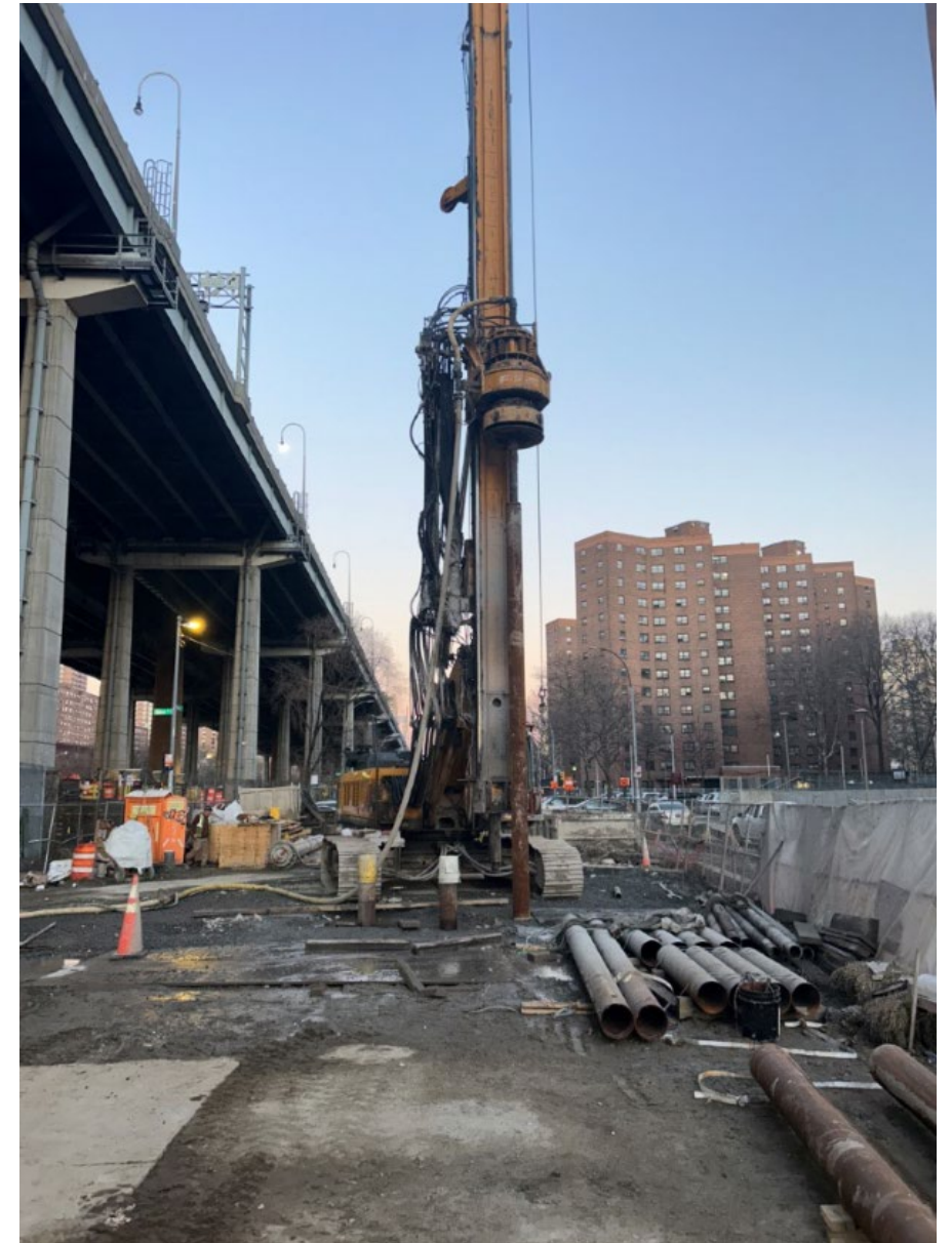
Caisson on rock pile installation on Delancey St. North – March 2026
