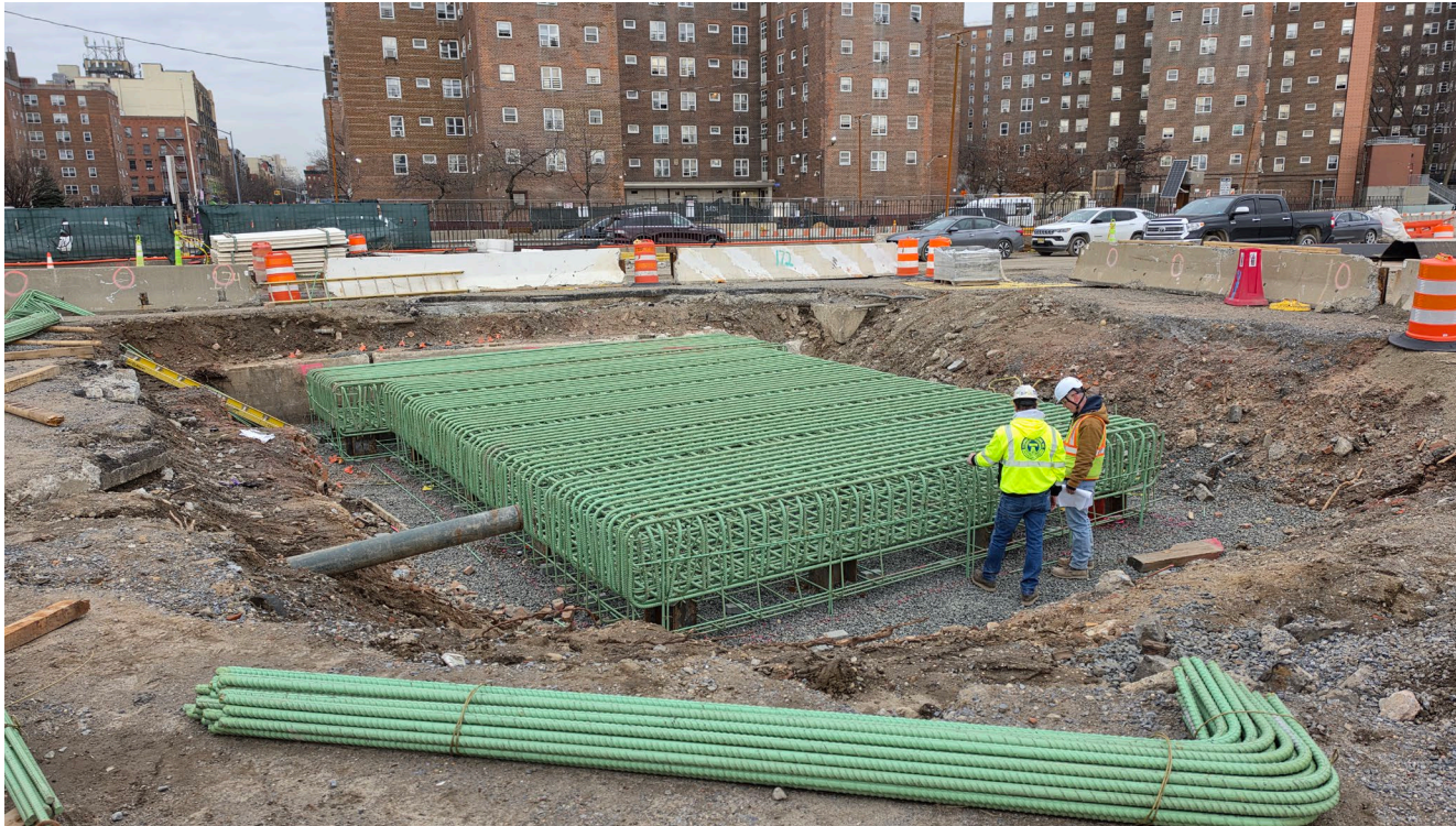
Rebar for E. 10 th Street bridge eastern abutment – March 2026
