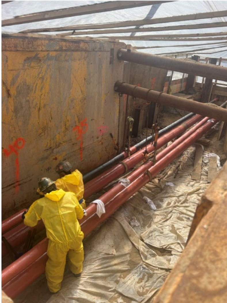
Utility work near Con Ed generation plant – March 2026
