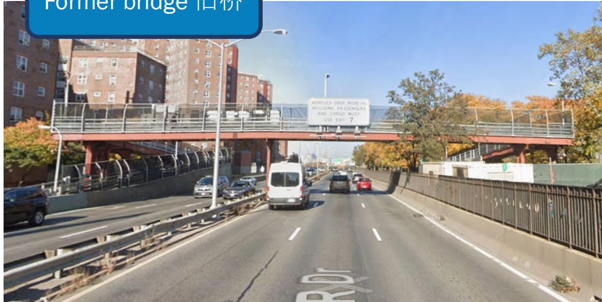
Former bridge 旧桥
