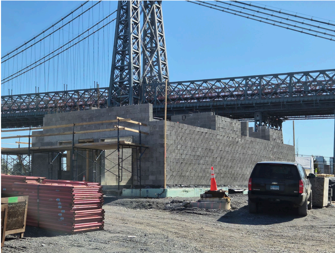
Tennis building construction – March 2026
