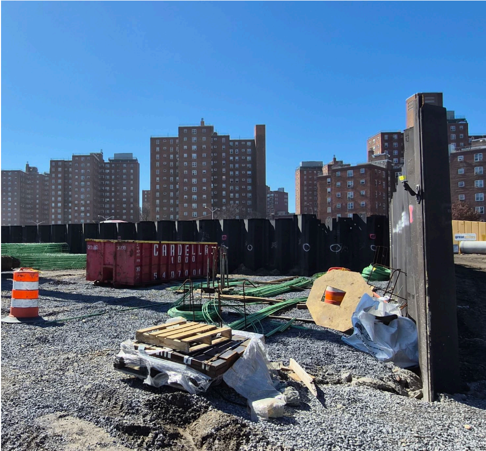
Buried floodwall near E. 10 th Street – March 2026
