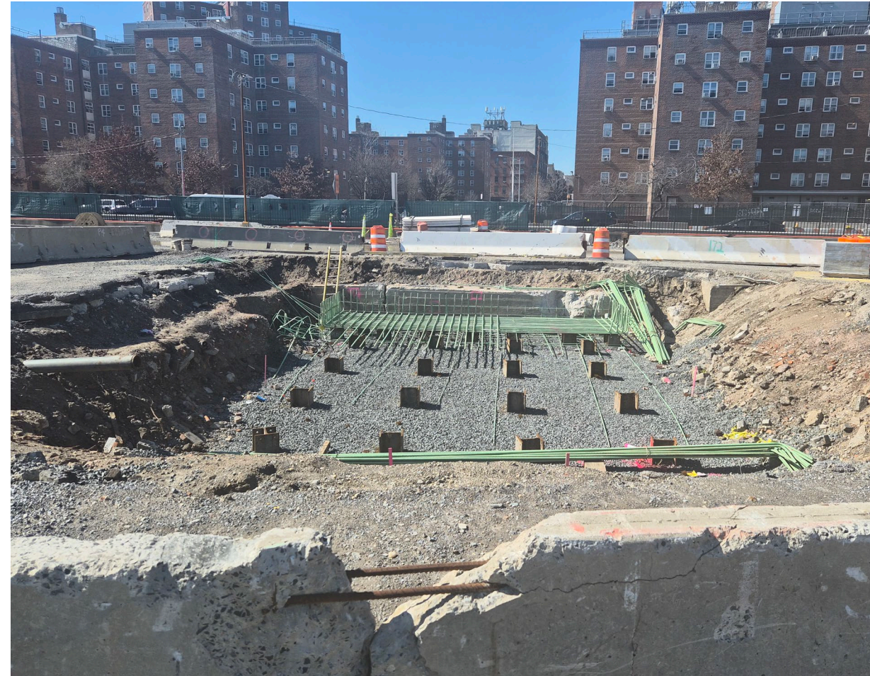
E. 10 th Street Bridge east abutment foundation - March 2026
