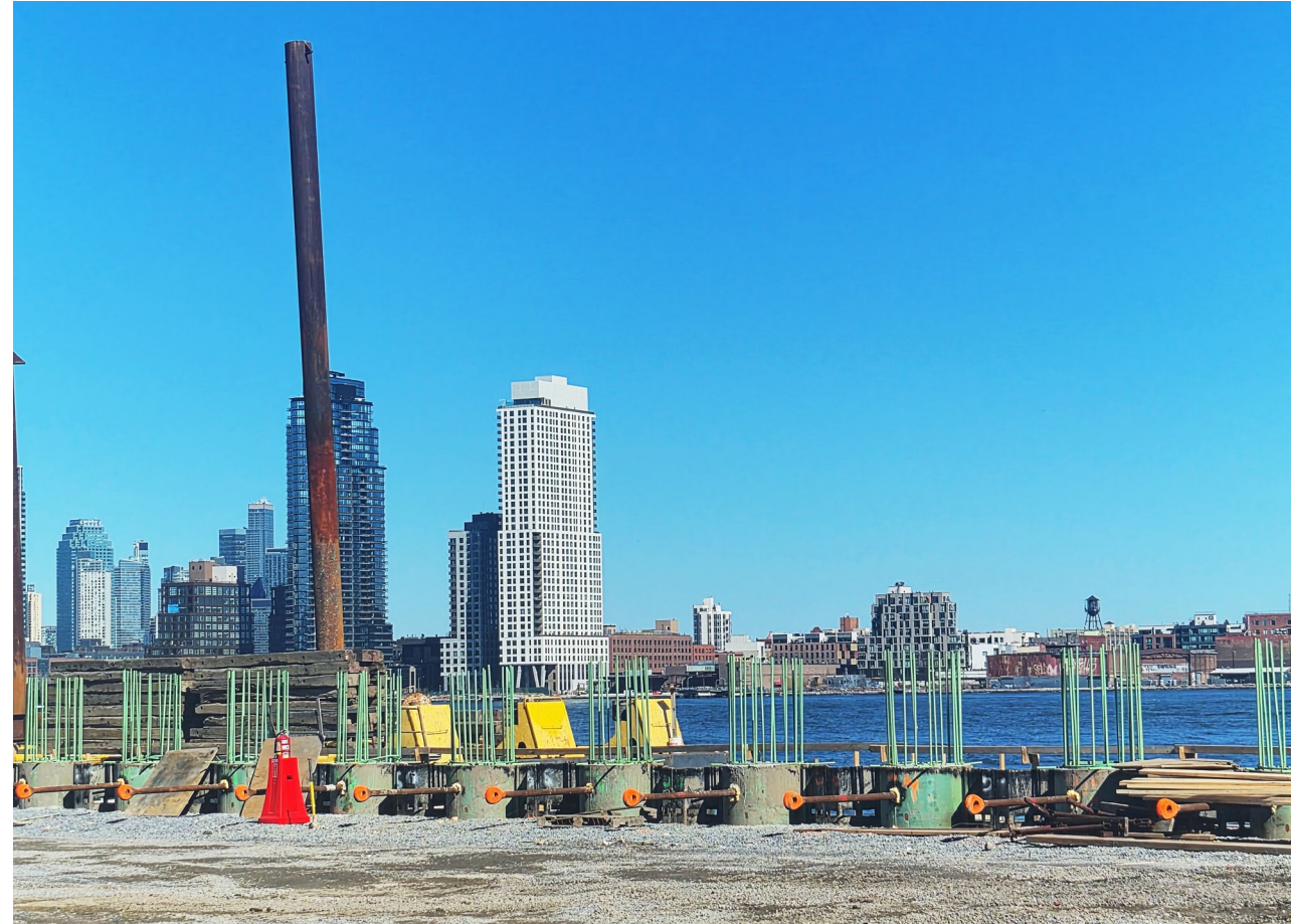
Combi-wall installation along waterfront in northern areas – March 2026
