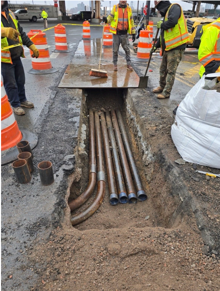
Installation of utility conduits on E. 20 th Street – March 2026
