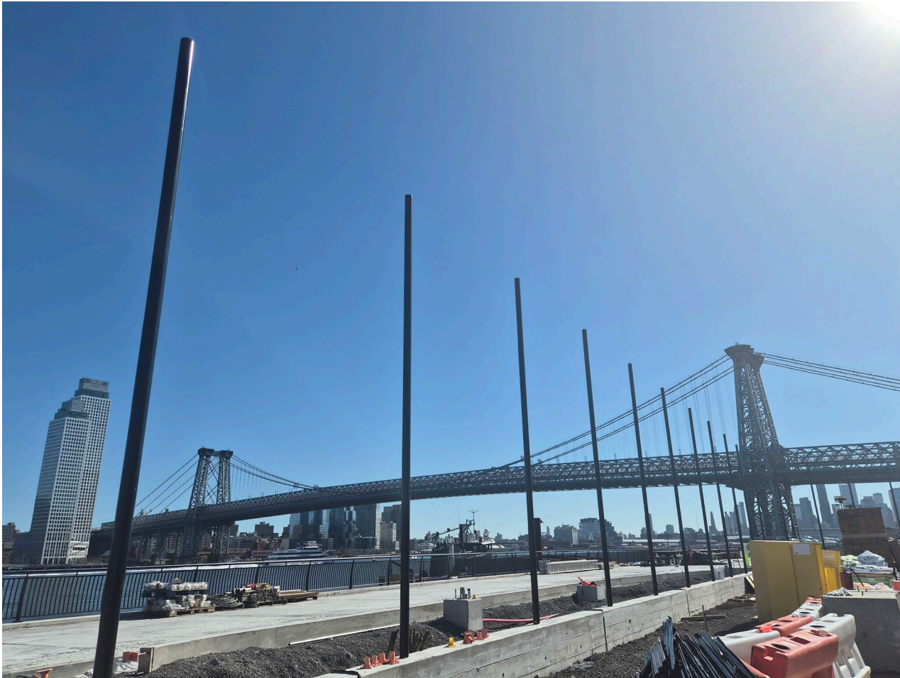
Fields 3 & 4 fence poles installed- March 2026
