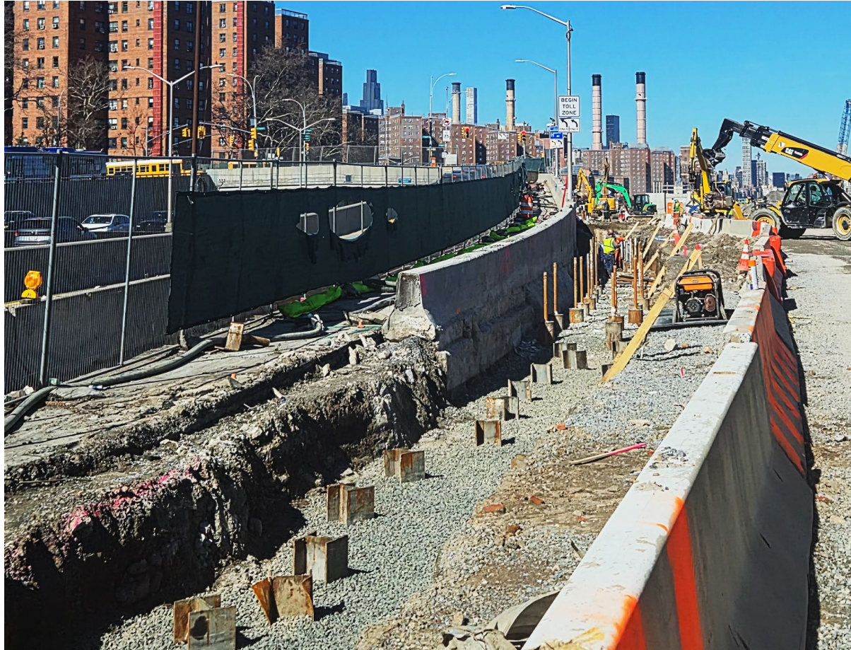
Micropile installation at E. Houston Street retaining wall – March 2026
