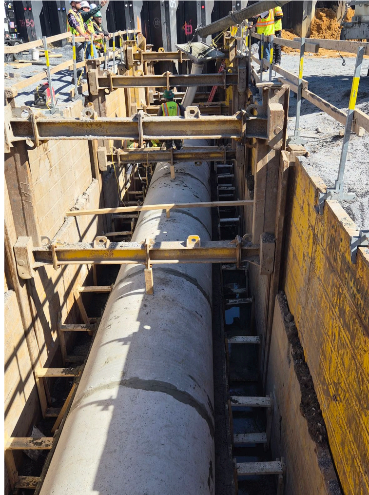
Sewer installation in Track area – March 2026
