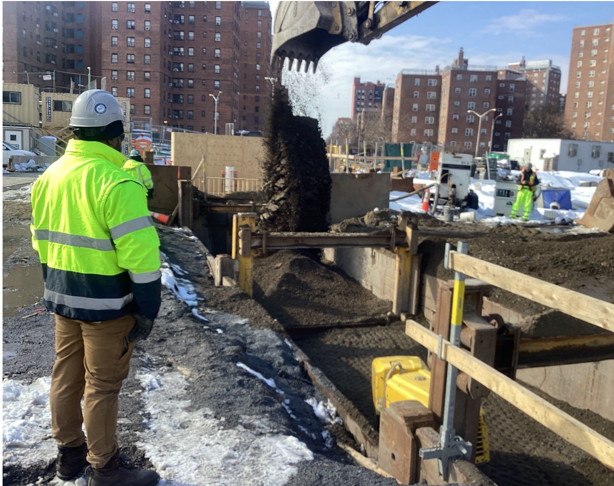
Backfilling sewer trench near Track area – February 2026
