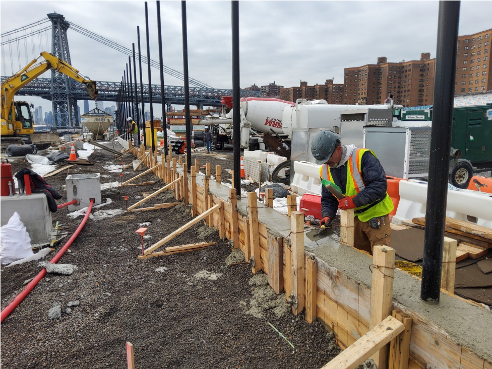
Installation of concrete curb for Fields 3 & 4 fence line – February 2026
