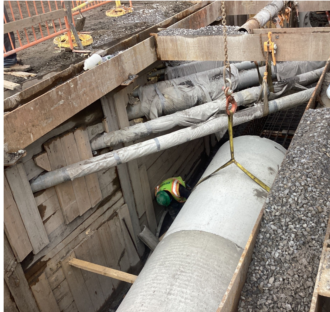
Sewer installation beneath existing utilities – February 2026
