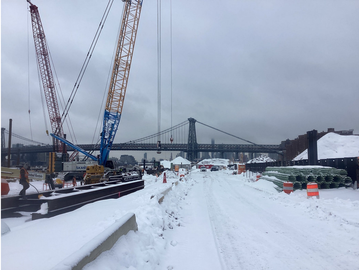
Snow on site north of Williamsburg Bridge – February 2026
