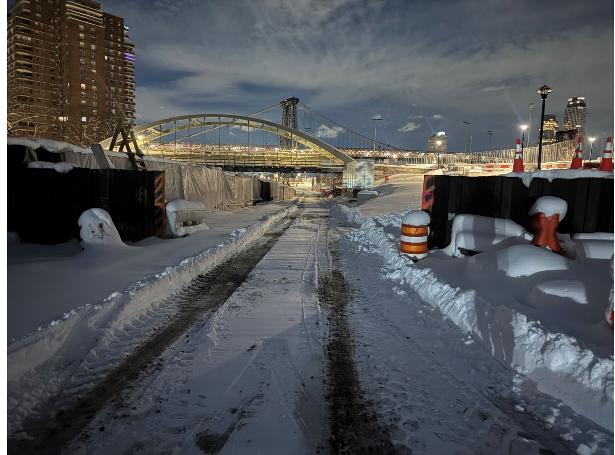
Snow removal along construction access road at Corlears Hook Bridge – February 2026
