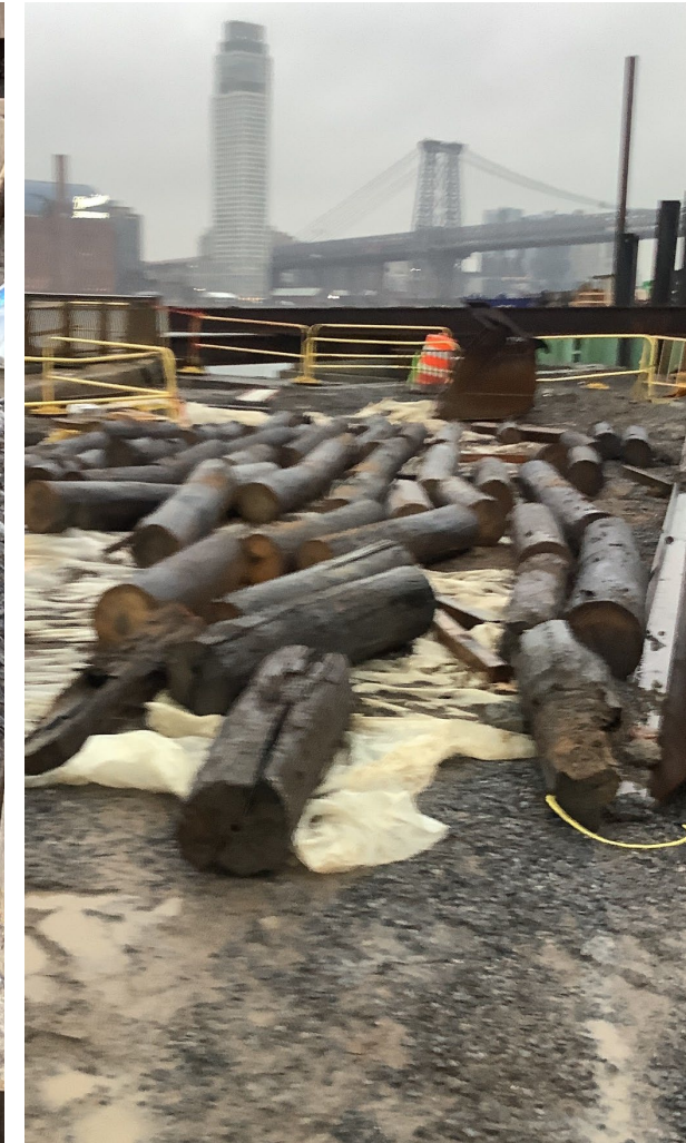
Removal of existing timber piles – February 2026
