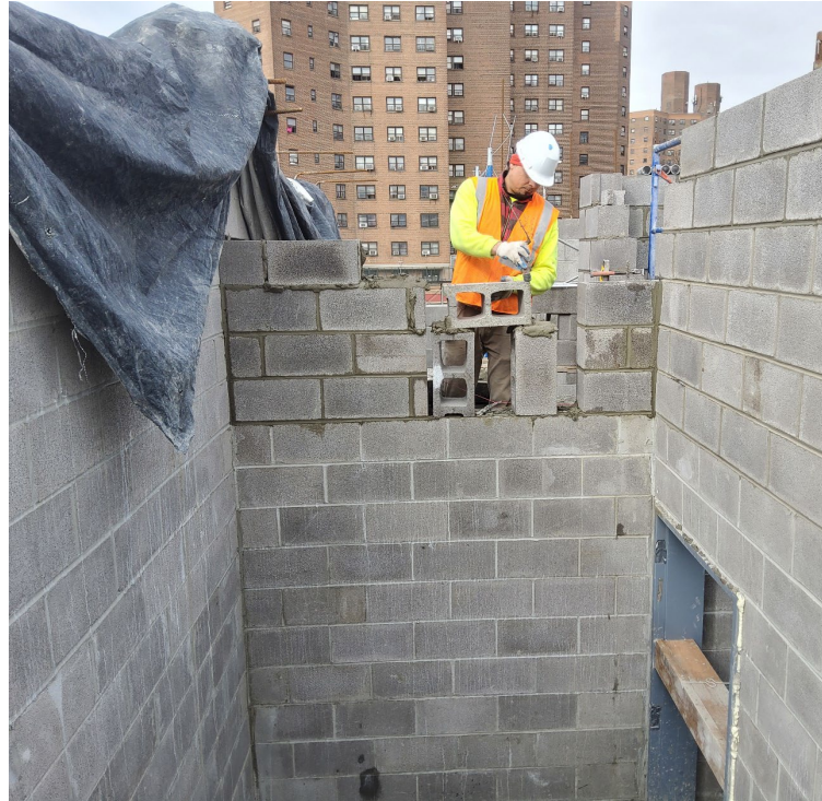
Masonry work at Tennis Building – February 2026
