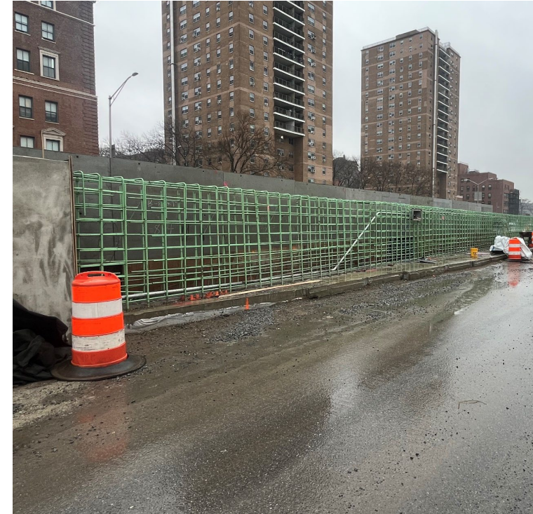
Rebar for floodwall along FDR Drive adjacent to Pier 42 – February 2026
