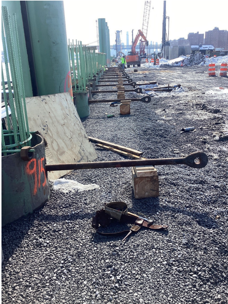
Tie-rod installation along waterfront – February 2026
