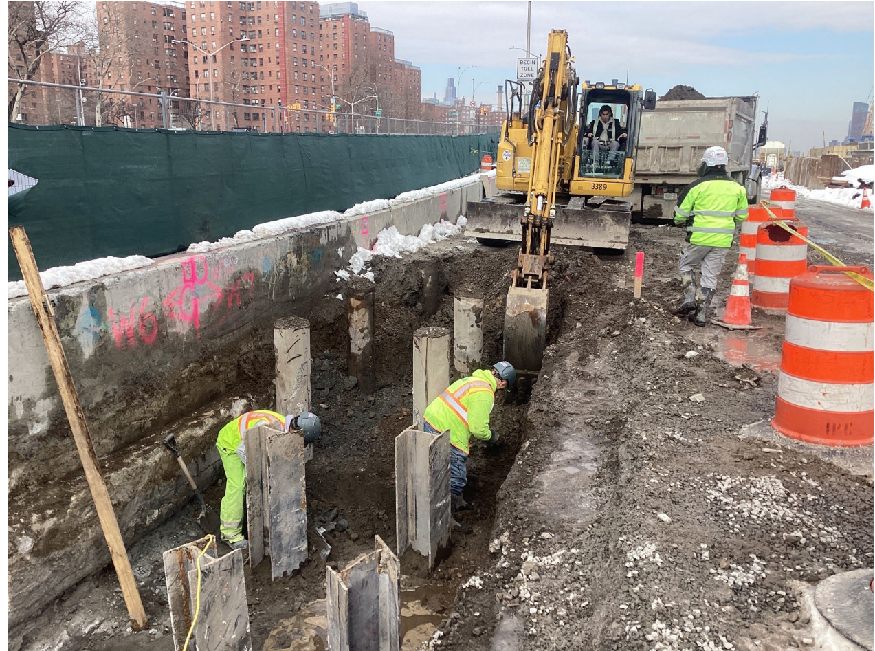
Excavation of E. Houston Street retaining wall footing – February 2026
