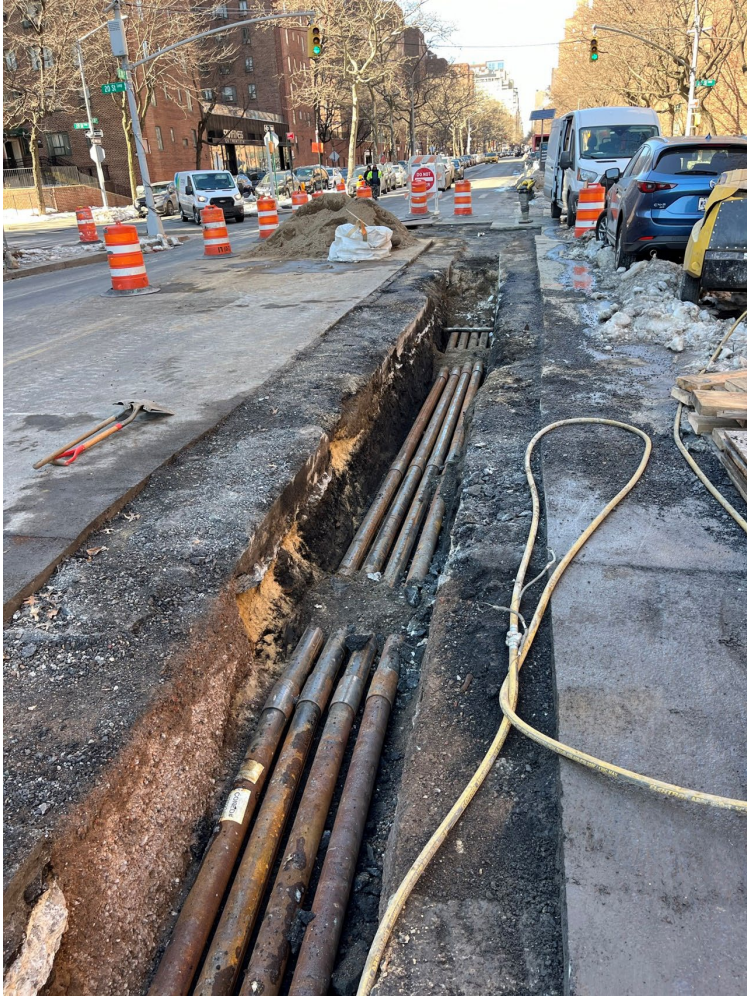
Con Ed conduit installation in E. 20 th Street – February 2026
