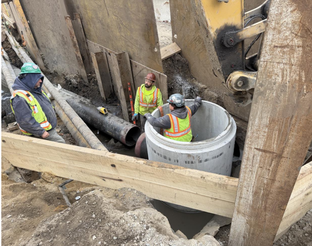
Manhole basin installed adjacent to FDR Drive and Riis Houses – January 2026
