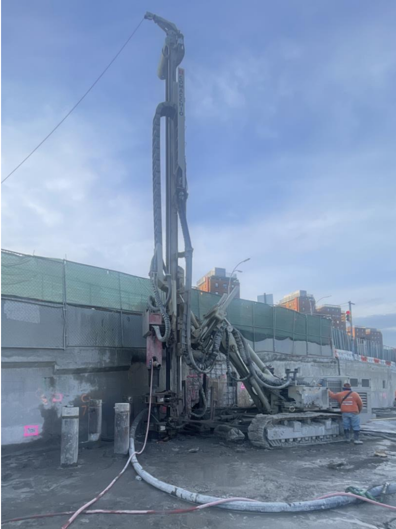
Micropile operation at E. Houston Street – January 2026
