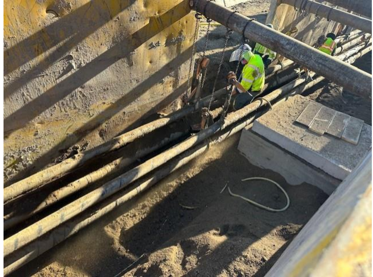
Hand-excavating around utility lines in vicinity of FDR Drive and Riis Houses – January 2026
