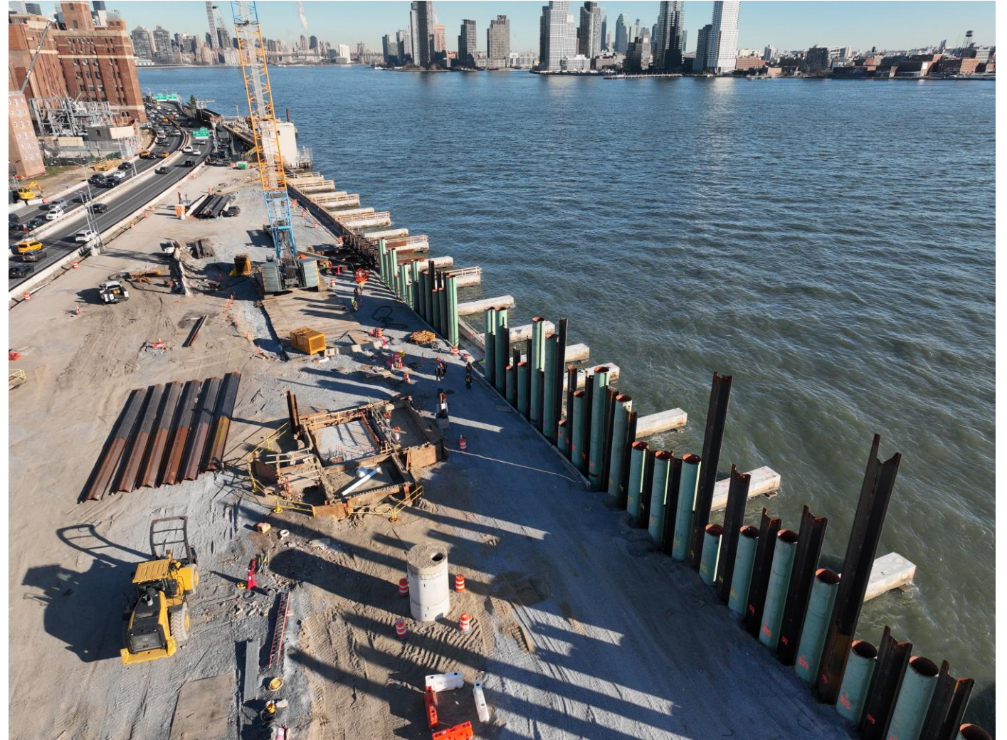
Combi-wall installation at north end of site – December 2025
