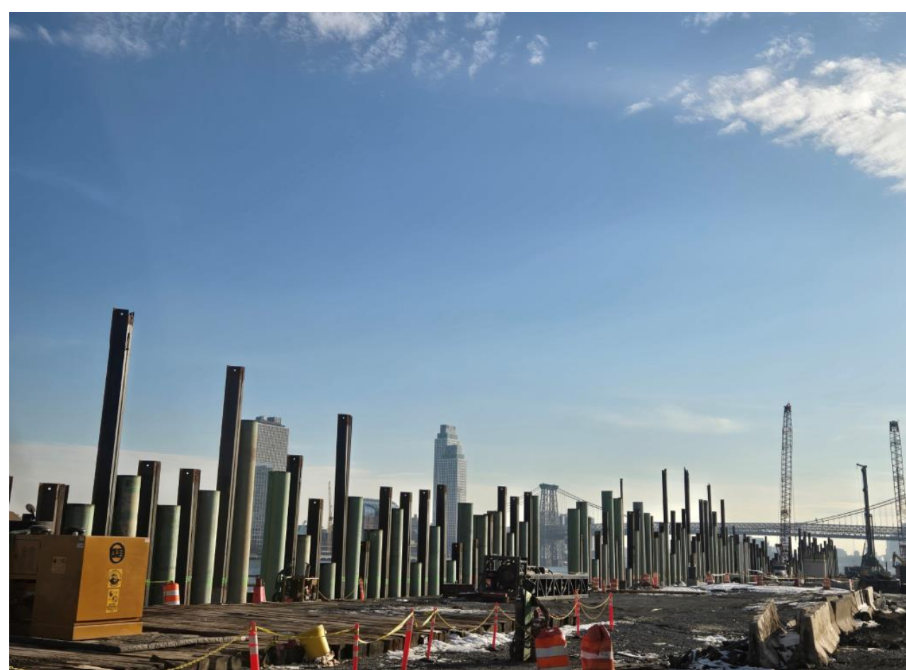
Combi-wall installation along East River waterfront – December 2025
