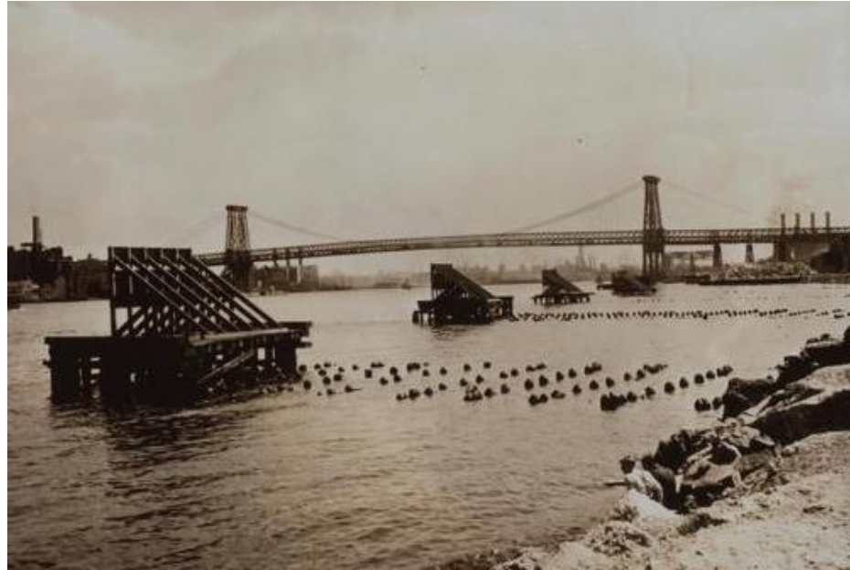
Bulkheads and pier stumps during demolition for East River Park and East River Drive – 1937
