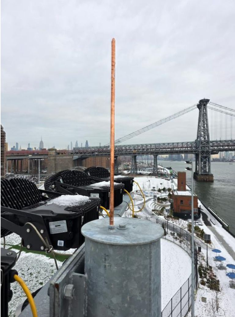
Lightning rod maintenance on Fields 1 & 2 sports light towers – December 2025
