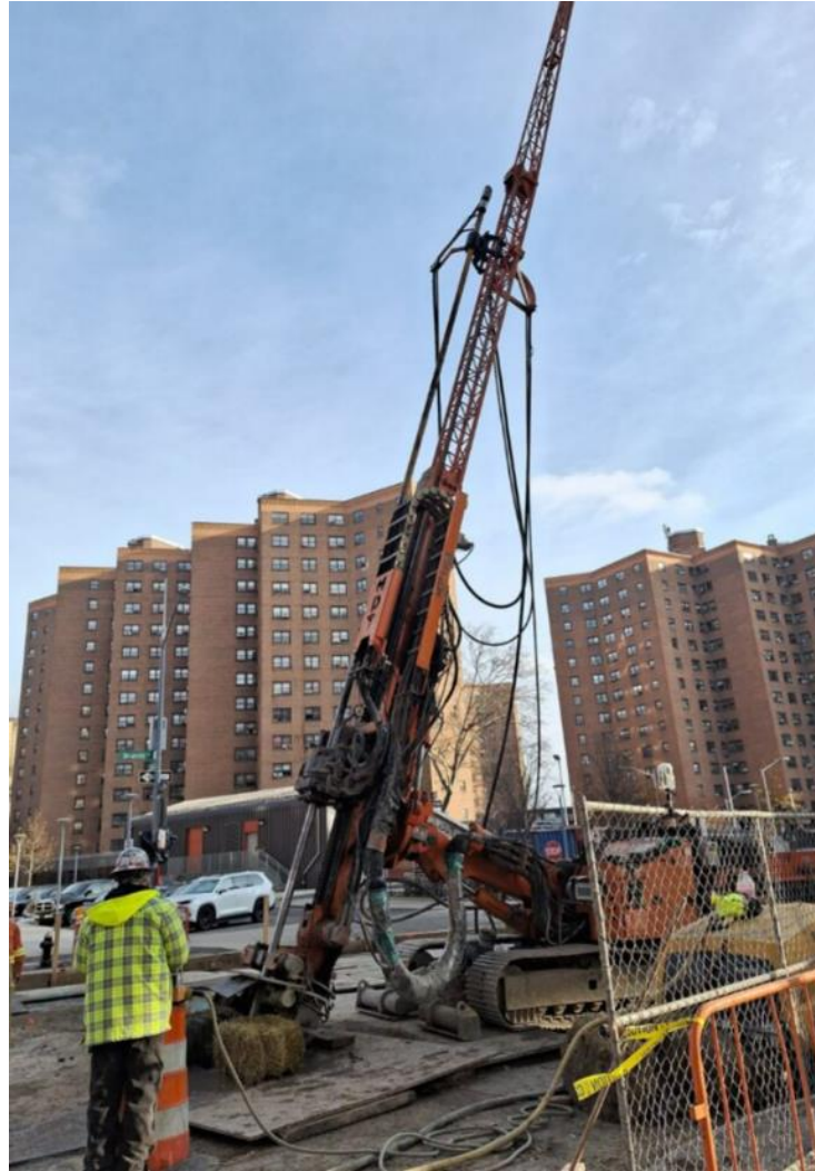
Jet grouting on Delancey St. N – December 2025
