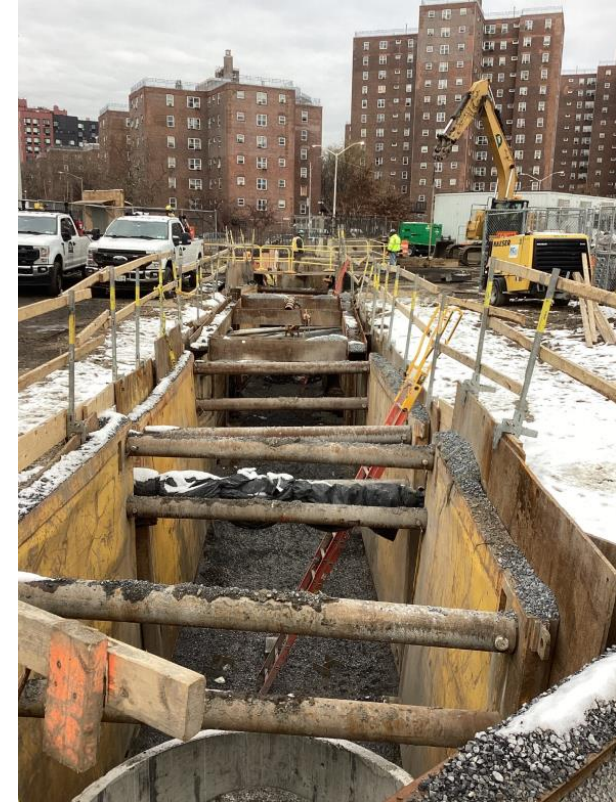
Trench for sewer construction near Track site – December 2025
