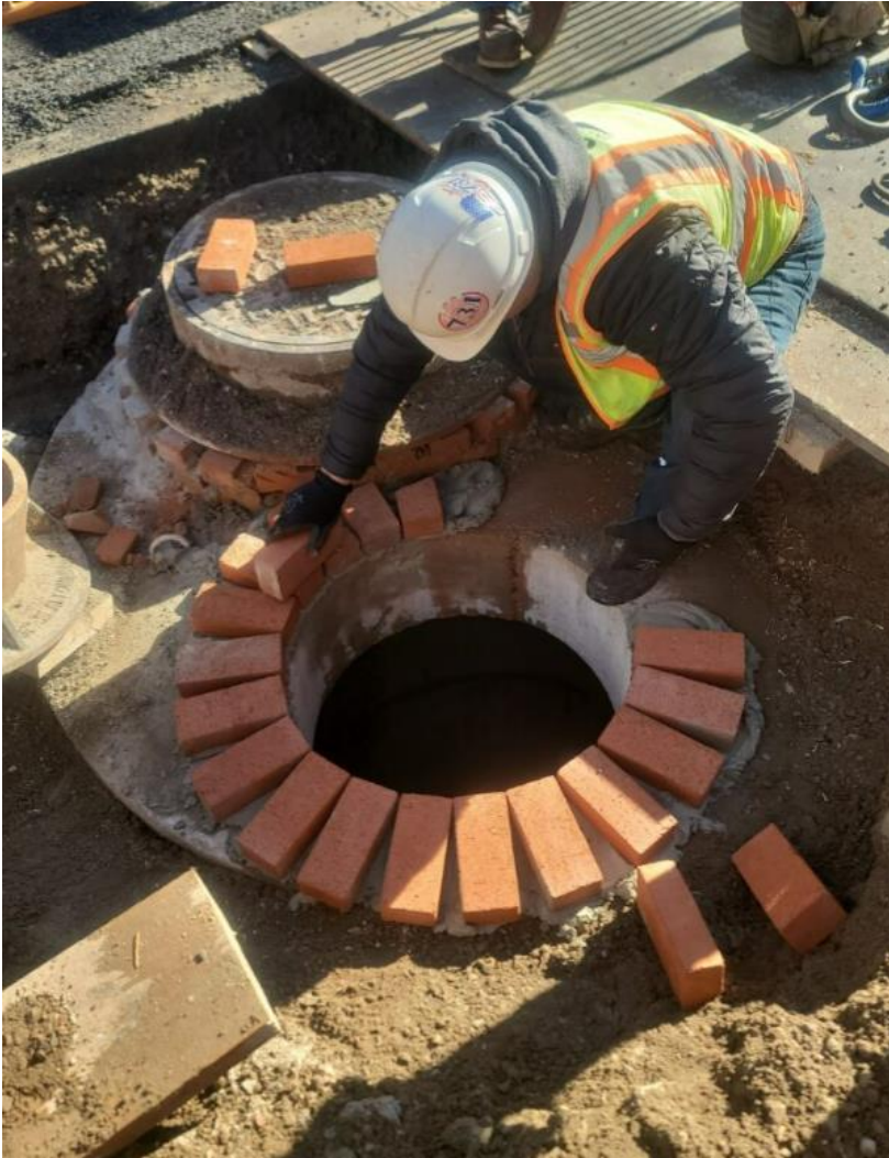
Installing frame and casting for manhole at Broome and Lewis St. – December 2025
