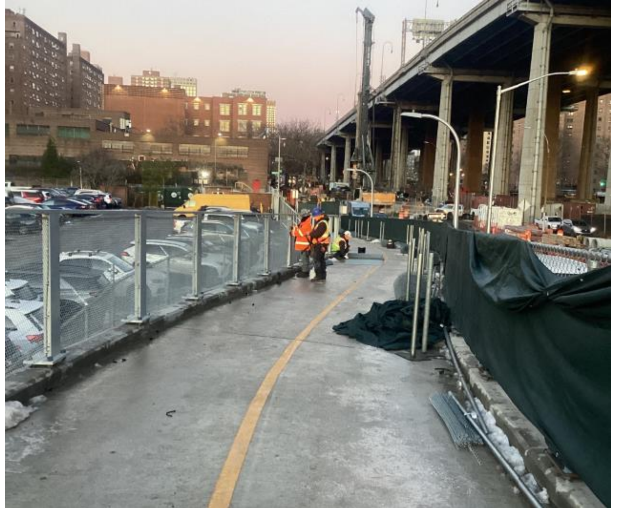
Installing rails on Delancey Street bridge – December 2025
