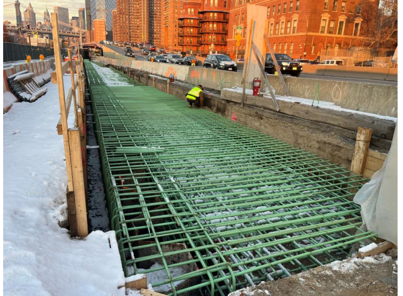
Rebar for floodwall footing near Pier 42 – December 2025
