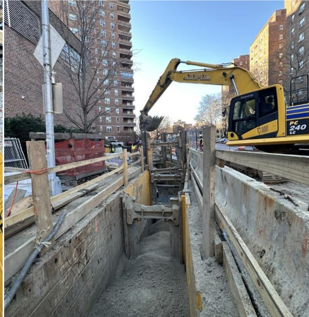
Backfilling sewer trench on Lewis St. – December 2025
