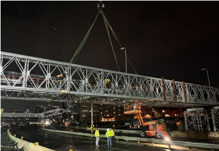
Removing overhead signage (top), bridge rigged with straps (bottom) – November 2025
