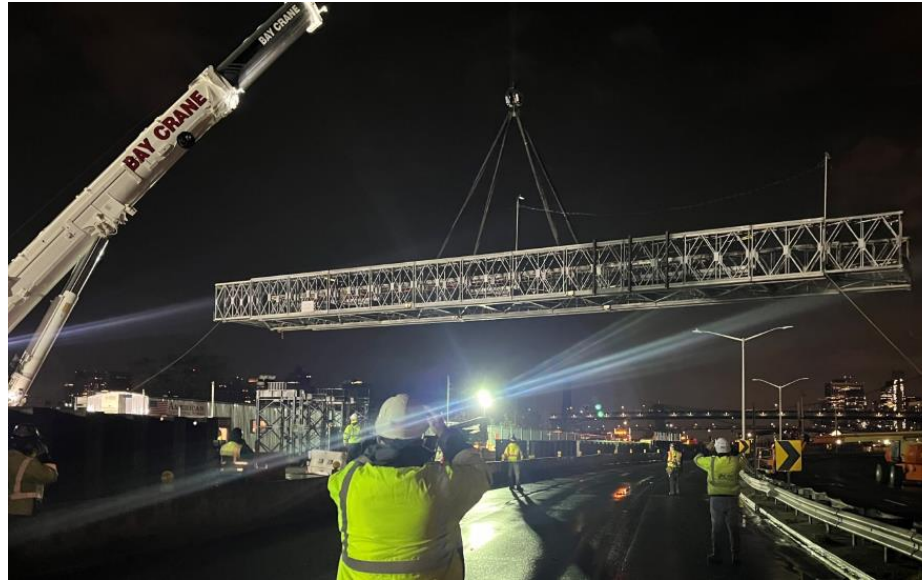
Temporary bridge span lifted by crane – November 2025
