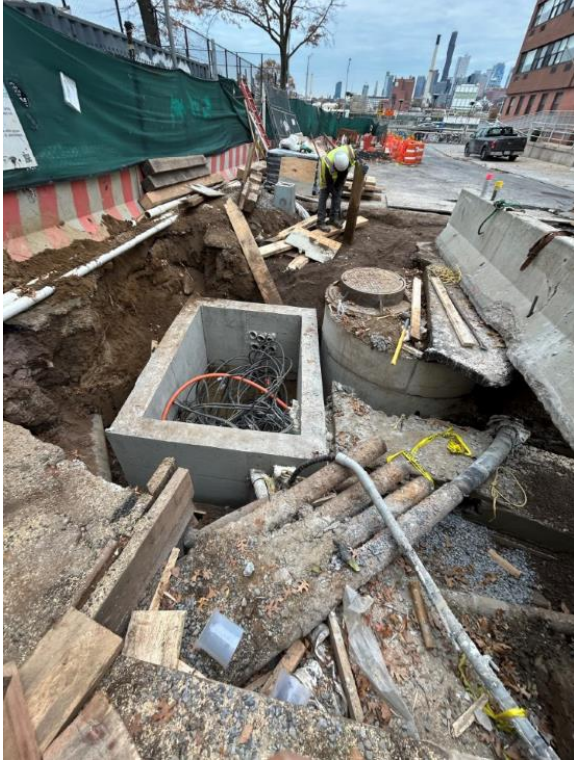
Manhole construction at Jackson St. and Water St. – November 2025
