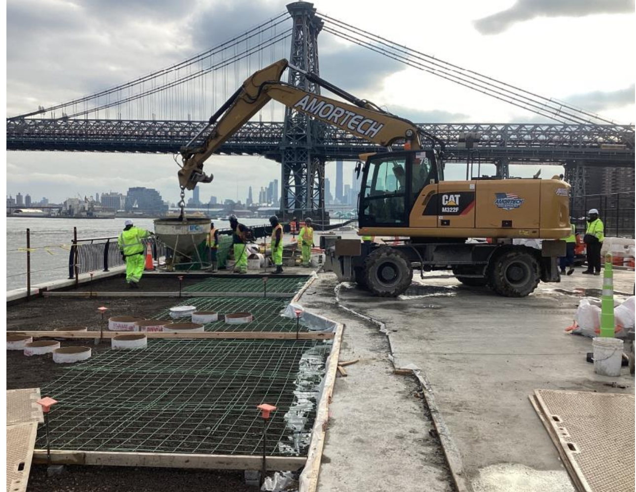
Concrete placement for esplanade north of Tennis Courts – November 2025
