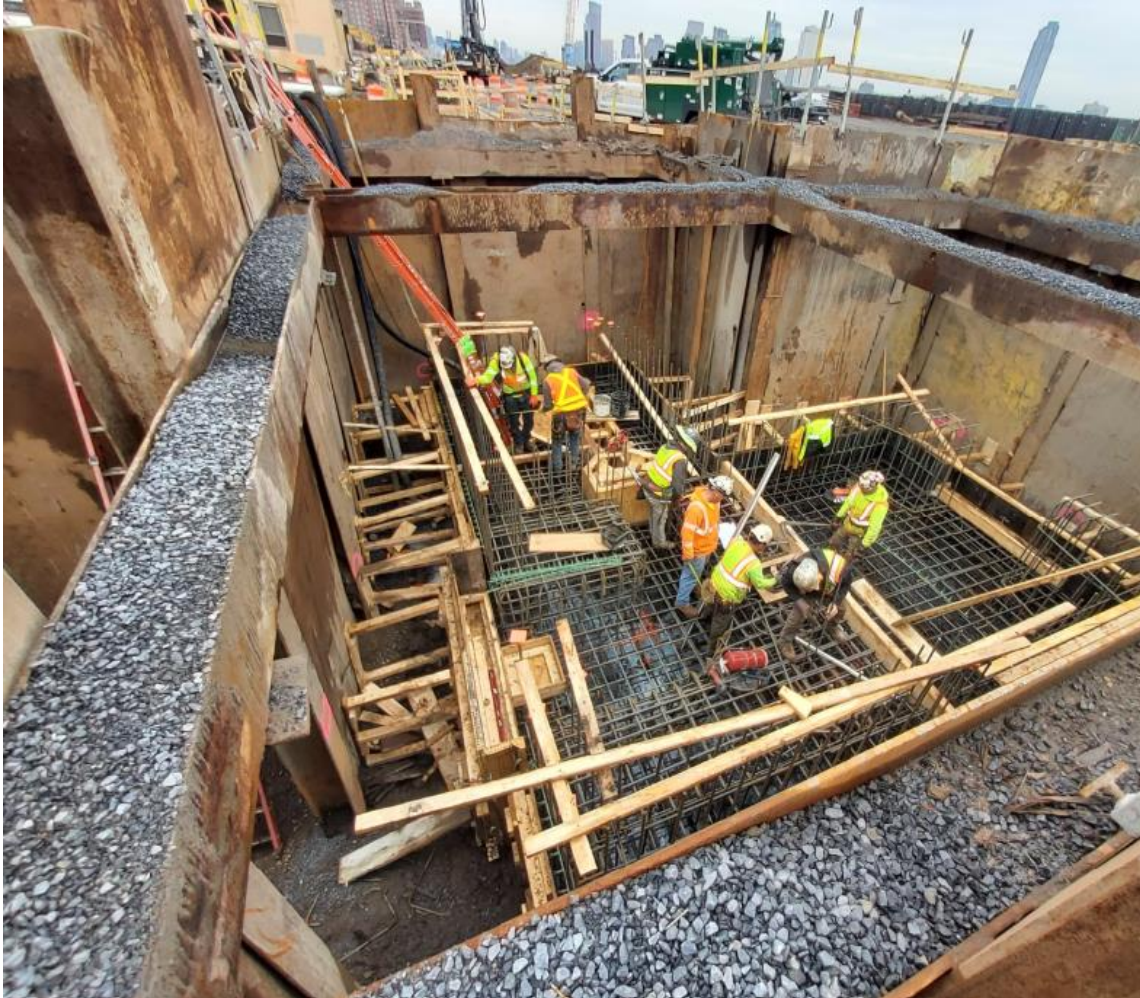
Regulator chamber construction near Track area – November 2025
