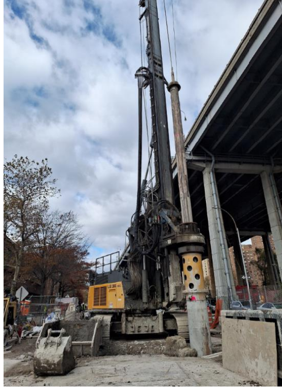
Secant pile installation at Delancey St. S and Baruch – November 2025
