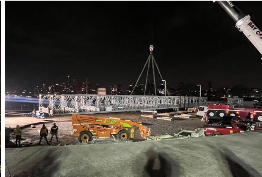
Temporary bridge span placed in construction area south of Amphitheater – November 2025
