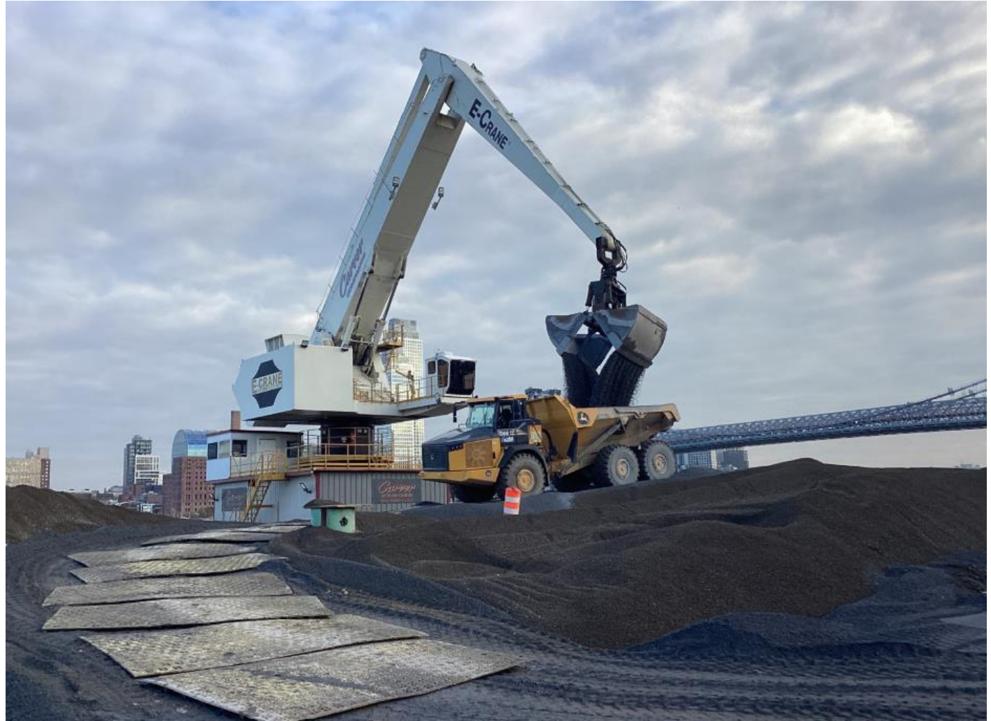
Clean fill unloaded from barge via crane – November 2025
