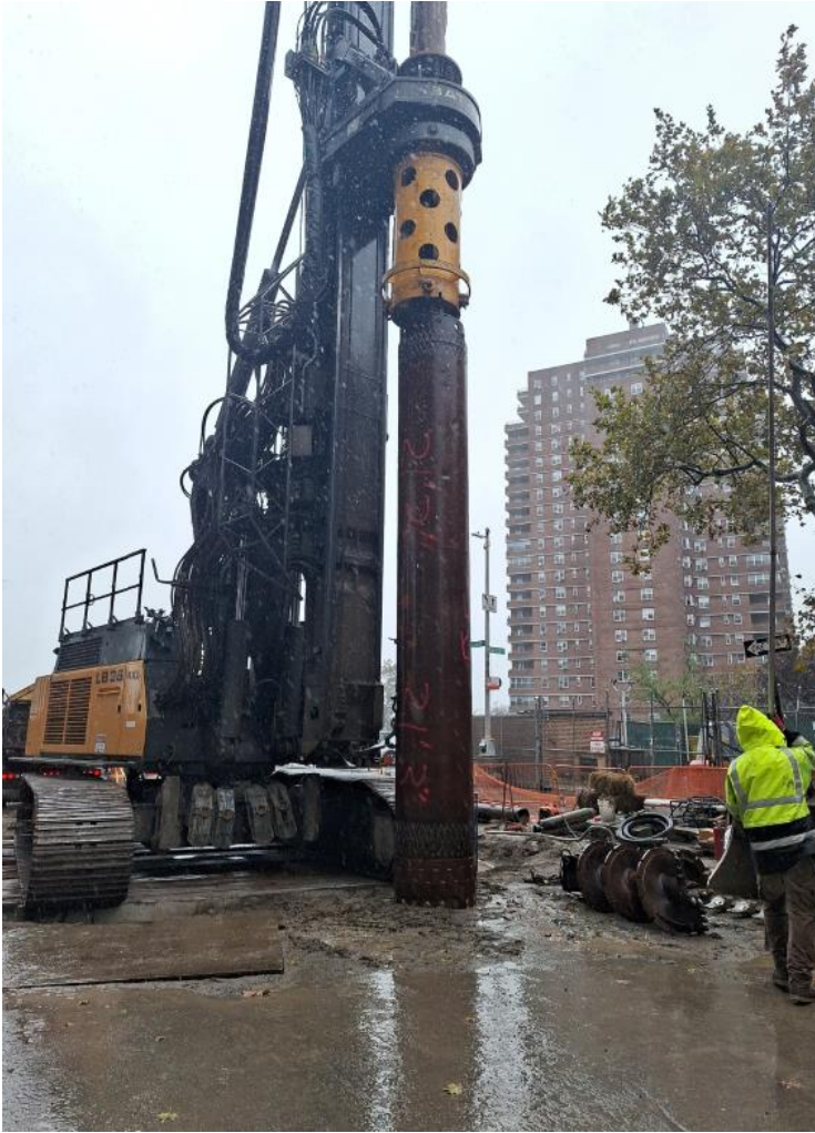
Secant pile installation at Delancey St. S and Baruch Drive – November 2025
