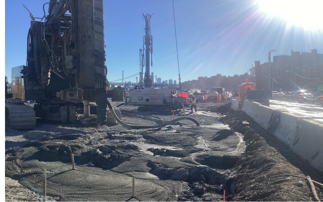
Earthwork and soil stabilization – November 2025
