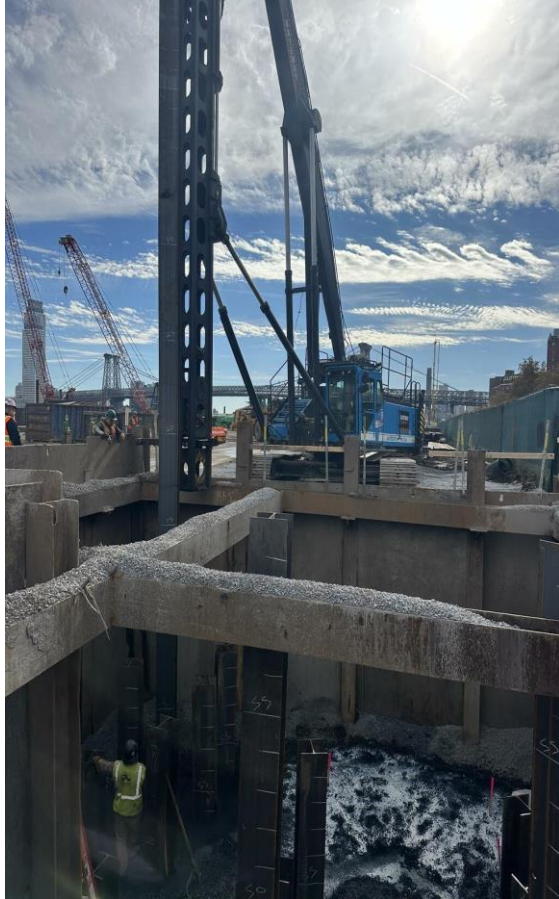
Installation of h-piles for sewer foundations – November 2025
