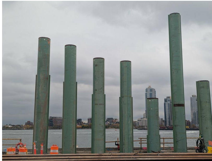
Installation of pipe piles for combi-wall – November 2025
