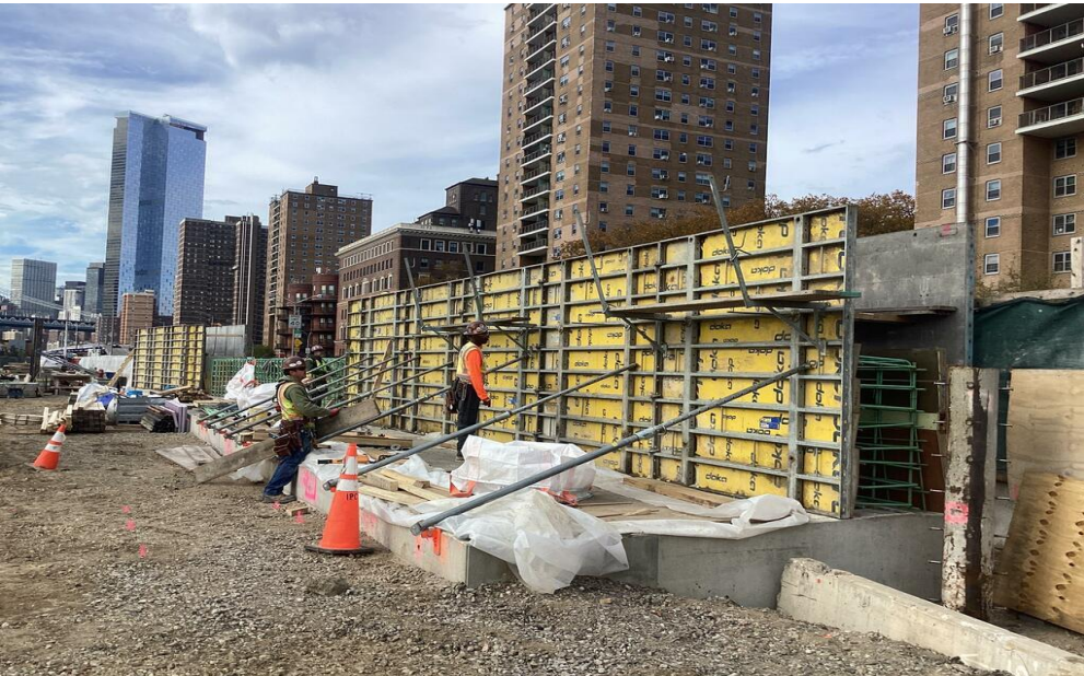
Southern floodwall formwork – November 2025
