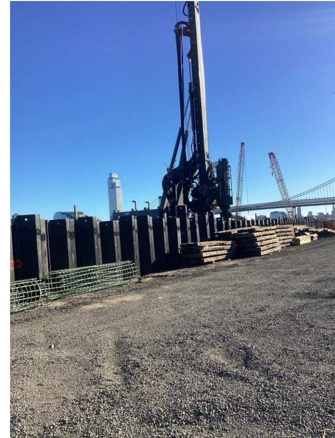
Installation of sheets for buried floodwall – November 2025
