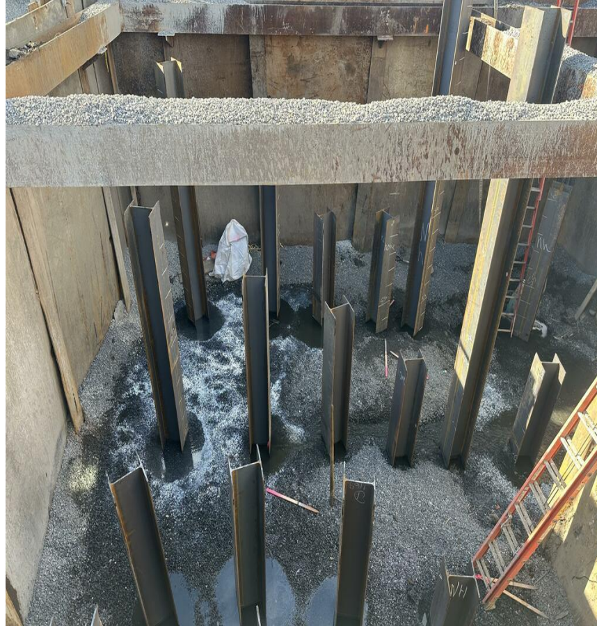
Installation of h-piles for sewer foundations – November 2025
