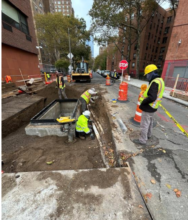
Utility relocation and manhole construction at Water St. and Jackson St. – November 2025
