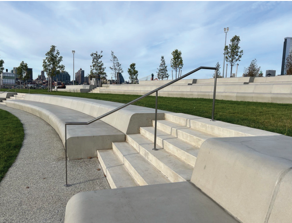
EAST RIVER PARK AMPHITHEATER- CONCRETE
