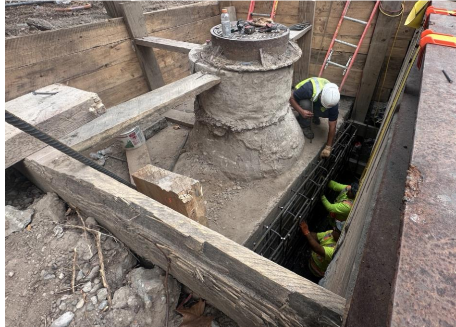
Manhole modification at Columbia St. and E. Houston St. – September 2025
