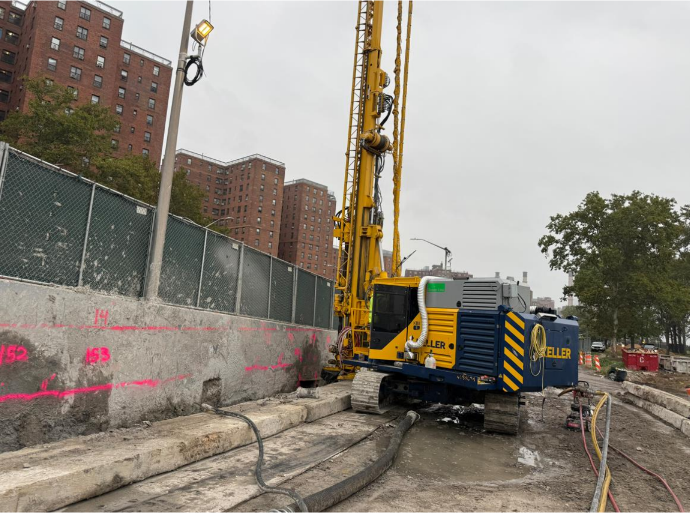
Jet grouting operations at E. Houston Street retaining wall – September 2025
