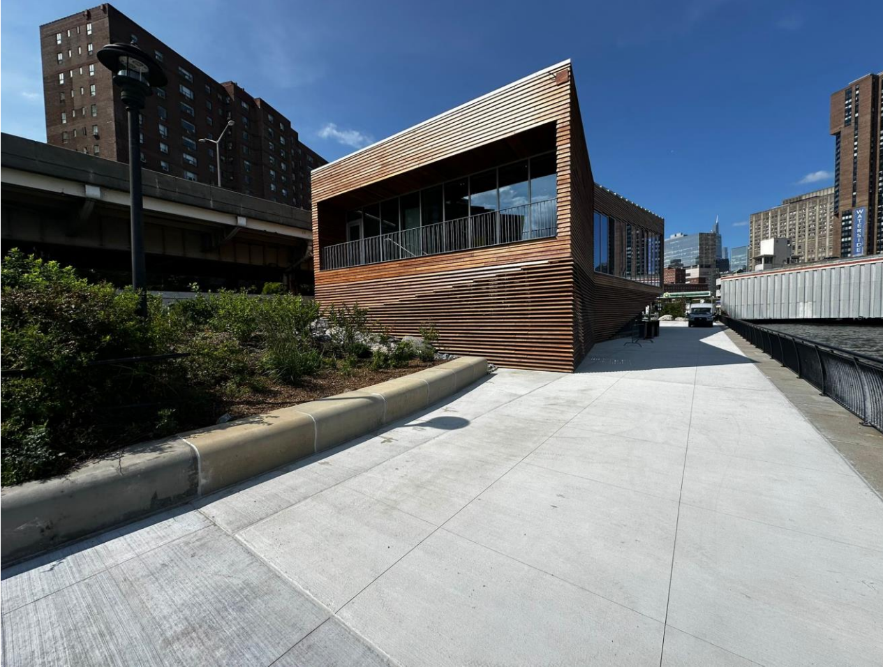
Completed Solar One building (separate from ESCR) – September 2025
