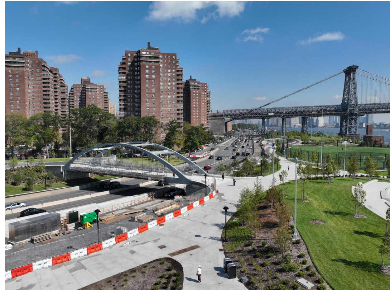
Park access via Corlears Hook bridge – September 2025
