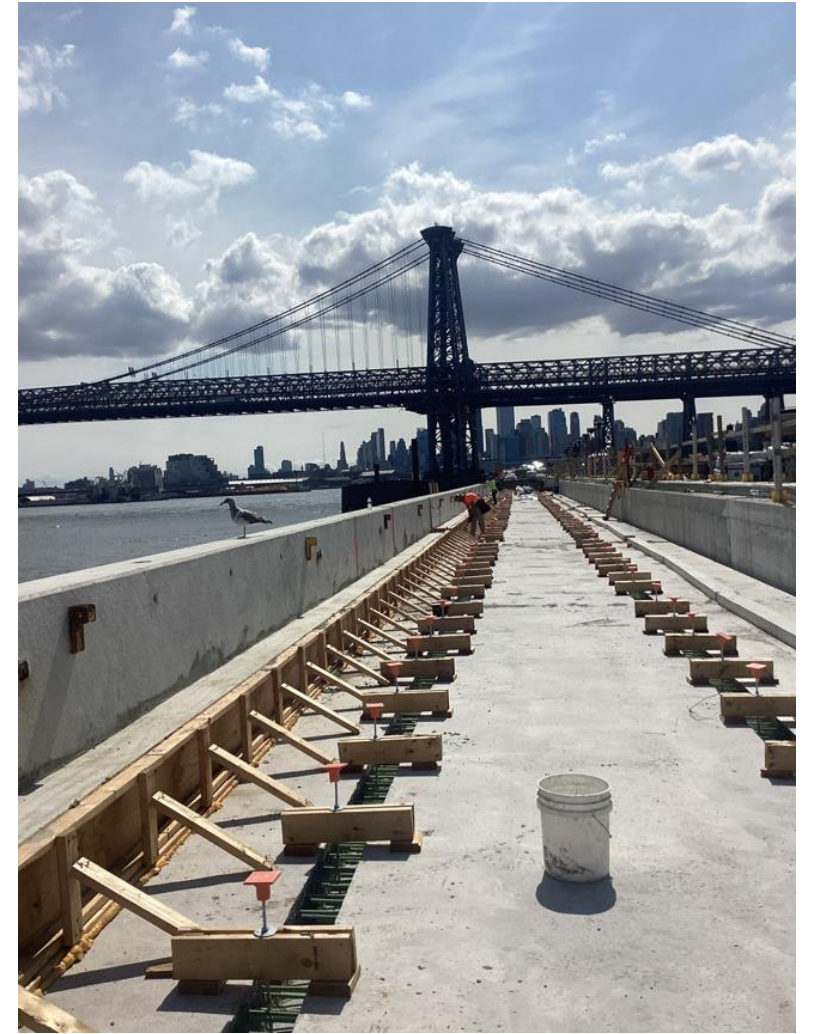
Concrete formwork removed from new esplanade sections north of Williamsburg Bridge – September 2025
