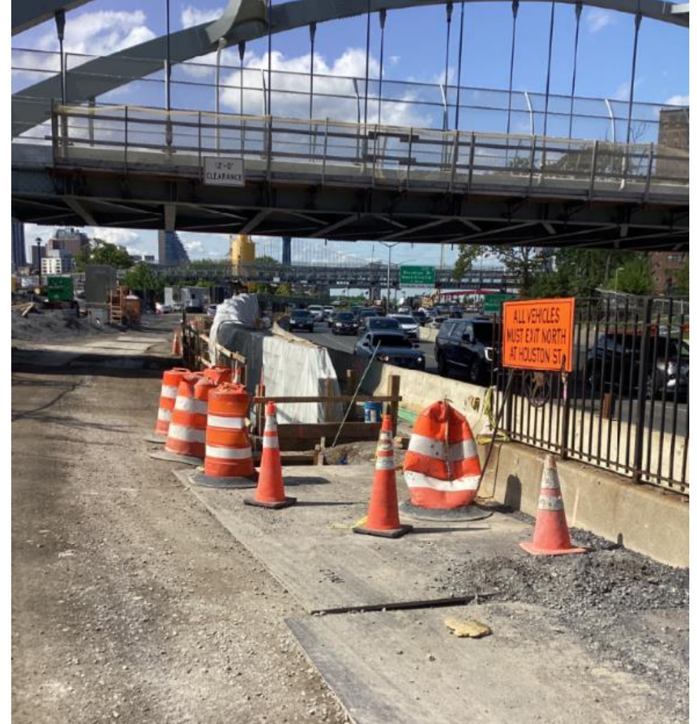
Floodwall construction under Corlears Hook bridge – September 2025
