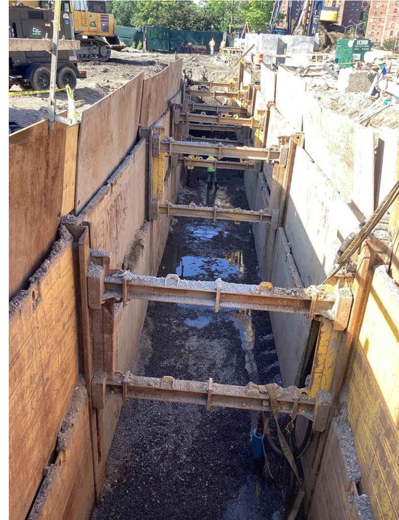
Deep sewer trench north of Track – June 2025
